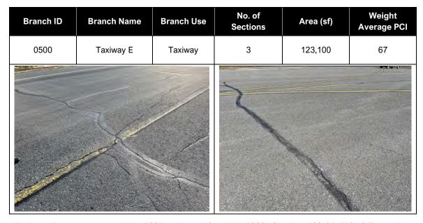
Taxiway E was constructed in 1965 and resurfaced in 1990. Section 500-01 (PCI 64) was last resurfaced in 2006, 500-02 (PCI 67) in 2005, and 500-03 (PCI 71) in 2010. Predominant distresses include low to medium severity longitudinal and transverse cracking, low to medium severity weathering and low severity raveling. Section 500-01 has some small areas with high severity longitudinal and transverse cracking and medium severity raveling.
