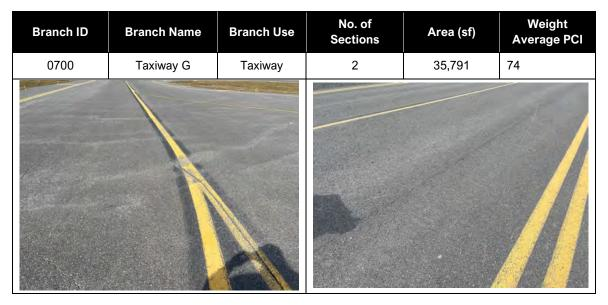
Taxiway G was constructed in 1968 and received resurfacing in 1990 and 2016. Common distresses include low severity longitudinal and transverse cracking and low severity weathering. Small quantities of medium severity longitudinal and transverse cracking and low severity raveling were observed.
