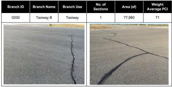
Taxiway B was constructed in 2006. Predominant distresses include low to medium severity longitudinal and transverse cracking, low and medium severity weathering and low severity raveling.
