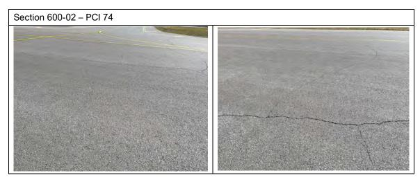
Section 600-02 of Taxiway F was constructed in 1965 and resurfaced in 1989, 1994 and 2016. Common distresses include low to medium severity longitudinal and transverse cracking and low severity weathering.
