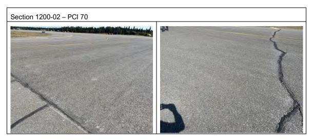
Section 1200-02 of Taxiway L was constructed in 1989 and was reconstructed in 2010. Common distresses are low to medium severity longitudinal and transverse cracking, low severity raveling and low to medium severity weathering.
