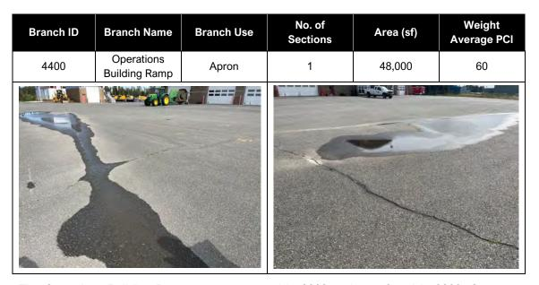
The Operations Building Ramp was constructed in 2002 and resurfaced in 2009. Common distresses include low to medium severity longitudinal and transverse cracking, low severity weathering and raveling, low severity depressions and alligator cracking.
