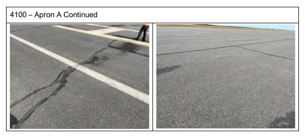
Apron A was constructed in 1965, resurfaced in 1985 and received surface reconstruction in 2010. Common distresses include low to medium severity longitudinal and transverse cracking and low to medium severity weathering.
