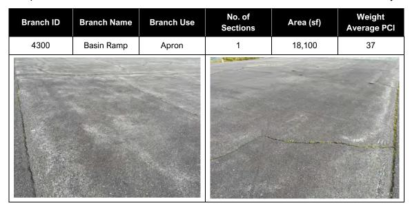
The Basin Ramp was constructed in 1989 and has received no work since. Common distresses include low, medium and high severity longitudinal and transverse cracking, low severity weathering and alligator cracking.
