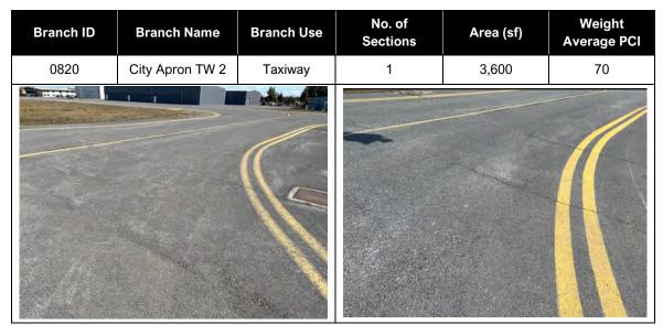
The City Apron Taxiway 2 was constructed in 1989 and resurfaced in 2016. Distresses observed include low to medium severity longitudinal and transverse cracking, low severity weathering and low severity raveling.
