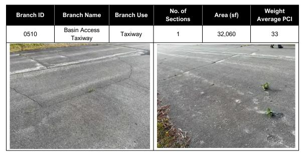
The Basin Access Taxiway was constructed in 1989 and has received no work since. Common distresses include low, medium and high severity longitudinal and transverse cracking, low severity weathering, and low, medium and high severity raveling. Other distresses include low and medium severity alligator cracking, with isolated high severity alligator cracking.
