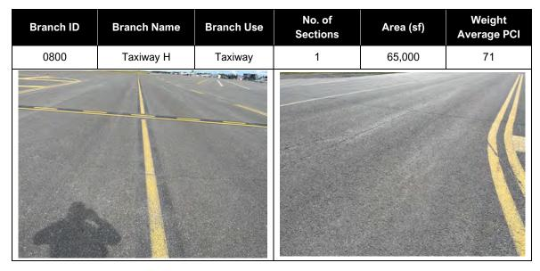
Taxiway H was constructed in 1989 and was resurfaced in 1994 and 2016. Common distresses include low to medium severity longitudinal and transverse cracking, low severity weathering and isolated areas of low severity raveling. A significant number of new longitudinal and transverse cracks were observed this inspection.
