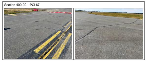
Section 400-02 of Taxiway D was constructed in 1971 the last known resurfacing was in 1990. Common distresses include low to medium severity longitudinal and transverse cracking, low severity weathering and small areas of low severity raveling.
