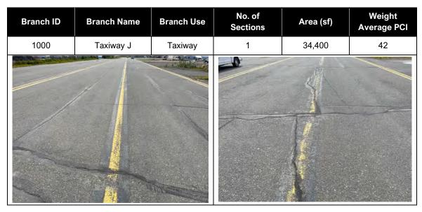
Taxiway J was constructed in 1968 and resurfaced in 1990. Common distresses include low, medium and high severity longitudinal and transverse cracking, low to medium severity raveling and low severity weathering. Other observed distresses are low severity depressions and alligator cracking.
