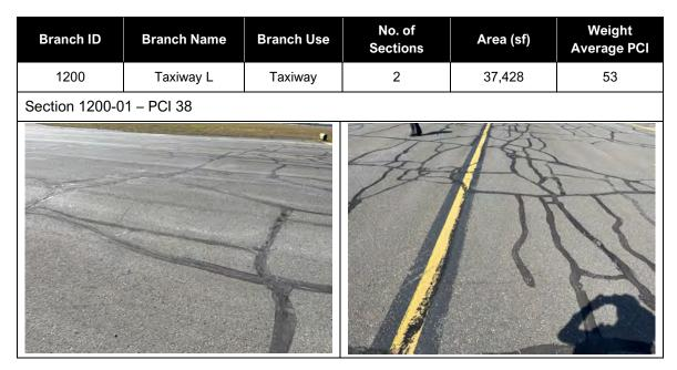
Section 1200-01 of Taxiway L was constructed in 1989 and has received no major work since. It contains low to medium severity block cracking, low severity weathering, and low to medium severity raveling. One small area of alligator cracking was observed.
