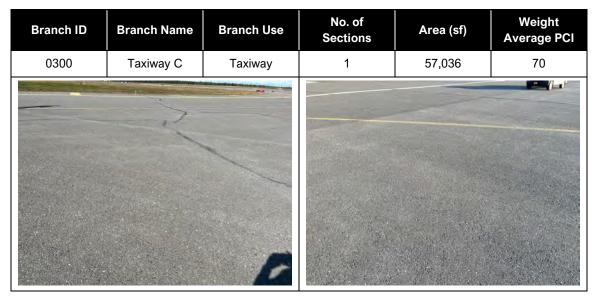
Taxiway C was reconstructed in 2006. Common distresses include low and medium severity longitudinal and transverse cracking, low severity weathering and low severity raveling.
