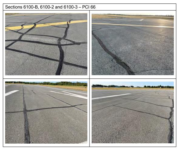
Sections 6100-B (PCI 62), 6100-2 (PCI 70) and 6100-3 (67) were constructed in 1990 and resurfaced in 2006. The top two photos are 6100-02 and 6100-03 (blast pads) and bottom two are 6100-B. Common distresses are low to medium severity longitudinal and transverse cracking and low severity weathering. Other distresses include low severity raveling and medium severity weathering.
