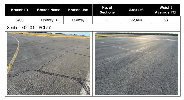
Section 400-01 of Taxiway D was constructed in 1971 was resurfaced in 1990 and 2006. Common distresses include low and medium severity longitudinal and transverse cracking, low severity weathering and low severity raveling. Other distresses observed include small areas of high severity cracking and medium severity weathering.
