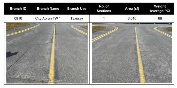
The City Apron Taxiway 1 was constructed in 1989 and resurfaced in 2016. Distresses observed include low to medium severity longitudinal and transverse cracking, low severity weathering and low severity raveling.
