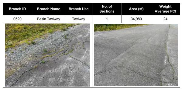
The Basin Taxiway was constructed in 1989 and has received no work since. Common distresses include low to medium severity block cracking, low to medium severity raveling, low to medium severity weathering, and low, medium and high severity alligator cracking. Other distresses observed include high severity depression and severe edge cracking.
