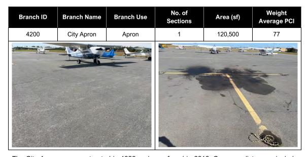
The City Apron was constructed in 1989 and resurfaced in 2016. Common distresses include low to medium severity longitudinal and transverse cracking, low severity weathering, and oil spillage.
