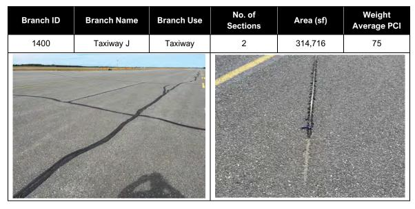
Taxiway J was constructed in 2010 and has received no work since. Common distresses include low severity longitudinal and transverse cracking, and low to medium severity weathering. There are small areas with raveling.
