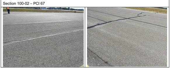
The last known resurfacing of the 100-02 portion of Taxiway A was in 1989. Predominant distresses include low to medium severity longitudinal and transverse cracking, low severity weathering, and low severity raveling. Distresses are in higher concentrations than in 100-01.
