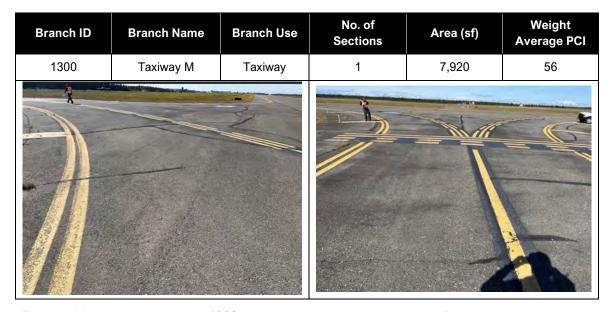
Taxiway M was constructed in 1998 and has received no work since. Distresses include low to medium severity longitudinal and transverse cracking, low severity raveling, low to medium severity weathering and a medium severity depression. There is a small area with medium severity raveling.
