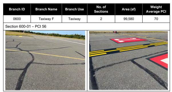
Section 600-01 of Taxiway F was constructed in 1965 and resurfaced in 1989 and 2006. Common distresses include low to medium severity longitudinal and transverse cracking, low to medium severity weathering and low severity raveling. Medium severity raveling was observed at isolated locations.
