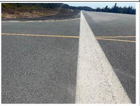
Taxiway A Section 0100-02 was initially constructed in 1991 and was completely reconstructed in 2018. Crack seal operations have not been performed on this section. The only distress observed was low severity weathering. No additional field observations were documented.
