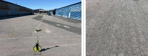
Taxilane B5 received a structural overlay in 1999. Crack sealing has not been performed on the branch. The most common distresses are low to medium severity fatigue cracking, low to high severity longitudinal and transverse cracking, low severity patching, and low to medium severity weathering. Field observations indicate highly degraded pavement with load-related distresses across the taxiway.
