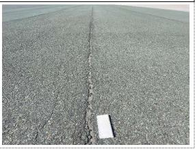
The pavement surface of Taxiway E1 Section 0510-04 was rehabilitated in 2006. Crack sealing has not been performed on this section. The most common distresses are low to medium severity longitudinal and transverse cracking, low to medium severity raveling, and low to medium severity weathering. Field observations indicate significant deterioration of the pavement surface characterized by widening of the paving lane joints and the progressive raveling of the coarse aggregate.
