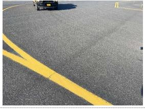
Taxiway D Section 0410-02 was realigned and completely reconstructed in 2020. Crack sealing has not been performed on the section. The most common distresses are low severity longitudinal and transverse cracking, and low severity weathering. Field observations include new unfilled cracks and initial surface deterioration.
