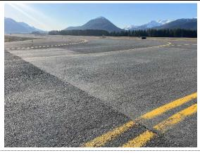
Surface rehabilitation was accomplished on Taxiway B2 Section 0220-03 in 2020. Crack sealing has not been performed on this section. The most common distresses are low severity longitudinal and transverse cracking, low severity raveling, and low severity weathering. Field observations include new unfilled cracks and initial surface deterioration, leading to localized areas of raveling across the taxiway.
