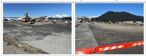
The portland cement concrete (PCC) sections of the Terminal Apron were under construction during the inspection. The 2021 PCIs for Sections 4100-HS1, 4100-HS2 and 4100-HS3 were 75, 71, and 64, respectively.
