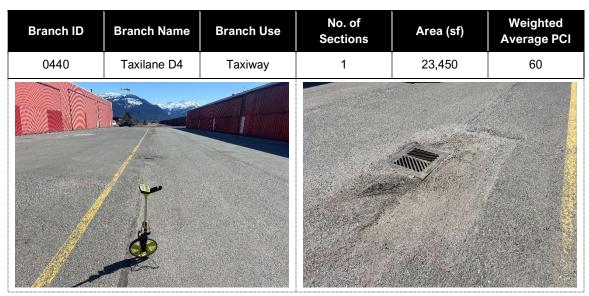
Taxilane D4 has not undergone any major work since its initial construction in 1998. Crack sealing has not been performed on the branch. The most common distresses are low to medium severity longitudinal and transverse cracking, low to high severity patching, low to high severity raveling, and low to medium severity weathering. Field observations indicate patches of variable quality, including some with indications of premature failure.
