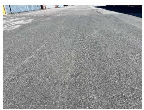
Taxilane B3 Section 0230-02 was reconstructed in 2020. Crack sealing has not been performed on this section. The most common distress is low severity weathering. Field observations include areas of mechanical damage from snowplow operations.
