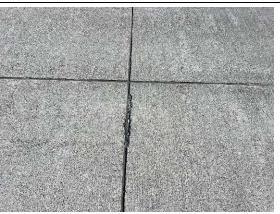
The Terminal Apron Section 4100-HS4 has not undergone any significant work since its initial construction in 2017. The most common distresses are medium severity joint seal damage, low severity joint spalling, and low severity corner spalling. Field observations suggest that initial damage to the joint sealant has progressed, resulting in joint and corner spalls.
