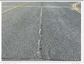
Major work has not been performed on Section 0220-02 since its initial construction in 2005. Crack sealing has not been performed on this section. The most common distresses are low severity longitudinal and transverse cracking, low to medium severity raveling, and low severity weathering. The pavement surface has deteriorated as characterized by widening of the paving lane joints and the progressive raveling of the coarse aggregate.
