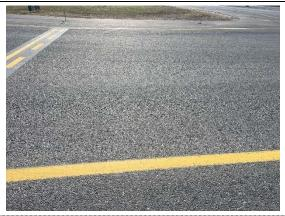
Taxiway E1 consists of five sections: 0510-01 through 0510-05. The pavement surface of Section 0510-01 was rehabilitated in 2020 along with Taxiway A. Crack sealing has not been performed on this section. The most common distresses are low severity raveling, and low severity weathering. Field observations include initial surface deterioration.
