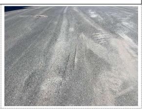
Taxilane B4 Section 0240-02 was reconstructed in 2020. Crack sealing has not been performed on this section. The most common distresses are low severity raveling and low severity weathering. Field observations include areas of mechanical snowplow damage.
