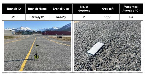
Taxiway B1 was realigned and fully reconstructed in 2016. Crack sealing has not been performed on the branch. The most common distresses are low severity longitudinal and transverse cracking, low severity patching, low to medium severity raveling, and low to medium severity weathering. Field observations indicate the initial deterioration of the AC surface layer has contributed to an increasing quantity and severity of raveling throughout the branch.
