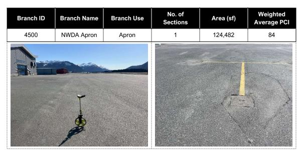
The Northwest Development Apron (NWDA) has not undergone any major work since its initial construction in 2016. Crack sealing has not been performed on the branch. The most common distresses are low severity patching, and low to medium severity weathering. Field observations highlight initial surface deterioration and localized patching around aircraft tie-down anchors.
