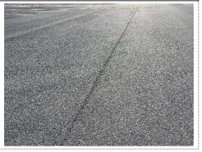
Taxiway C Section 0300-02 is an AC pavement that received surface rehabilitation in 2020. Crack sealing has not been performed on this section. The most common distresses are low severity raveling and low severity weathering. Field observations include initial surface deterioration which lead to localized areas of raveling and weathering across the taxiway.
