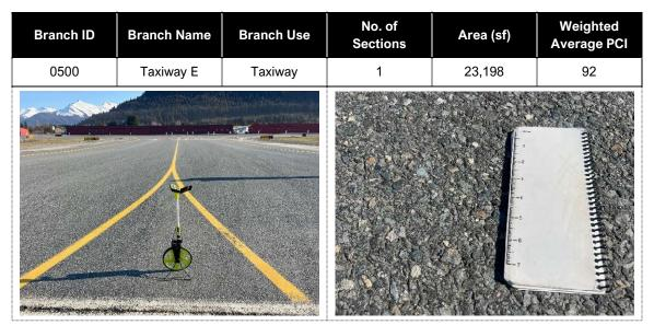
The Taxiway E pavement surface was rehabilitated, along with Taxiway A, in 2020. Crack sealing has not been performed on the branch. The most common distresses are low severity longitudinal and transverse cracking, and low severity weathering. Field observations include new unfilled cracks and initial surface deterioration.
