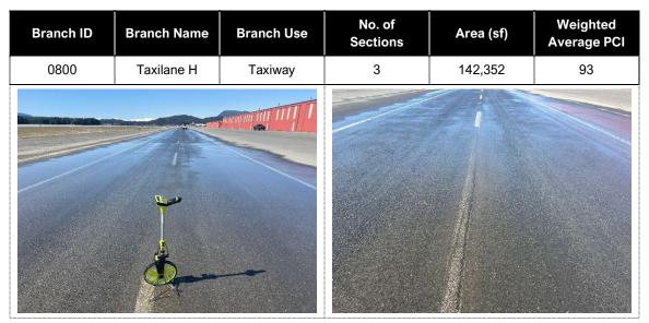
The Taxilane H pavement was completely rehabilitated in 2020. Crack sealing has not been performed on the branch. The most common distresses are low severity longitudinal and transverse cracking, and low severity weathering. Field observations include new unfilled cracks and initial surface deterioration.
