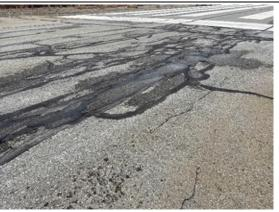
Runway 18/36 was constructed in 2003. Annual crack seal operations have been performed on the section. The most common distresses observed are low to medium severity longitudinal and transverse cracking, low to medium to high severity raveling, and low severity weathering. Field pavement observations include development of new unfilled cracks, widening of previously filled cracks, and areas of increased severity and quantity of raveling.
