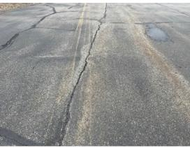
Taxiway C was also constructed in 2003 and received a sand tar surface treatment in 2015. Annual crack seal operations have been performed on the branch. The most common distresses observed are low to medium severity longitudinal and transverse cracking, low severity raveling, and low severity weathering. Field observations include wearing of the sand tar application due to climate and traffic, the initiation of new unfilled cracks, and widening of previously filled cracks.
