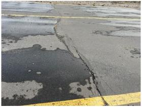
Similar to Taxiway A, Taxiway B was constructed in 2003 and received a sand tar surface treatment in 2015. Annual crack seal operations are behind schedule on this branch. The most common distresses observed are low to medium to high severity longitudinal and transverse cracking. Field observations include the development of new unfilled cracks, widening of previously filled cracks, and vegetation growth in the cracks.
