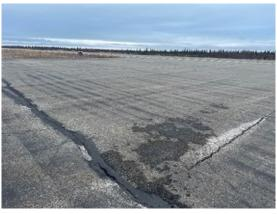
Taxiway A was constructed in 2003 and received a sand tar surface treatment in 2015. Annual crack seal operations have been performed on the branch. The most common distresses observed are low to medium severity longitudinal and transverse cracking, low severity raveling, and low severity weathering. Field observations include wearing of the sand tar application due to climate and traffic, creation of new unfilled cracks, and widening of previously filled cracks.
