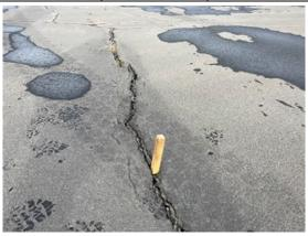
The West Apron was constructed in 2003 and received a sand tar surface treatment in 2015. Annual crack seal operations are behind schedule on this branch. The most common distresses observed are low to medium to high severity longitudinal and transverse cracking. Field observations include creation of new unfilled cracks, widening of previously filled cracks, and vegetation growth in the cracks.
