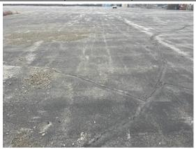
The Helipad was constructed in 2003 and received a sand tar surface treatment in 2015. Annual crack seal operations have been performed on the section. The most common distresses observed are low to medium severity longitudinal and transverse cracking, low severity raveling, and low severity weathering. Field observations include wearing of the sand tar application (not as much wear as the taxiways), initiation of new unfilled cracks, and widening of previously filled cracks.
