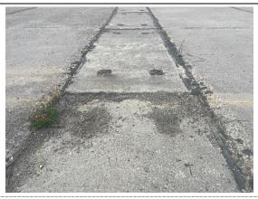
PCC Section 4100-03 was constructed in 1987 and has not received any major work since. The most common distresses are low severity linear cracking, medium severity joint seal damage, low to medium severity scaling, and low to medium severity faulting. This section of the North Apron is behind the Alert Hangar and is not often used due to its location. The large quantity of distresses at increasing severities is consistent with the nearly 40-year age of the pavement.
