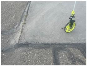
PCC section 4100-HS consists of four individual hardstands that were constructed in 1987 and have not received any major work since. The most common distresses are low severity joint seal damage, low to medium joint spalling, and low to medium corner spalling. The edges of the concrete hardstands are spalled, which is evident on each of the four hardstands.
