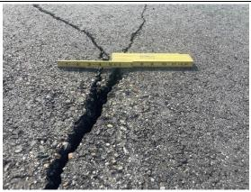
AC Section 4100-02 was constructed in 1987 and reconstructed in 2018. Crack seal operations have not been performed on the branch. The most common distresses are low to medium severity longitudinal and transverse cracking, oil spillage, low severity raveling, and low severity weathering. The quantity and severity of cracks is increasing across the parking apron. Crack sealing is recommended to slow the rate of deterioration.
