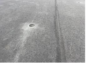
The East Ramp is made up of three sections, Section 4200-01 through 4200-03. Original construction of the East Ramp dates back to 1970. In 2023, the branch was reconstructed using the process of full depth reclamation. Crack seal operations have yet to be performed on the branch. Pavement inspectors observed no distresses other than a few core hole patches.
