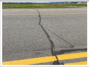
Originally constructed in 1975, Taxiway B Sections 0200-01, 0200-04, and 0200-06 were reconstructed in 2018. Routine crack seal operations have been performed on these sections. The most common distresses are low severity longitudinal and transverse cracking, low severity raveling, and low to medium severity weathering. Transverse cracks are developing across the width of the taxiway.
