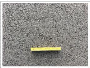
Taxiway W is composed of three sections, Sections 2300-01 through 2300-03. Sections 2300-01 and 2300-02 were constructed in 2002 and were reconstructed using a full-depth reclamation process in 2023. Crack seal operations have yet to be performed on these sections. No distresses were observed during the inspection.
