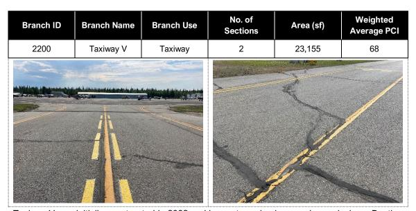
Taxiway V was initially constructed in 2002 and has not received any major work since. Routine crack seal operations have been performed on the branch. The most common distresses are low to medium severity longitudinal and transverse cracking, low severity patching, low severity raveling, and low to medium severity weathering. Pavement inspectors noted several transverse cracks and a utility patch that span the width of the taxiway.
