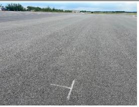
Taxiway S Section 1900-02 was newly constructed in 2022 together with the project on Section 1900-01. Crack seal operations have yet to be performed on the section. The most common distress was low severity weathering.
