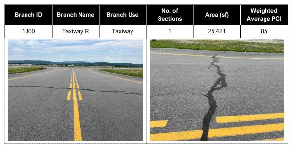
Taxiway R was originally constructed in 1985, reconstructed in 2002 and subsequently received an AC resurfacing in 2022 consisting of 4 inches of FDR and a 3-inch thick AC overlay. Routine crack seal operations have been performed on the branch. The most common distresses are low severity longitudinal and transverse cracking and low severity weathering. Transverse cracks are developing across the width of the taxiway.
