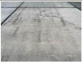
The PCC hardstands, Section 4400-HS, were constructed in 2007 and have not received any major work since. Routine crack and joint seal operations have been performed on the section. The most common distresses are low severity linear cracking, low severity scaling, and shrinkage cracking. Nearly every slab exhibits signs of shrinkage cracking, though this type of cracking typically does not extend through the full depth of the slab.
