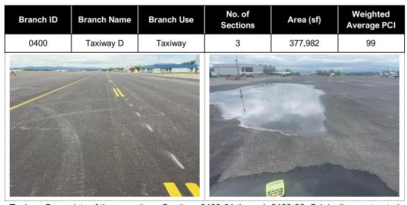
Taxiway D consists of three sections, Sections 0400-01 through 0400-03. Originally constructed during the period 1970 to 1998, TW D was reconstructed in 2023 through a process of full depth reclamation. Crack seal operations have yet to be performed on the branch. The most common distress is a number of low to medium severity depressions. A large depression was observed with standing water at the edge of TW D near the Wright Air Services lot.
