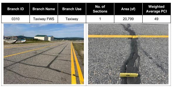
The Fish and Wildlife Services (FWS) Taxiway was initially constructed in 1985 and has not received any major work since. Routine crack seal operations have been performed on the branch. The most common distresses are low severity block cracking, low to medium severity longitudinal and transverse cracking, low severity raveling, and low to medium severity weathering. The pavement surface is developing new unfilled cracks and raveling of the coarse aggregate particles is progressing.
