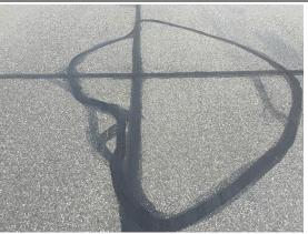
Section 0100-03 was originally constructed in 1961 and was most recently reconstruced in 2012. Routine crack seal operations have been performed on the section. The most common distresses are low severity longitudinal and transverse cracking, low severity raveling, and medium severity weathering. The pavement surface is developing new unfilled cracks outside the planned relief cuts. Pavement inspectors note the development of fatigue cracking in high-traffic areas across the section.
