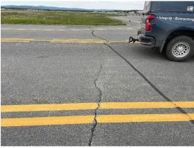
Taxiway S consists of two sections, Section 1900-01 and Section 1900-02. Section 1900-01 was originally constructed in 2002 and was resurfaced in 2022 (4 inches FDR followed by a 3-inch thick AC overlay). Routine crack seal operations have been performed on the section. The most common distresses are low severity longitudinal and transverse cracking and low severity weathering. Transverse cracks are developing across the width of the taxiway.
