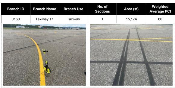
Taxiway T1 was constructed in 1991 and in 2005 was subsequently realigned and reconstructed. Routine crack seal operations have been performed on the branch. The most common distresses are low severity longitudinal and transverse cracking, low to medium severity raveling, and medium severity weathering. The AC surface continues to deteriorate as evidenced by the higher quantity and severity of raveling and weathering across the branch.
