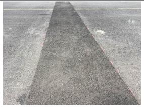
Taxiway T is composed of two sections, Section 2000-01 and Section 2000-02. Section 2000-01 was originally constructed in 2002 and in 2022 received AC resurfacing (4 inches of FDR following by a 3-inch thick AC overlay). Routine crack seal operations have been performed on the section. The most common distresses are low severity patching and low severity weathering. A utility patch spans the width of the taxiway.
