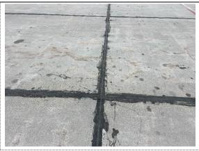
West Ramp PCC Sections 4100-C4 and 4100-C5 were constructed in 2007 and have not received any major work since. Routine crack and joint seal operations have been performed on these sections. The most common distresses observed are low severity scaling and low severity joint spalling. Pavement inspectors observed low severity scaling, which manifests as delamination of the slab surface.
