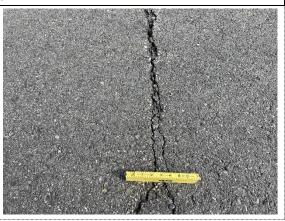
Taxiway B Section 0200-05 was constructed in 1975 and was reconstructed in 2022. Section 0200-08 was constructed as part of the 2008 project. Crack seal operations have yet to be performed on these sections. The most common distresses are low severity longitudinal and transverse cracking, low severity raveling, and low to medium severity weathering. Transverse cracks are developing across the width of the taxiway.
