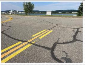
Taxiway W Section 2300-03 was constructed in 2002 and has not received any major work since. Crack seal operations have yet to be performed on the section. The most common distresses are low to medium severity longitudinal and transverse cracking, low severity patching, low severity raveling, and low severity weathering. Pavement inspectors noted several transverse cracks and a utility patch that span the width of the taxiway.
