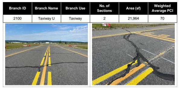
Taxiway U was initially constructed in 2005 and has not received any major work since. Routine crack seal operations have been performed on the branch. The most common distresses are low to medium severity longitudinal and transverse cracking, low severity patching, low severity raveling, and low to medium severity weathering. Pavement inspectors noted several transverse cracks and a utility patch that span the width of the taxiway.
