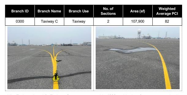
Like Taxiway A and B, Taxiway C was constructed in 1998 and had surface reconstruction in 2012. Annual crack seal operations have been performed on the branch. The most common distresses observed are low severity depression, low severity longitudinal and transverse cracking, low severity raveling, and low severity weathering. Field observations include areas of standing water along the length of the taxiway.
