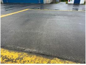
Taxiway B Section 0200-02 was constructed in 1995 and has not received any major work since. The only distress observed was low severity linear cracking. No additional field observations were made during the inspection.
