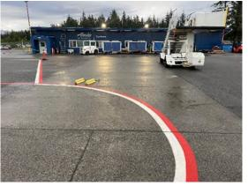
The Paved Apron Section 4100-04 was initially constructed in 2010 and has not received any major work since. The most common distresses observed are low severity joint seal damage and low severity scaling. Field observations include wearing of the surface of the concrete leading to the low severity scaling, and initial deterioration of the joint sealant causing low severity joint seal damage.
