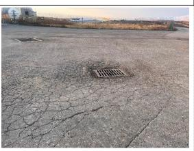
The smaller section (27,340 Sq Ft) of the North Ramp was constructed in 1970 and has not received any major work since. Crack seal operations have not been performed on the branch. The most common distresses observed are low to high severity alligator cracking, low to medium severity longitudinal and transverse cracking, low to high severity raveling, and low severity weathering.
