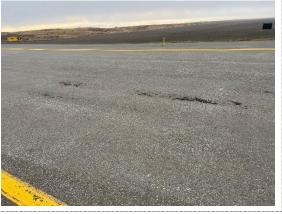
Taxiway A was initially constructed in 1942 and the most recent major work was a surface course in 2005. Crack seal operations have not been performed on the branch. The most common distresses observed are low severity longitudinal and transverse cracking, low to medium severity raveling, and low to medium severity weathering. Field observations include wearing of the pavement surface due to climate and traffic and the creation of new unfilled cracks.
