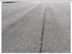
The larger section (301,000 Sq Ft) of the North Ramp, connected to Taxiway C, was first built in 1972 and underwent surface reconstruction in 2012. Crack seal operations have not been performed on the branch. The most common distresses observed are low severity longitudinal and transverse cracking, low severity raveling, and low severity weathering. Field observations include expedited wearing of the paving joints causing an increased quantity and severity of distresses.
