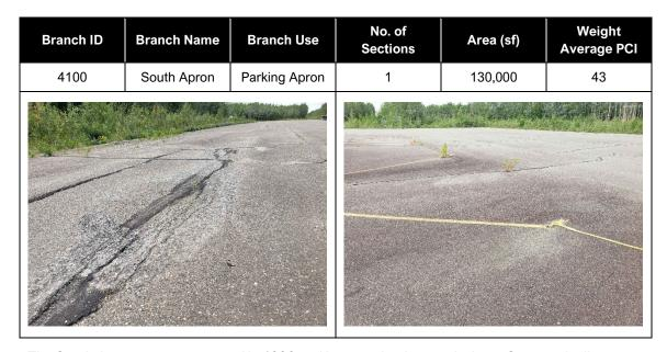
The South Apron was constructed in 1996 and has received no work since. Commonly distresses are low to medium severity longitudinal and transverse cracking, low severity weathering and low severity raveling. Areas near the edge of the apron have more severe distresses that include low to medium severity alligator cracking, medium severity raveling, medium severity swelling and a high severity depression.
