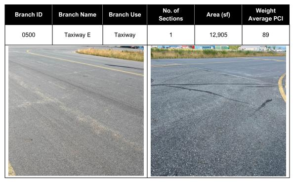
Taxiway E was constructed in 1978 and was resurfaced in 2018. The distresses on the taxiway are low to moderate severity longitudinal and transverse cracking and low severity weathering.
