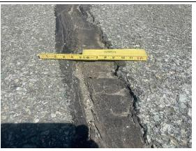
Section 1000-02 was constructed in 2007 and has not received any major work since. Occasional crack seal operations have been performed on the section. The most common distresses observed are low to medium severity longitudinal and transverse cracking, low severity raveling, and low severity weathering. Field observations include sealed cracks where the sealant is failing in areas.
