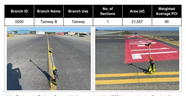
Like Taxiway A, Taxiway B was initially constructed in 1985 then received a 2-inch mill and overlay in 2012 and another mill and overlay in 2022. The most common distresses observed are low severity longitudinal and transverse cracking. Field observations include localized spots of raveling, plus cracks developing on the new pavement that should be crack sealed.
