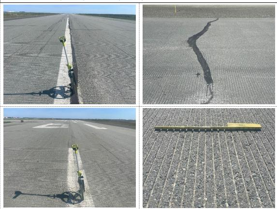
Runway 01R/19L Sections 6300-01 and 6300-03 were initially constructed in 2009 and received a 2-inch overlay in 2021. Occasional crack seal operations have been performed on the branch. The most common distresses observed are low severity longitudinal and transverse cracking. Field observations include localized spots of weathering and sealed cracks that should continue to be crack sealed.
