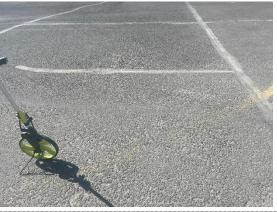
Taxiway M Section 1300-01 was constructed in 1999 and has not received any major work since. Occasional crack seal operations have been performed on the section. The most common distresses observed are low severity longitudinal and transverse cracking and low severity raveling. Field observations include localized spots of medium to high severity raveling, plus cracks that are adequately sealed.
