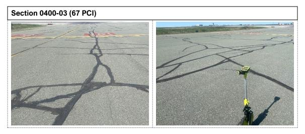
Taxiway D Section 0400-03 was initially constructed in 2009 and has not received any major work since. Occasional crack seal operations have been performed on the section. The most common distresses observed are low severity longitudinal and transverse cracking, low severity raveling, and low severity weathering. Field observations include a large amount of cracking, all of which are sealed, plus localized spots of medium to high severity raveling.
