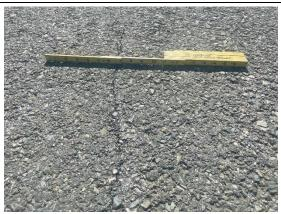
Taxiway O Section 1500-01 was constructed in 2009 and has not received any major work since. Occasional crack seal operations have been performed on the section. The most common distresses observed are low severity longitudinal and transverse cracking and low to medium severity weathering. Field observations include sealed cracks and further wearing of the pavement surface leading to the medium severity weathering.
