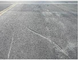
Taxiway D Section 0400-01 was initially constructed in 1989 then received a 2-inch mill and overlay in 2012 and another mill and overlay in 2022. Section 0400-02 was initially constructed in 2009 then received a mill and overlay in 2022. The most common distresses observed are low severity longitudinal and transverse cracking. Field observations include localized spots of raveling, plus cracks developing on the new pavement that should be crack sealed.
