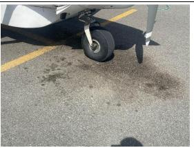
The south GA apron Section 4400-01 was initially constructed in 1988 and received a 2-inch mill and overlay in 2018. Crack seal operations have not been performed on the section. The most common distresses observed are low severity longitudinal and transverse cracking, oil spillage, and low severity weathering. Field observations include numerous locations of oil spillage from the GA aircrafts, and the development of low severity cracking that should be crack sealed.
