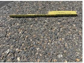
Taxiway E Section 0500-02 was constructed in 1985 and has not received any major work since. Occasional crack seal operations have been performed on the section. The most common distresses observed are low to medium severity longitudinal and transverse cracking, low severity raveling, and medium severity weathering. Field observations include wearing of the surface leading to the medium severity weathering, and sealed cracks that should be touched up with additional sealant.
