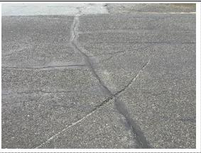
Taxiway G Section 0700-03 was initially constructed in 1985 and received a surface reconstruction in 2001. Occasional crack seal operations have been performed on the section. The most common distresses observed are low to medium severity longitudinal and transverse cracking, low severity raveling, and medium severity weathering. Field observations include wearing of the surface leading to the medium severity weathering, and sealed cracks where the sealant is failing in areas.
