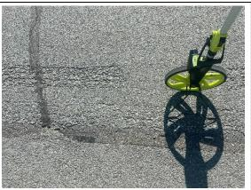
Section 4300-05 was initially constructed in 1985 and received a 2-inch overlay in 2012. Occasional crack seal operations have been performed on the section. The most common distresses observed are low to medium severity longitudinal and transverse cracking and low severity weathering. Field observations include localized spots of low to high severity raveling.
