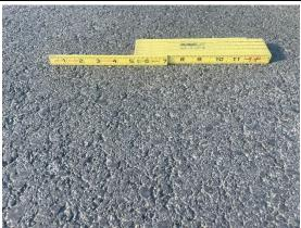
Taxiway G Sections 0700-01 and 0700-05 were initially constructed in 1996 and 2009, respectively, then both received a mill and overlay in 2022. Crack seal operations have not been performed on these sections. The most common distresses observed are low severity longitudinal and transverse cracking. Field observations include localized spots of raveling, plus cracks developing on the new pavement that should be crack sealed.
