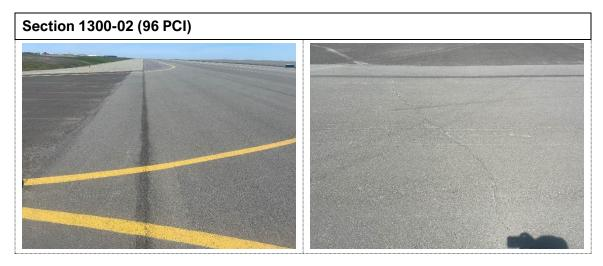
Section 1300-02 was initially constructed in 1999 and received a mill and overlay in 2022. Crack seal operations have not been performed on the section. The most common distresses observed are low severity longitudinal and transverse cracking. Field observations include cracks developing on the new pavement that should be crack sealed.
