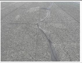
The west apron Section 4200-01 was initially constructed in 1985 and received a surface reconstruction in 2001. Occasional crack seal operations have been performed on the branch. The most common distresses observed are low to medium severity longitudinal and transverse cracking, low severity raveling, and medium severity weathering. Field observations include wearing of the surface leading to the medium severity weathering, and sealed cracks where the sealant is failing in areas.
