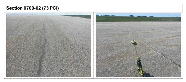
Section 0700-02 was initially constructed in 1985 then received a surface reconstruction in 2001 and a 2-inch overlay in 2017. Occasional crack seal operations have been performed on the section. The most common distresses observed are low to medium severity longitudinal and transverse cracking and low severity weathering. Field observations include sealed cracks, some of which have progressed into medium severity, that should be touched up with additional sealant.
