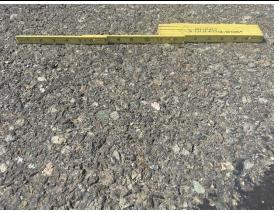
Section 4100-02 was initially constructed in 1973 then received a surface reconstruction in 2001. Occasional crack seal operations have been performed on the section. The most common distresses observed are low severity longitudinal and transverse cracking, low severity raveling, and medium severity weathering. Field observations include wearing of the surface leading to the medium severity weathering, and sealed cracks that should be touched up with additional sealant.
