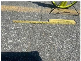
Taxiway J Section 1000-01 was initially constructed in 1988 and received a mill and overlay in 2018. Crack seal operations have not been performed on the section. The most common distresses observed are low to medium severity longitudinal and transverse cracking and low severity weathering. Field observations include localized spots of low to high severity raveling, plus the development of cracks that should be crack sealed.
