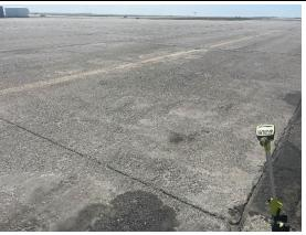
The PCC section 4100-04 was constructed in 2017 and has not received any major work since. The most common distresses observed are high severity joint seal damage, medium severity scaling, and medium severity joint and corner spalling. Field observations include wearing of the surface of the concrete leading to the medium severity scaling.
