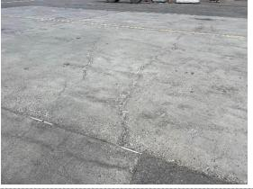
PCC Section 4100-03 was constructed in 2014 and has not received any major work since. The most common distresses observed are low to medium linear cracking, high severity joint seal damage, and low to high severity joint spalling. Field observations note the high severity joint seal damage compromises the pavement's ability to prevent water infiltration. This infiltration can exacerbate existing distresses and lead to further deterioration of the pavement structure.
