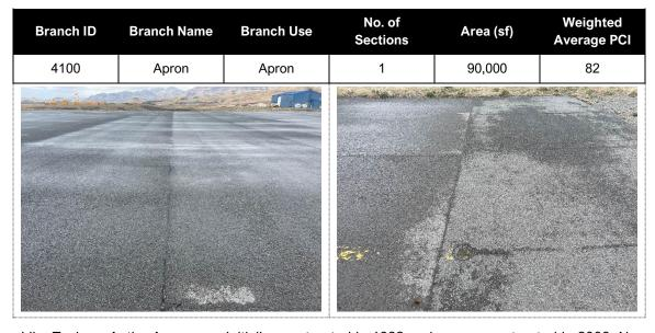
Like Taxiway A, the Apron was initially constructed in 1982 and was reconstructed in 2009. No crack seal operations have been performed on the branch. The most common distresses observed are low severity longitudinal and transverse cracking, low to medium severity raveling, and low severity weathering. Field observations include development of new unfilled cracks and the deterioration of the paving joints creating additional cracks and raveling throughout the apron.
