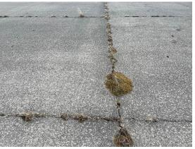
The PCC section was also constructed in 1990 and has not received any major work since. The most common distresses observed are high severity joint seal damage and low severity scaling. Field observations include wearing of the surface of the concrete leading to the low severity scaling, and vegetation growth in every joint leading to the high severity joint seal damage.
