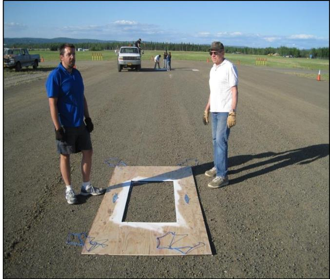
A template was cut from a sheet of plywood, with rope loops attached to the corners to make them easy to pick up and move. The template was hinged for easy transport and storage. In some cases, loose rocks were brushed away from the painting surface.
