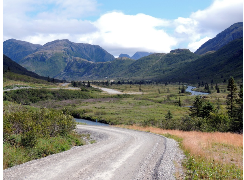
Figure 32: Williamsport Pile Bay Road
