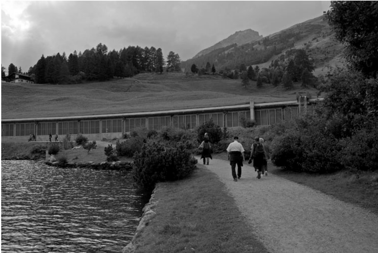
Figure 15: Shed-roof Gallery Snowshed, Davos, Switzerland
