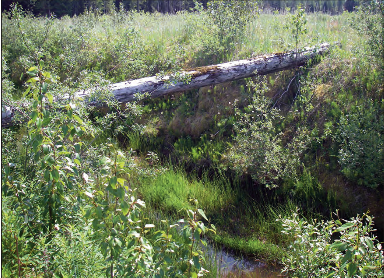
Figure 21. Collector ditch south of runway 11/29. CRC LLC 2009.
