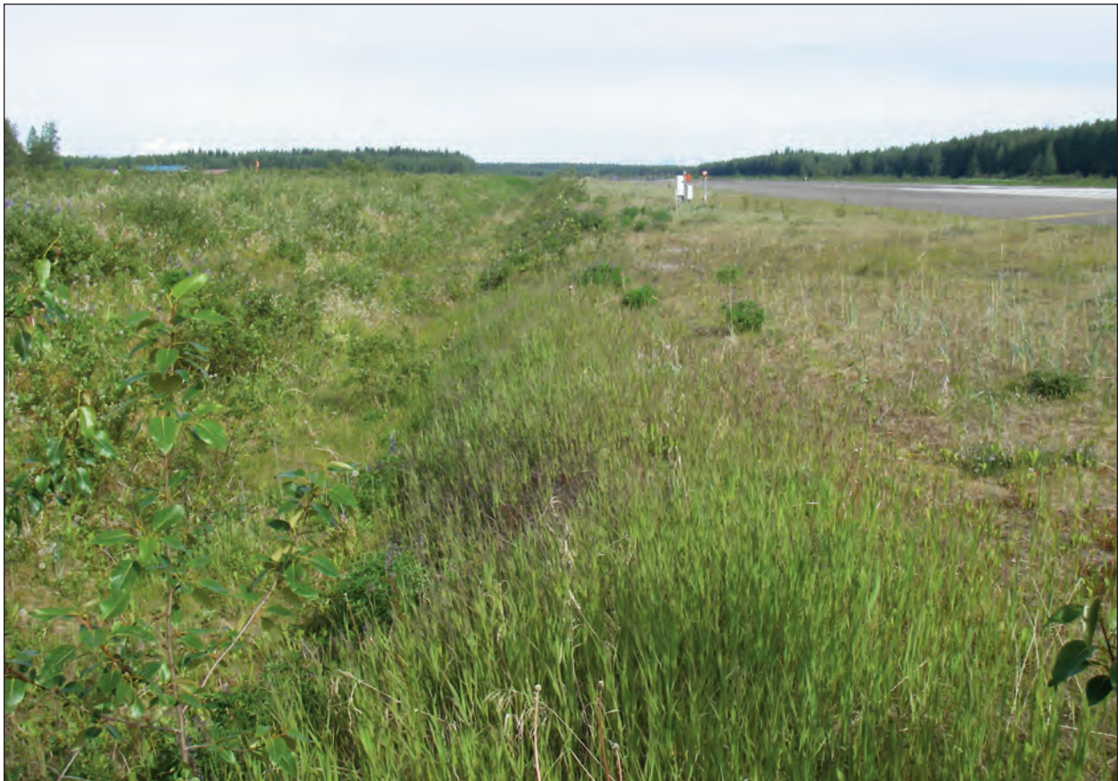
Figure 20. Feeder ditch paralleling the western edge of runway 11/29. View northwest. CRC LLC 2009.
