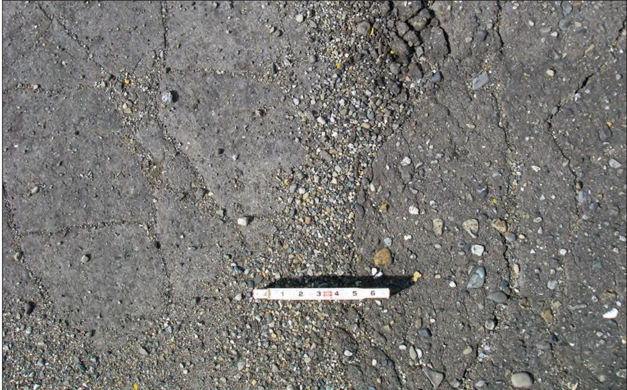
Figure 16. Layered pavement, with World War II-era pavement to the left. CRC LLC 2009.
