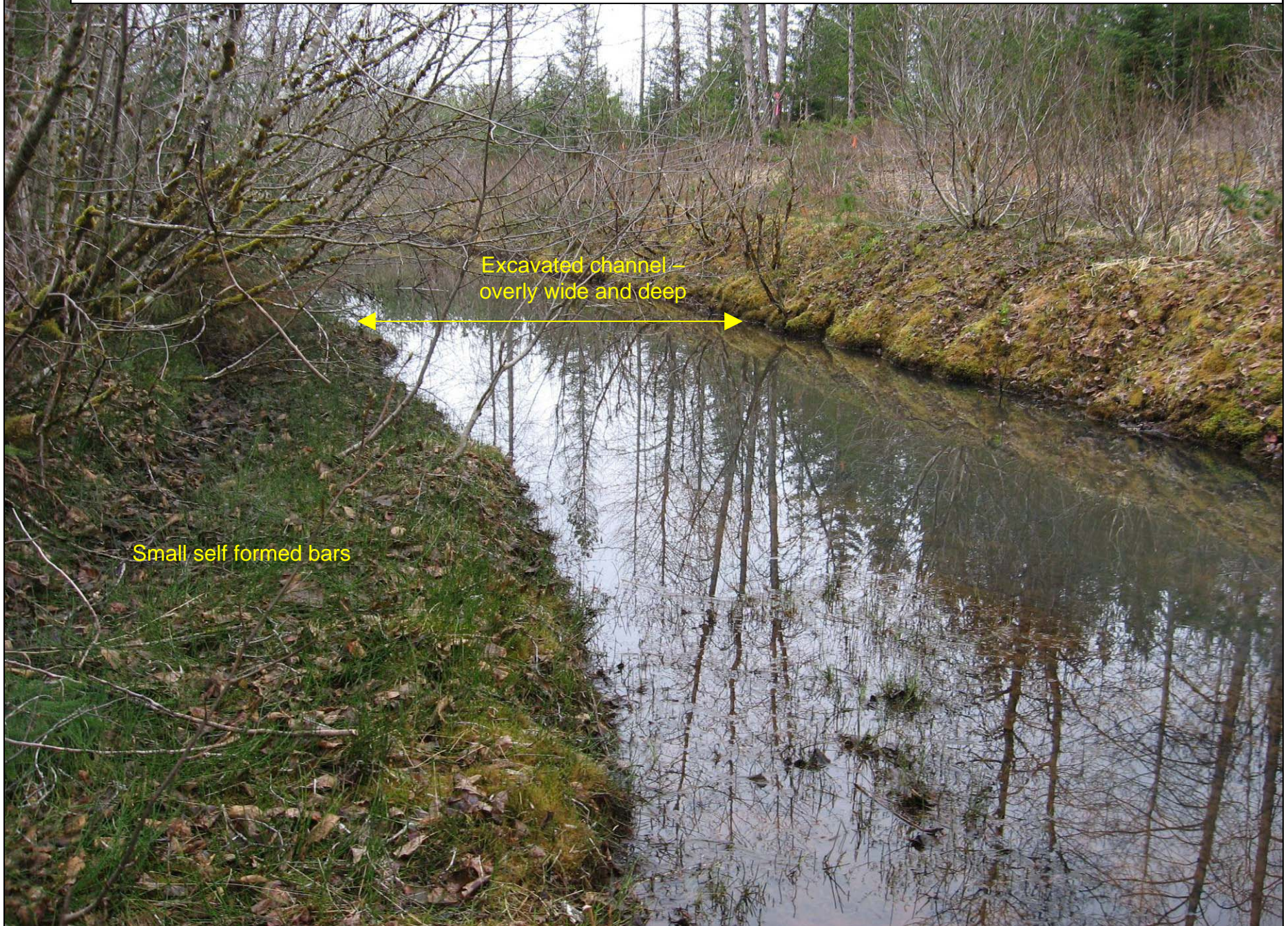
Figure 3 - Typical conditions for reach to be abandoned and filled
