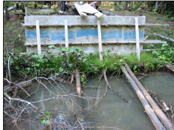
Abutment just above OHW
