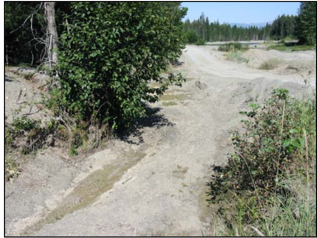
Drainage constructed to reduce flooding
