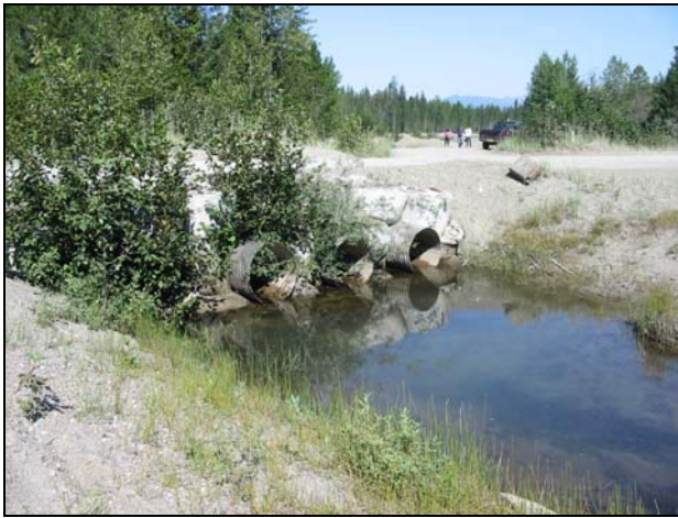
Culverts below DNR Gravel Pits
