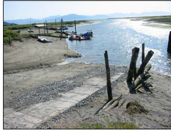
Repaired Launch Ramp
