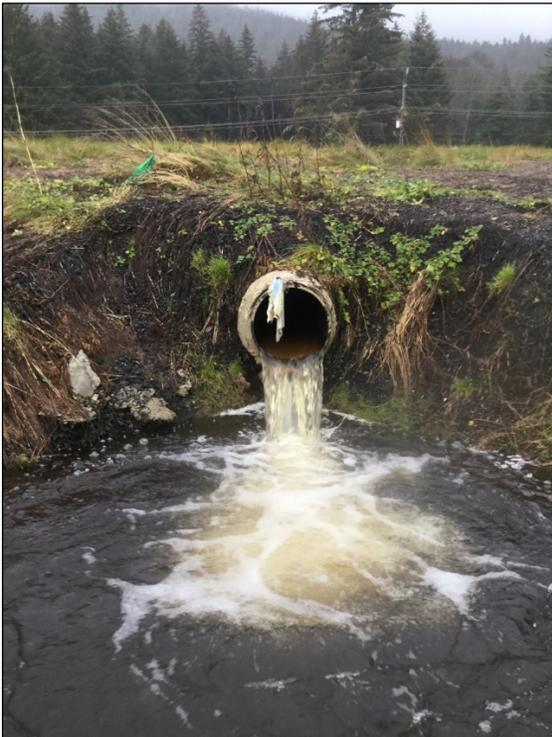
Figure 3.—Perched culvert on the stream at WP 4104.
