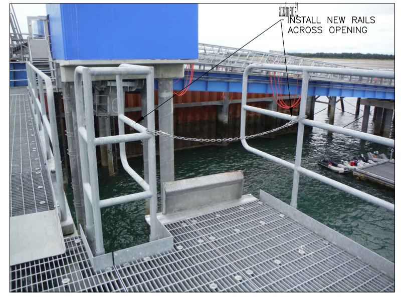
VIEW OF RAIL OPENING
