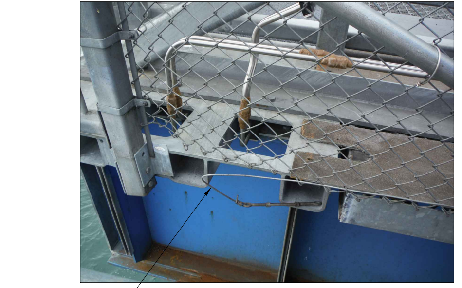
ADD END CLAMP AND REPAIR TENSION WIRE
