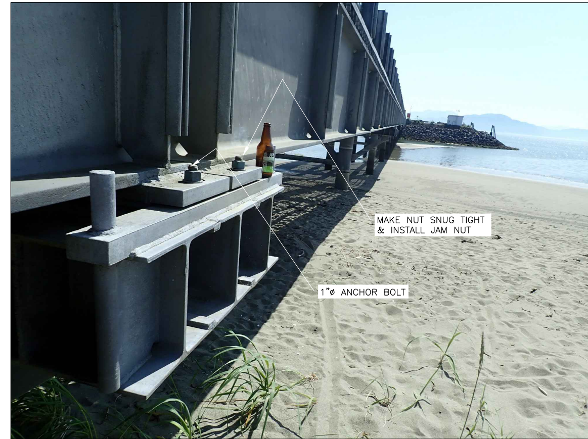
3 ANCHOR BOLT RETROFIT 001|003
