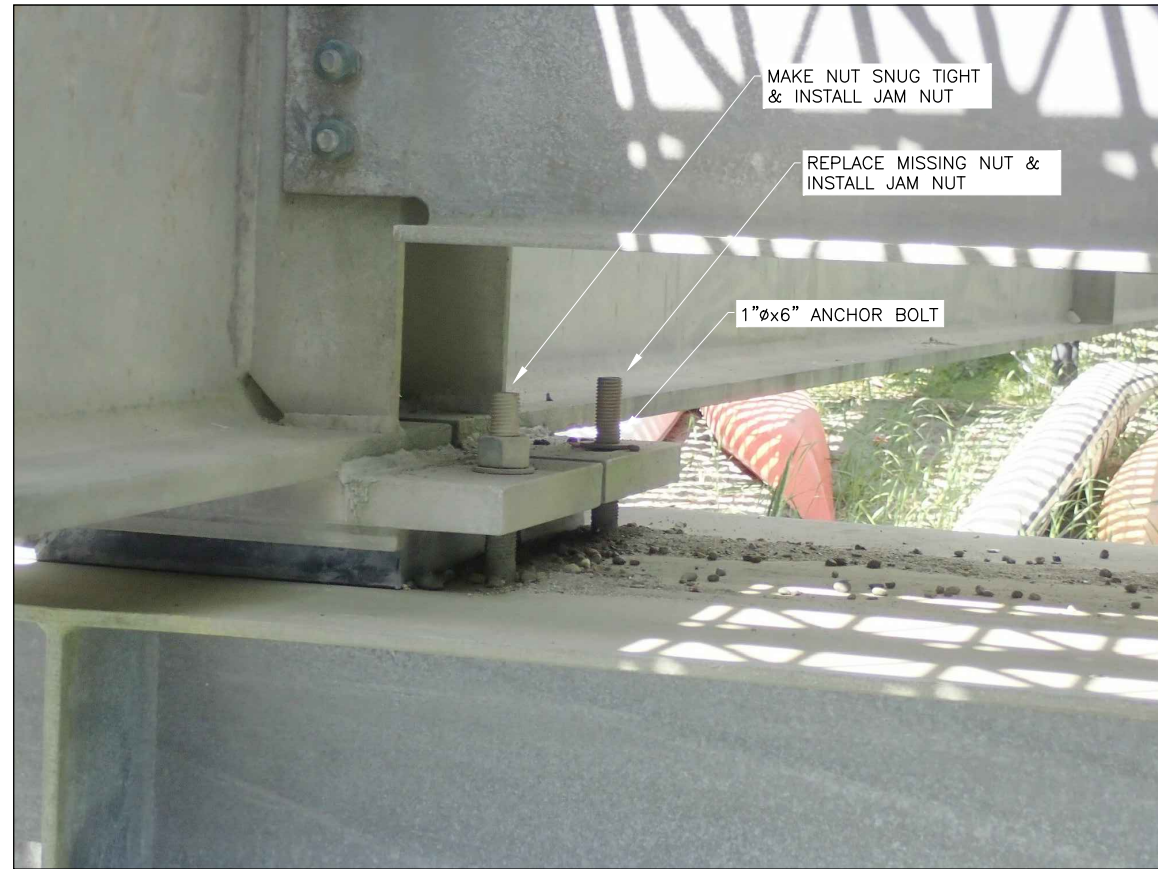
2 ANCHOR BOLT RETROFIT 001|003
