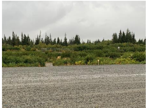
Figure 13: Fencing Beside Runway, Looking South
