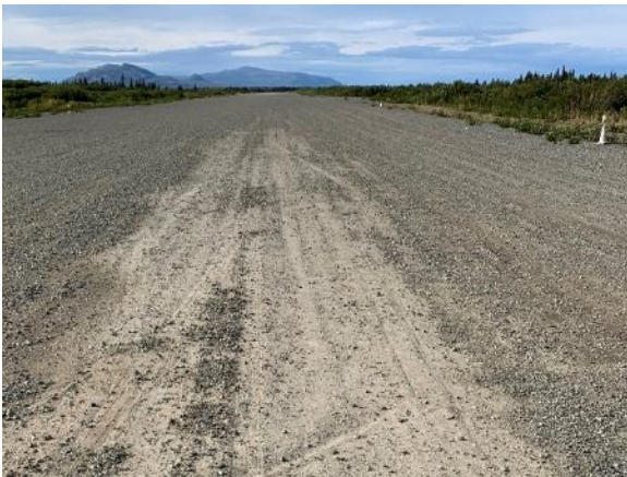
Figure 4: Thin Surfacing on Runway, Looking West
