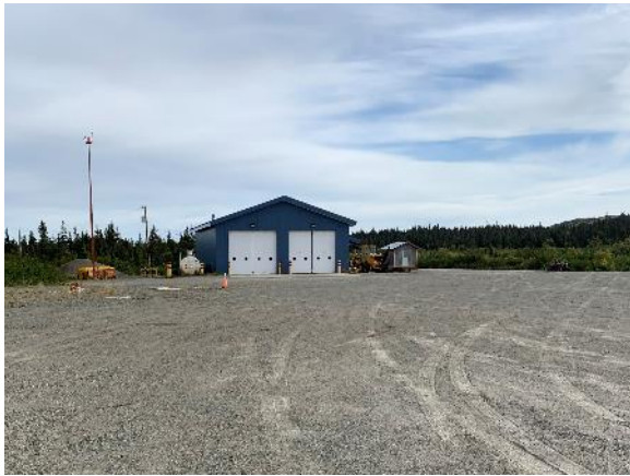
Figure 10: SREB and Eastern Portion of Apron, Looking East
