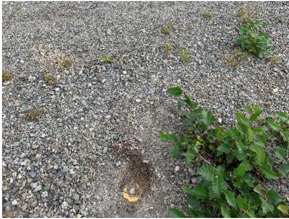
Figure 8 Base of Missing Edge Light
