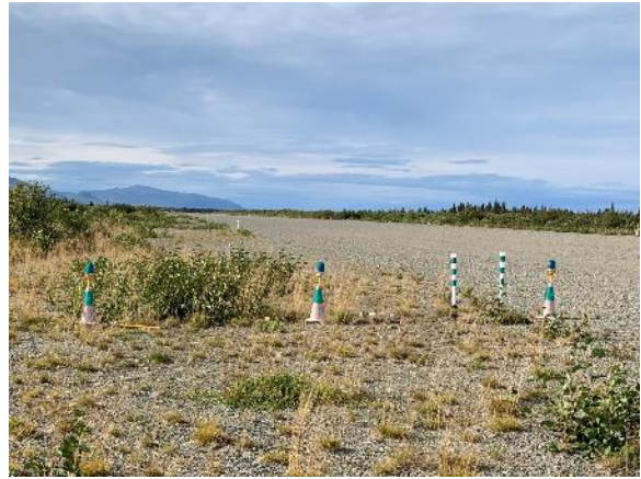
Figure 9: Missing Threshold markers, Looking West
