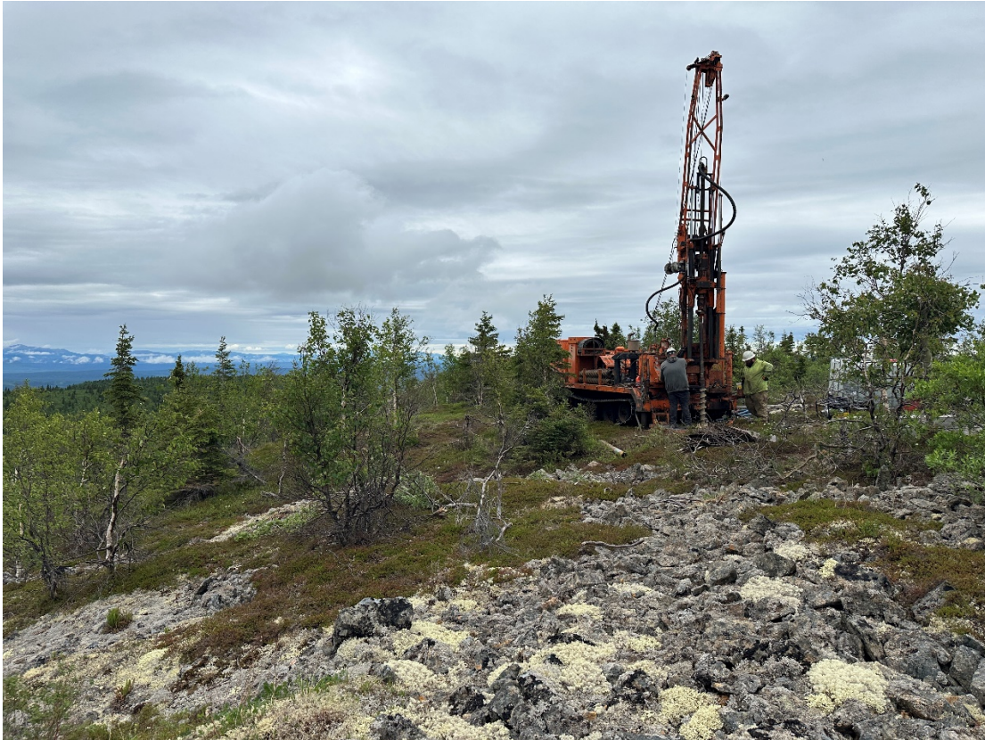
Drilling at TH35-03
