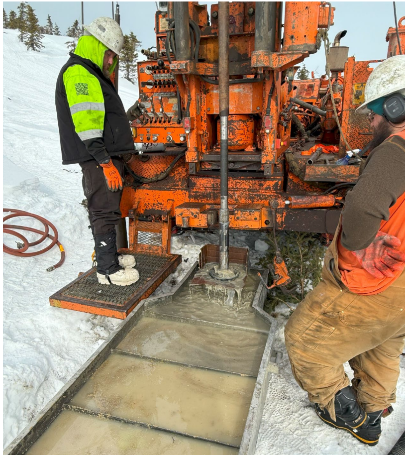
NQ Coring at TH25-01
