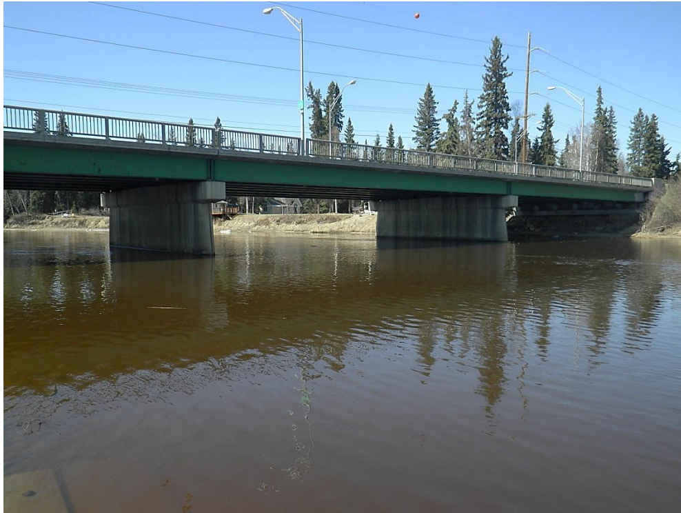
Photo 1 Chena River Bridge at University Avenue looking northwest; May 20, 2013
