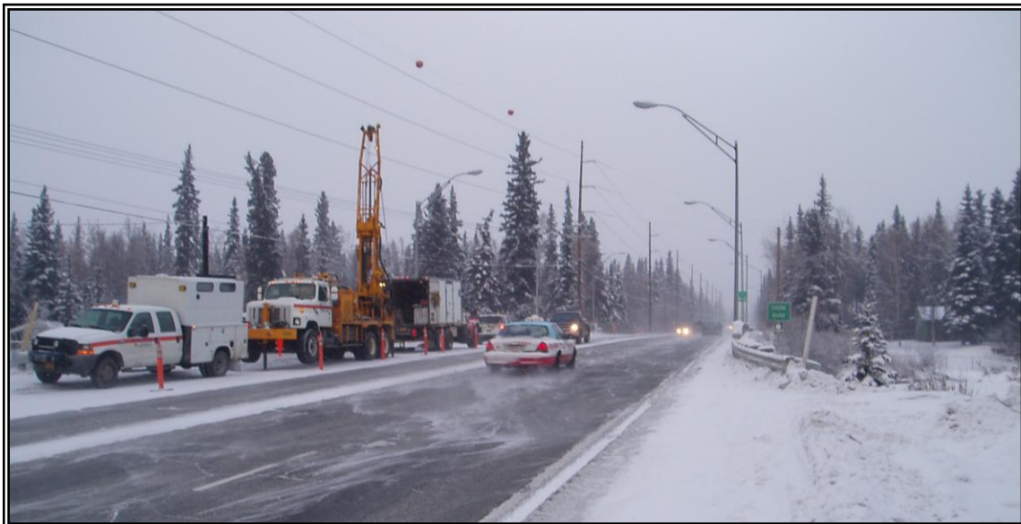
Figure 2. University Ave. Chena River Bridge, looking north.
