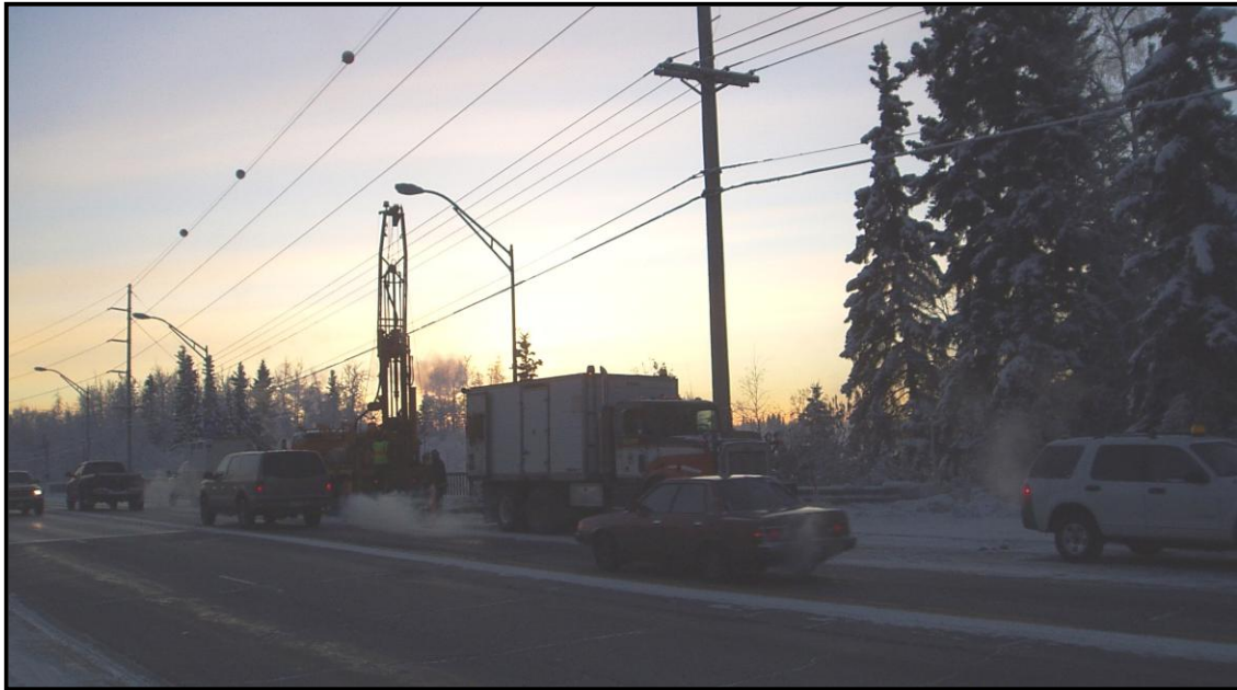
Photo 1. University Ave. southbound. Overhead powerlines along west side.
