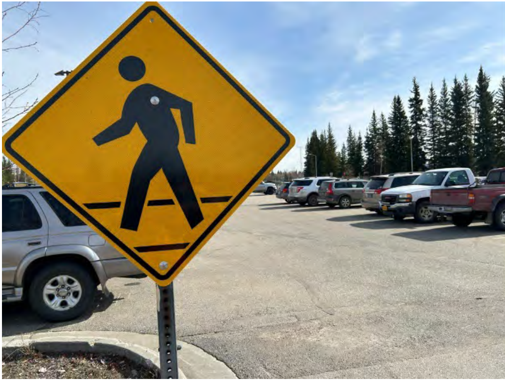
Figure 45. Pedestrian warning signs in parking lot mounted lower than SUV vehicles
