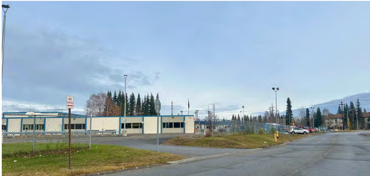
Figure 53. 24-10-13 SUN 1:41 PM U-Park Building access to midblock Sandvik St (2 driveways)
