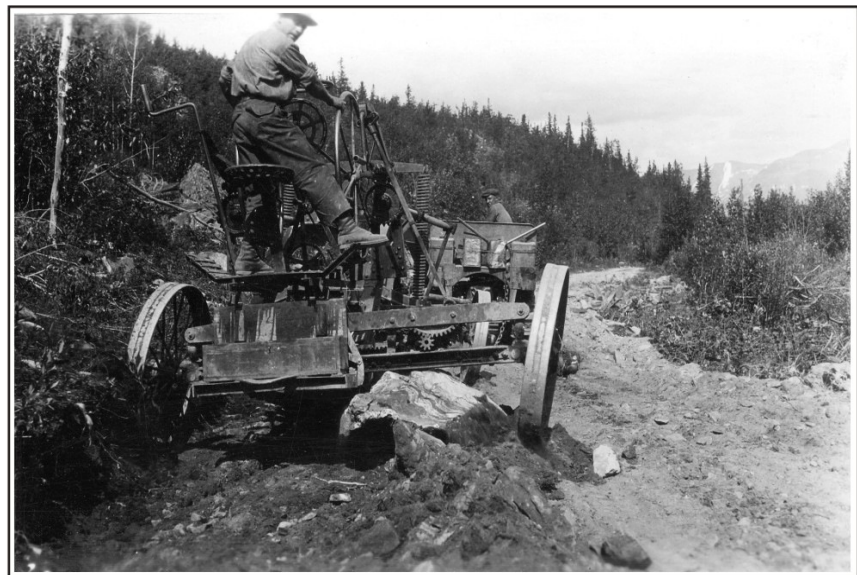
Figure 9. An ARC employee using a mechanical grader to widen a road. Photo courtesy of ADOT&PF Bridge Section, Juneau.
