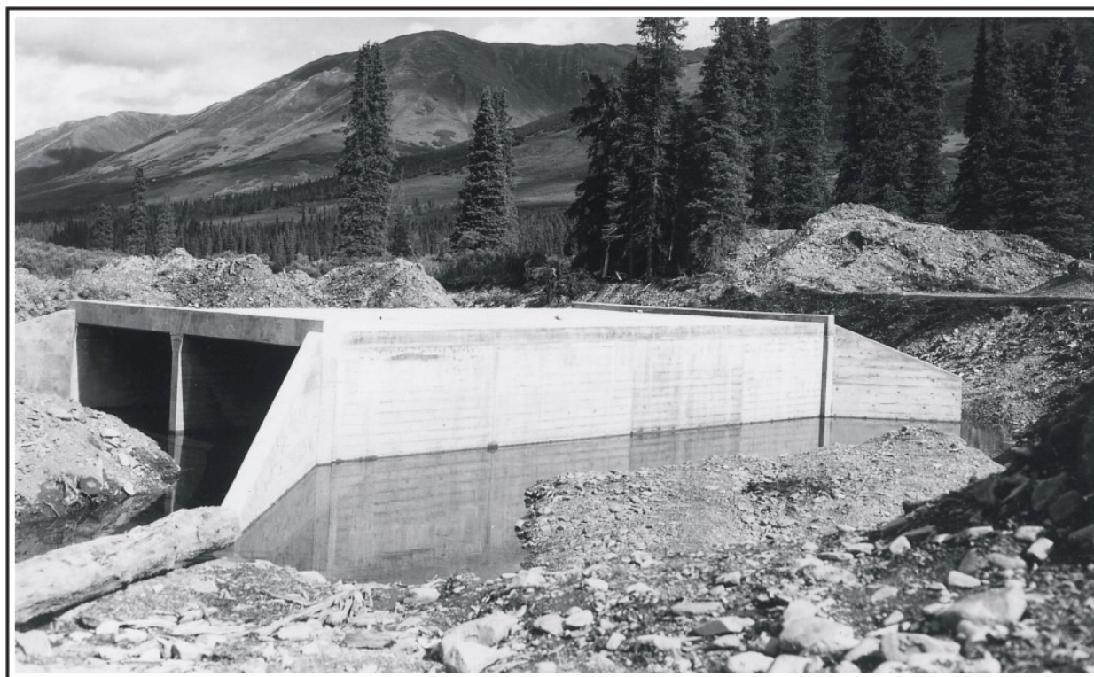
Figure 167. Rigid frame concrete bridge near completion at Summit Creek, Seward Highway, September 1951. U.S. Alaska Road Commission Collection, PCA 61-94-22, Alaska State Library.
