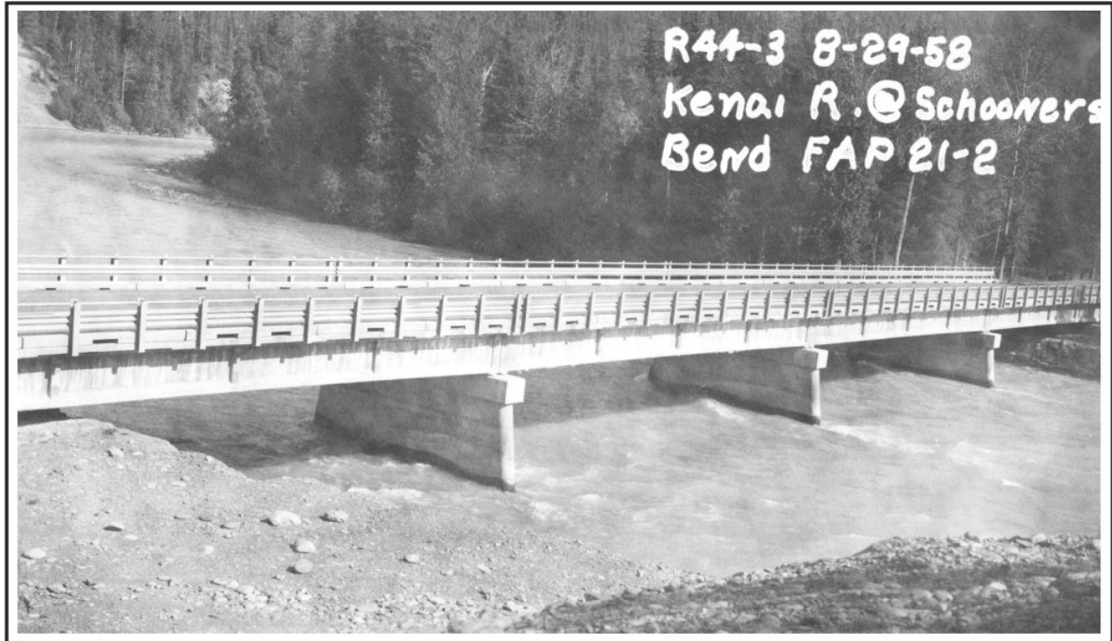
Figure 165. The light-weight concrete girder bridge at Schooners Bend on the Kenai River, August 29, 1958. BPR photograph, ADOT&PF Bridge Section, Juneau.
