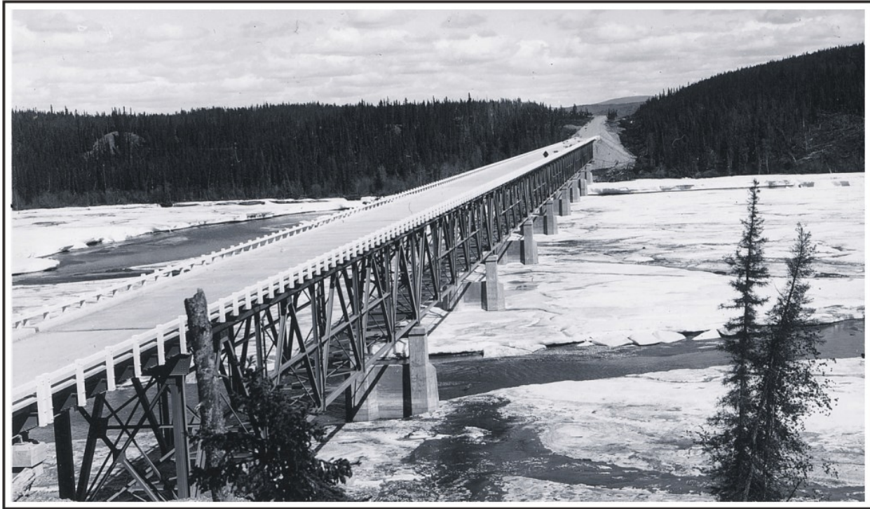
Figure 141. The 9-span steel deck truss bridge at Robertson River on the Alaska Highway, June 1946. U.S. Alaska Road Commission Collection, PCA 61-15-125, Alaska State Library.
