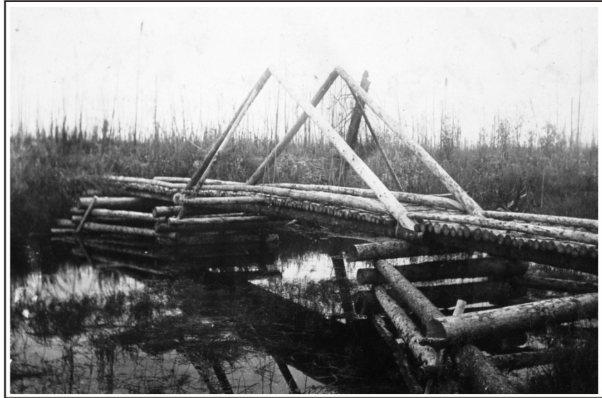
Figure 35. A king post log bridge with log cribbed piers at Mile 89 on the WAMCATS Line, 1913. Rita Cottnair Collection, 1974-130-100, University of Alaska Fairbanks.
