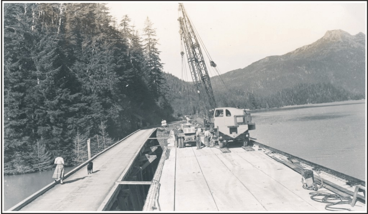
Figure 164. The Eyak River Bridge (right), the first prestressed concrete bridge built in Alaska, nearing completion, August 1954. The old CR&NW trestle bridge, which was converted to automobile use in the late 1940s, is at left. BPR photo courtesy of ADOT&PF Bridge Section, Juneau.
