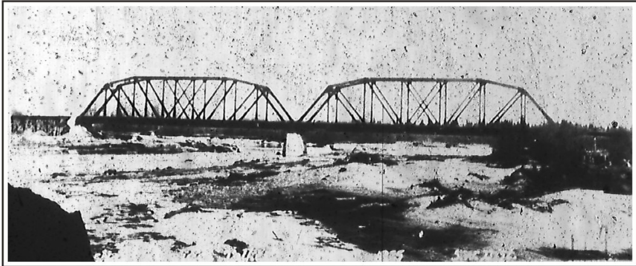
Figure 117. The two span camelback steel truss bridge at Resurrection Creek on the Seward Highway, 1935. U.S. Alaska Road Commission Collection, PCA 61-10-419, Alaska State Library.
