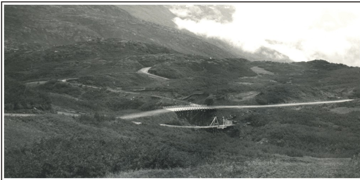
Figure 133. The new timber trestle bridge and the old “A” truss bridge at Ptarmigan Drop at Mile 32 of the Richardson Highway, August 25, 1944. U.S. Alaska Road Commission Collection, PCA 61-21-139, Alaska State Library.
