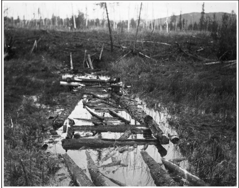
Figure 52. A collapsed bridge at Mile 88 of the WAMCATS Line, August 1913. Rita Cottnair Collection, 1974-130-130, University of Alaska Fairbanks.
