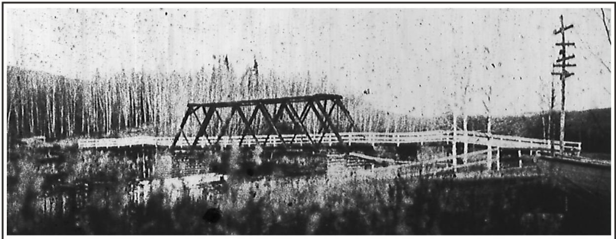
Figure 90. The Hot Springs Slough Howe timber truss bridge, October 24, 1938. U.S. Alaska Road Commission Collection, PCA 61-12-468, Alaska State Library.
