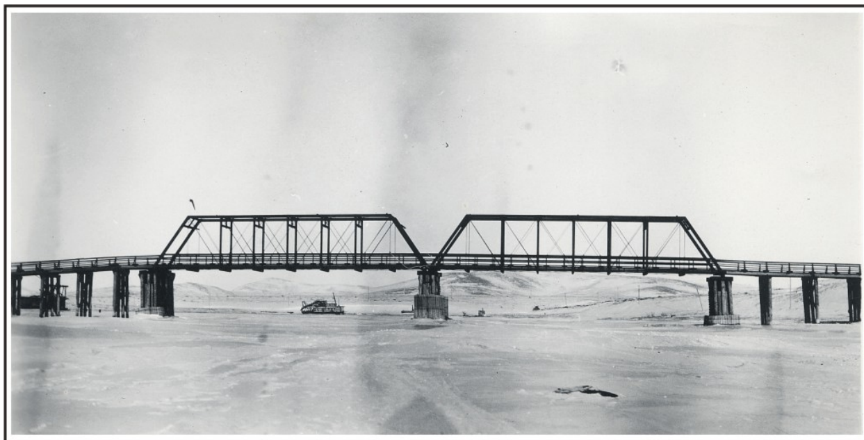
Figure 49. The Snake River Bridge, a two span Pratt timber truss, built in 1916. U.S. Alaska Road Commission Collection, PCA 61-141-7, Alaska State Library.
