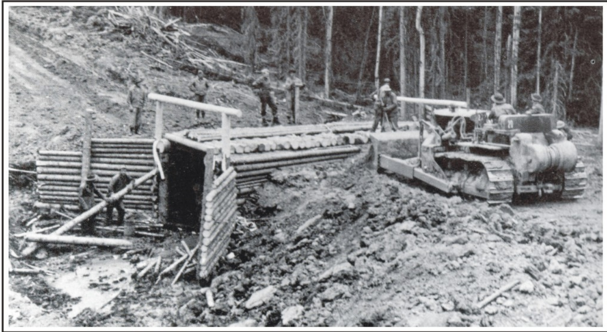
Figure 138. Army engineers from the 35 th Engineers Battalion constructing a log culvert on the Alaska Highway, 1942. Photo from the Chief of Engineers, Office of History, U.S. Army, reprinted from Twitchell 1992:144.
