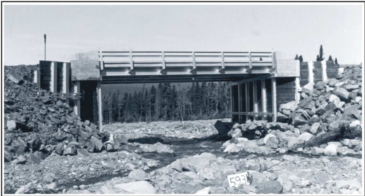
Figure 156. The single span steel I-beam bridge at Bear Creek on the Richardson Highway, built in 1952. The bridge was designed using standard plans. Photo by Larry A. Carlson, July 13, 1962, ADOT&FP Bridge Design Section, Juneau.
