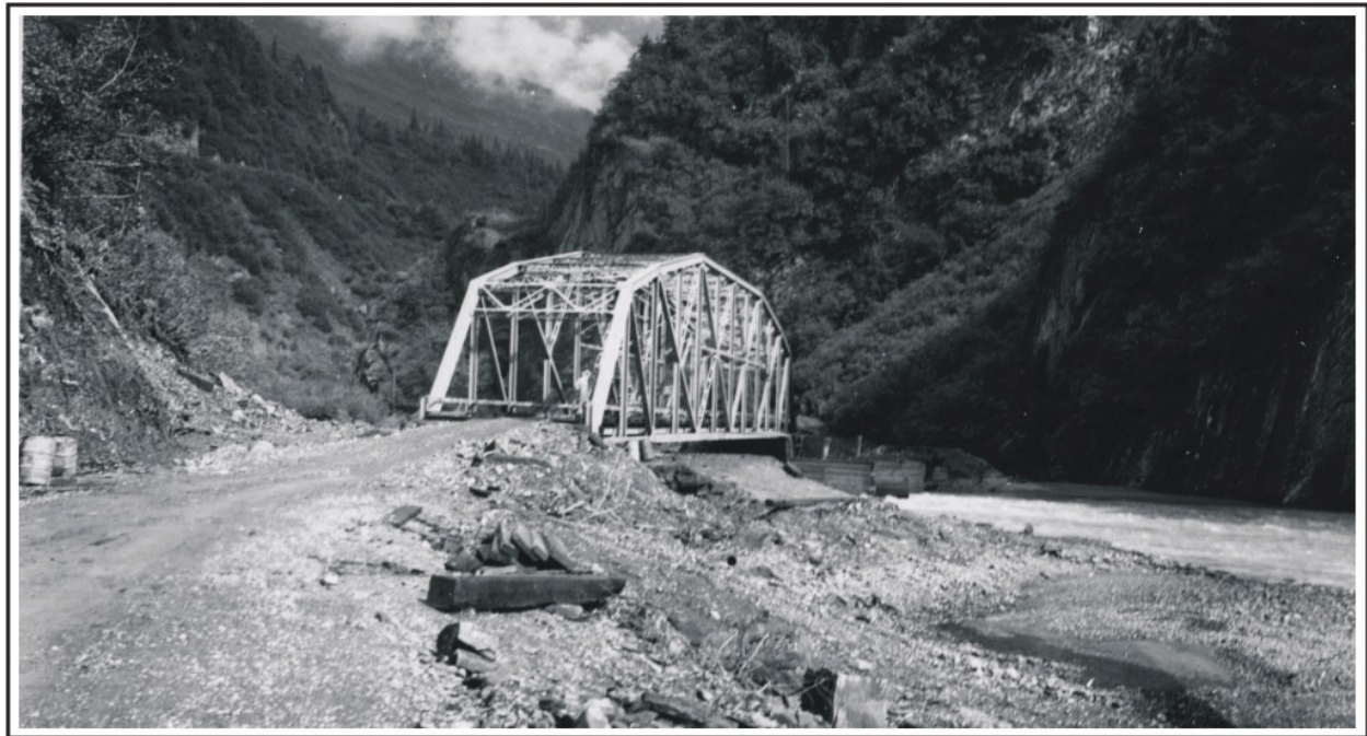
Figure 145. The camelback truss bridge, lower crossing of the Lowe River, on the Richardson Highway, 1946. U.S. Alaska Road Commission Collection, PCA 61-21-39, Alaska State Library.
