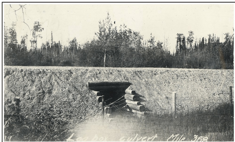
Figure 73. An ARC timber culvert on the Richardson Highway, 1920s. U.S. Alaska Road Commission Collection, PCA 61-12-25, Alaska State Library.
