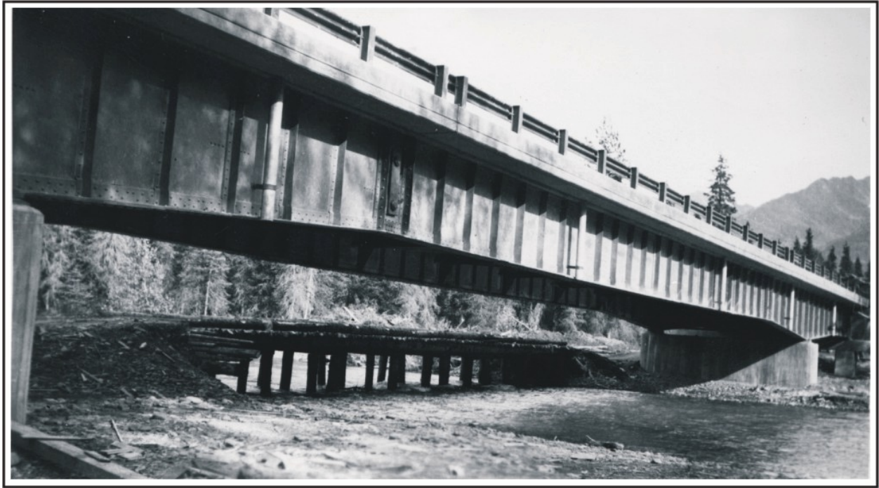
Figure 153. The two-span steel girder bridge at East Fork of Sixmile Creek on the Seward Highway, September 1949. U.S. Alaska Road Commission Collection, PCA 61-29-181, Alaska State Library.
