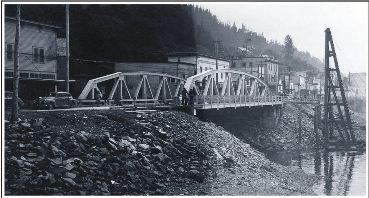
Figure 144. The steel pony truss bridge at Ketchikan Creek, downtown Ketchikan, June 9, 1945. U.S. Alaska Road Commission Collection, PCA 61-89-10, Alaska State Library.
