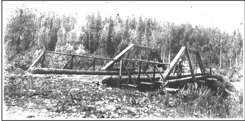
Figure 64. A queen post bridge at Moose Creek at Mile 12 of the Talkeetna-Cache Creek Road, 1920s. U.S. Alaska Road Commission Collection, PCA 61-10-11, Alaska State Library.
