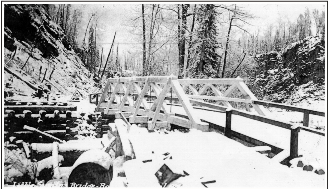
Figure 55. A "Type B" ARC standard bridge, 1920s. This pony truss bridge was located at the Little Susitna River at Mile 12.2 of the Wasilla-Fishhook Road. U.S. Alaska Road Commission Collection, PCA 61-9-54, Alaska State Library.
