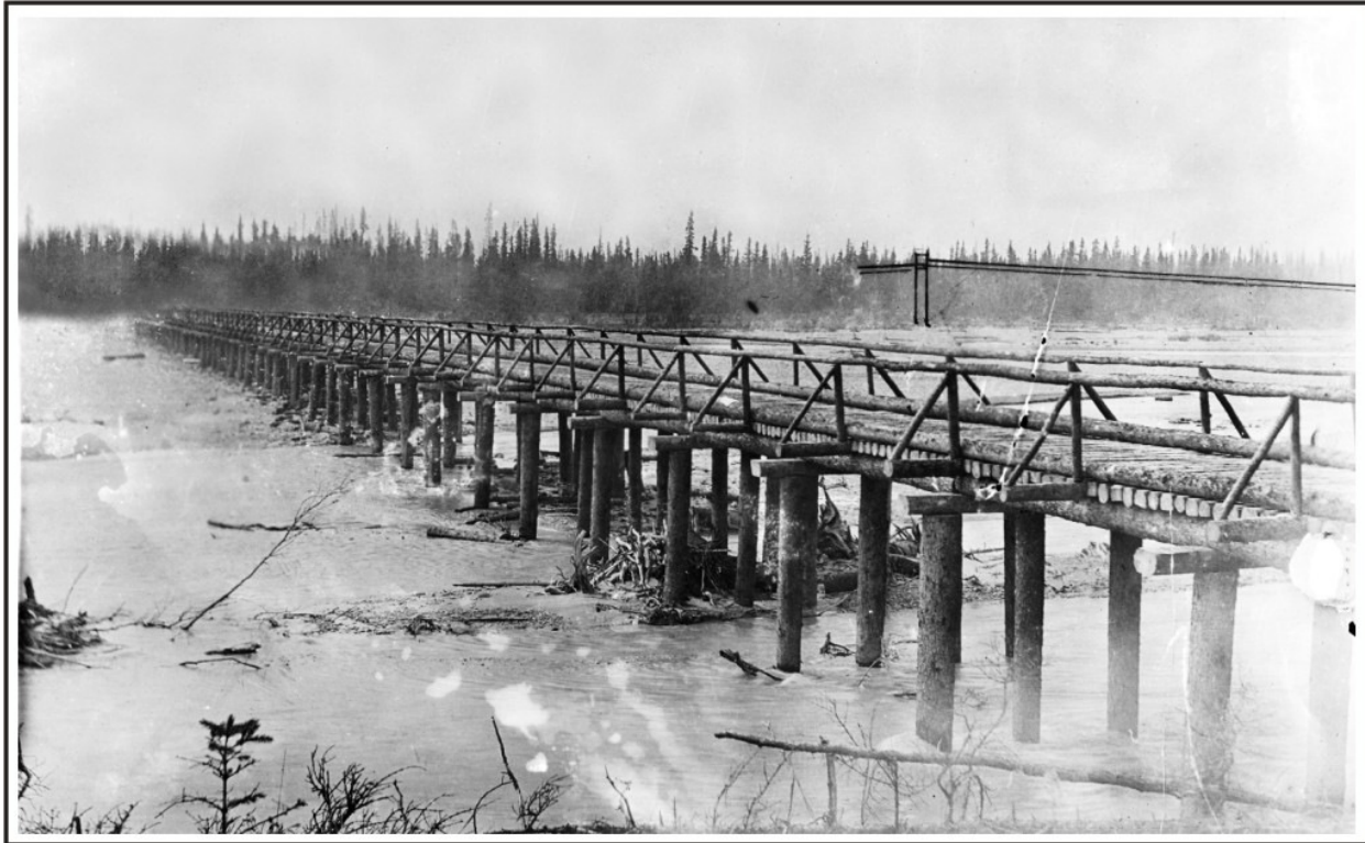
Figure 41. A log bridge supported by pile bents at Jarvis Creek on the Valdez-Fairbanks Trail, 1910. Rita Cottnair Collection, 1974-130-42, University of Alaska Fairbanks.
