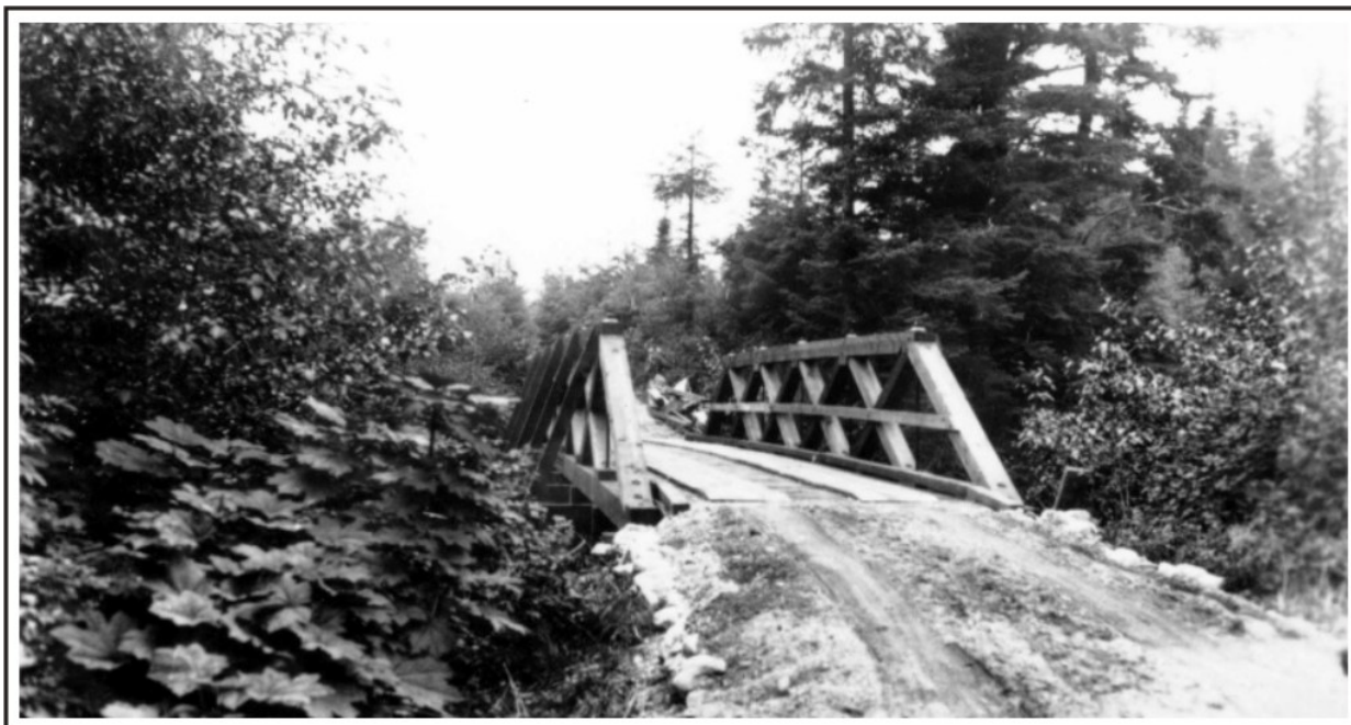
Figure 58. The Indian River Bridge, a timber pony truss, at Sitka, July 14, 1929. Estelle and Phillip Georges Collection, HMC-0381 series 2-7-2, University of Alaska Anchorage.
