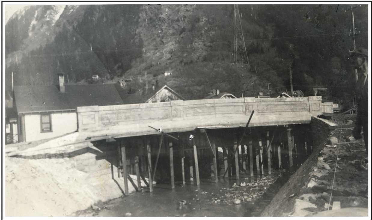
Figure 124. The concrete girder bridge under construction at Gold Creek on Ninth Street in Juneau, 1934. U.S. Alaska Road Commission Collection, PCA 61-14-130, Alaska State Library.
