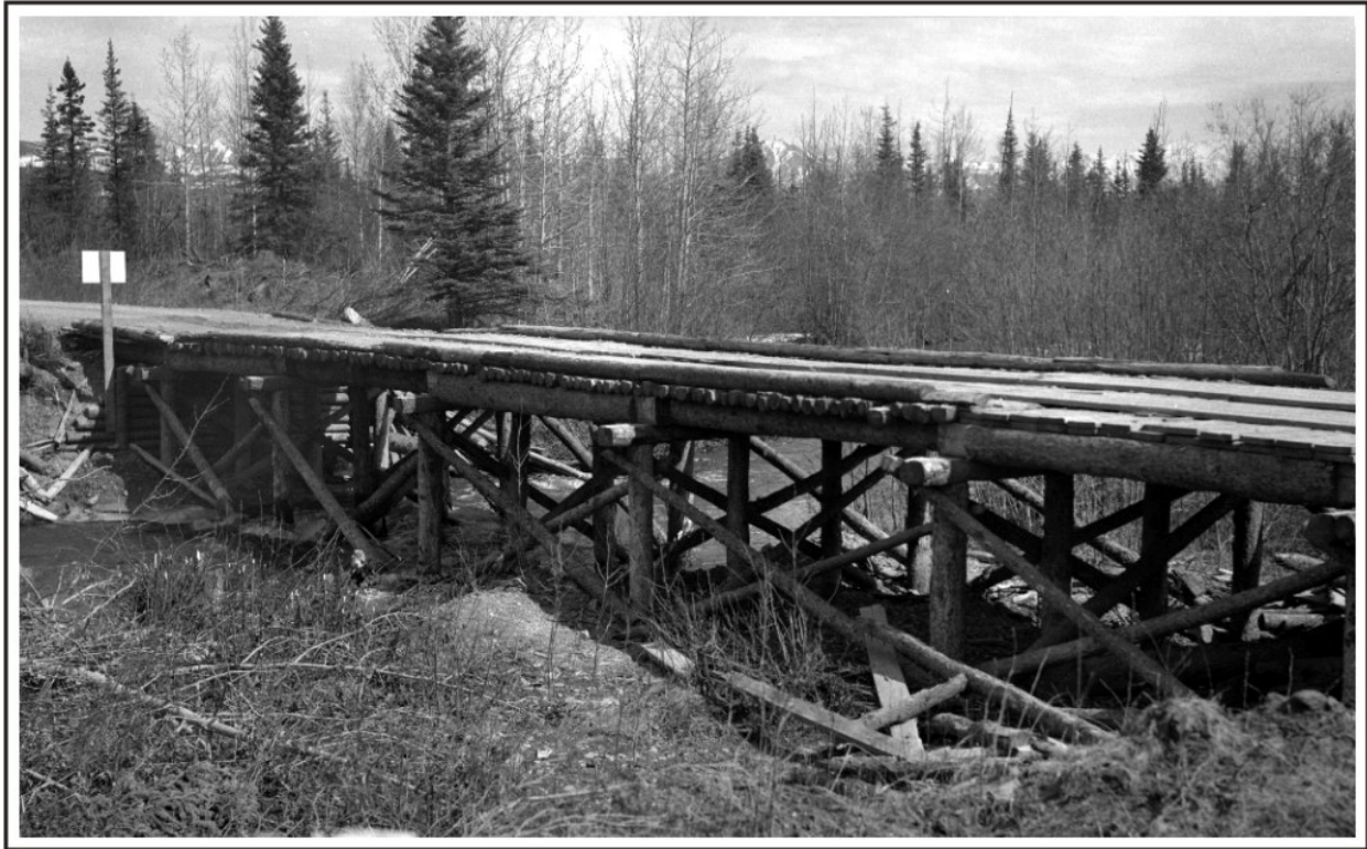
Figure 142. The timber trestle bridge at Porcupine Creek on the Tok Cut-off Highway, May 1949, was typical of one-lane timber trestle bridges built during World War II. U.S. Alaska Road Commission Collection, PCA 61-23-78, Alaska State Library.
