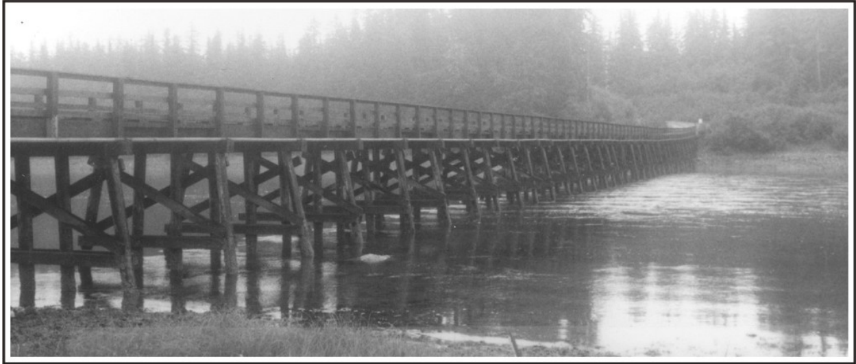
Figure 188. The treated timber trestle bridge built by the U.S. Coast Guard at Ankau Slough, July 28, 1971. Photo by Michael Murray and Robert Lium, ADOT&PF Bridge Section, Juneau.
