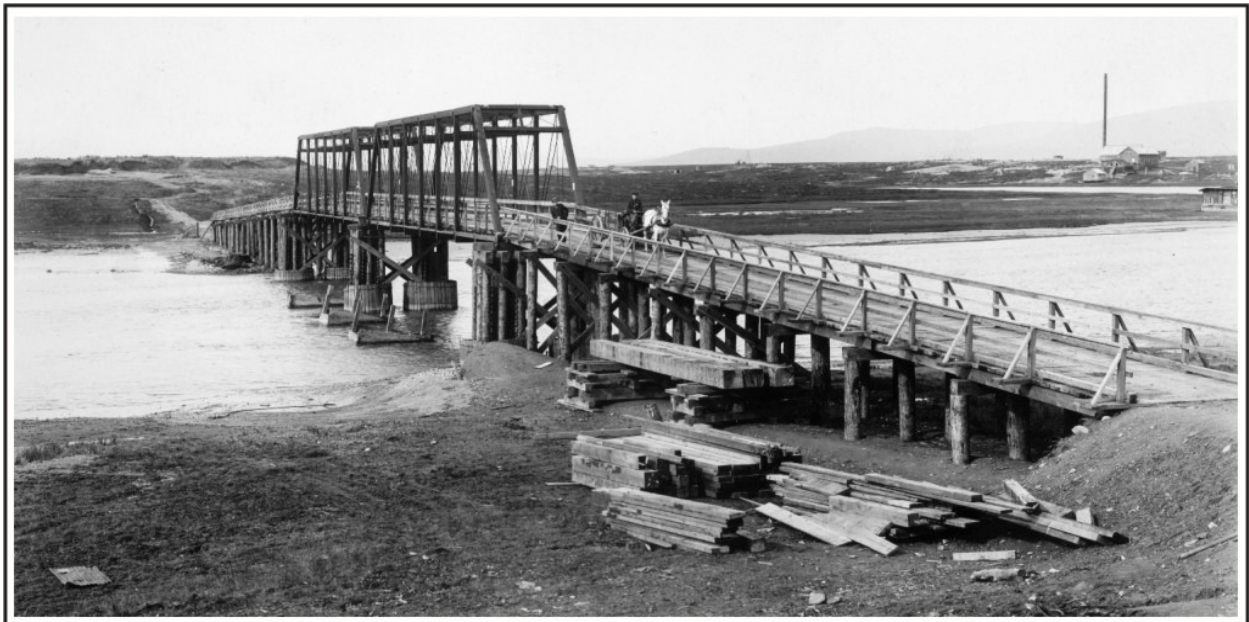
Figure 46. The Snake River Bridge, a two span Pratt through truss structure near Nome, early 1900s. John Zug Collection, 1980-68-333, University of Alaska Fairbanks.
