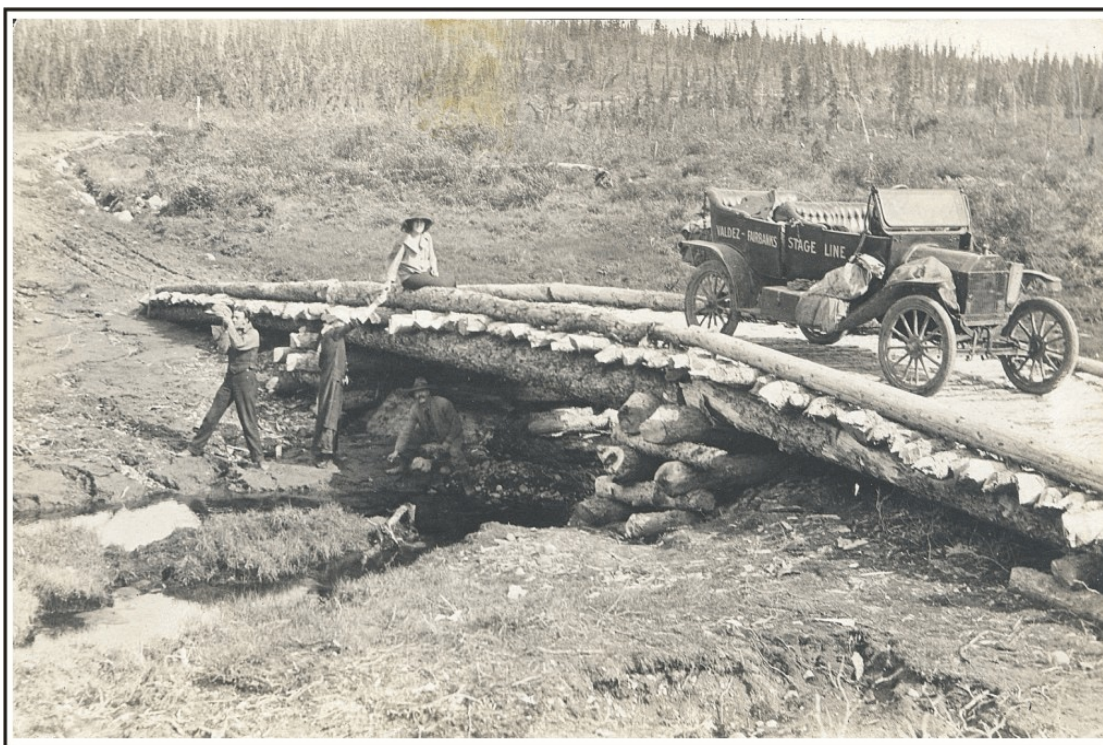
Figure 38. A log stringer bridge on the Valdez-Fairbanks Road, 1910. Note the cribbed log piers. U.S. Alaska Road Commission Collection, PCA 228-225, Alaska State Library.
