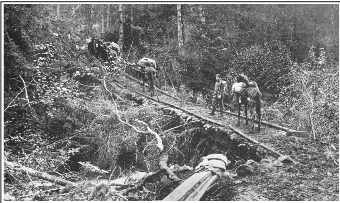
Figure 21. A log pack horse bridge, Porcupine Creek, White Pass Trail, seven miles north of Skagway, 1897. Frank LaRoche photo, Klondike Gold Rush National Park, Skagway.
