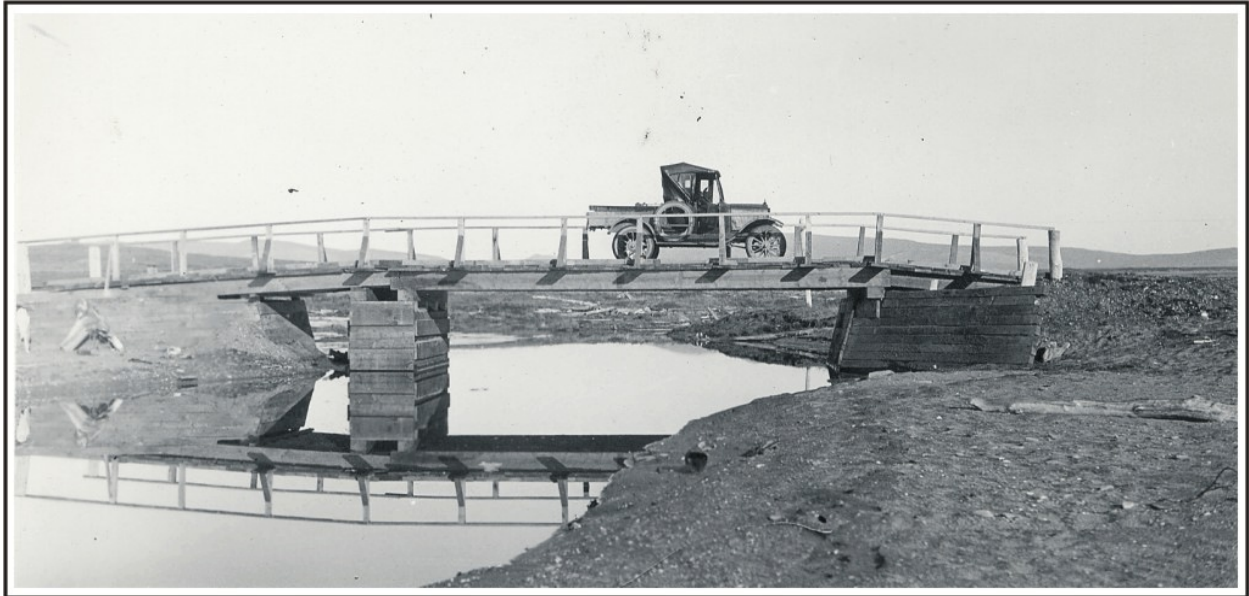
Figure 39. A timber stringer bridge on Peluk Creek near Nome, late 1910s. U.S. Alaska Road Commission Collection, PCA 61-141-21, Alaska State Library.
