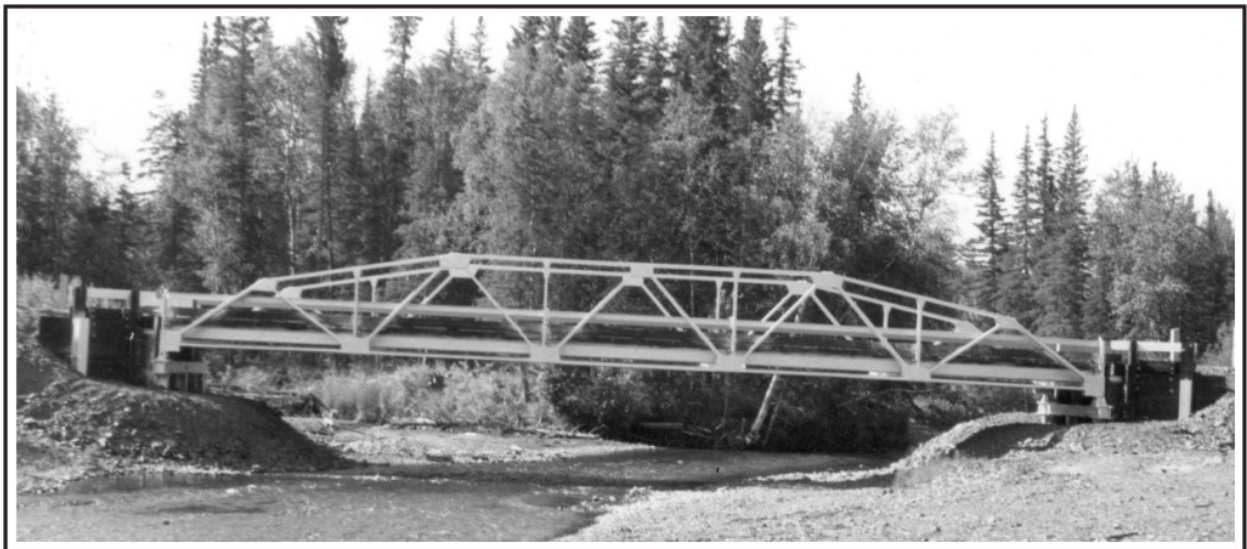
Figure 183. The old Phelan Creek steel pony truss bridge after it was re-erected at Hutlinana Creek on the Elliott Highway, October 1961. Photo courtesy of ADOT&PF Bridge Section, Juneau.
