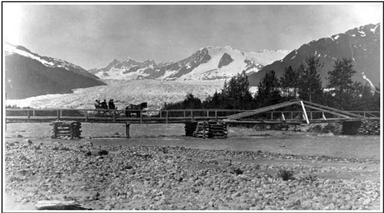
Figure 48. The king post truss bridge over the Mendenhall River, about 1916. Winter and Pond Collection, PCA 87-1887, Alaska State Library.
