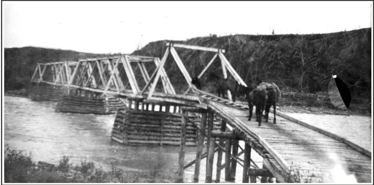
Figure 45. The Tanana River Bridge, consisting of two Howe truss spans, a king post span and pile trestle approach, 1908. Francis E. Pope Collection, 1966-15-480, University of Alaska Fairbanks.
