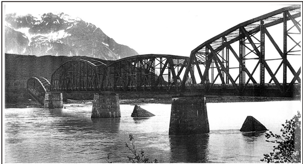
Figure 196. The south end of the north span of the Million Dollar Bridge dropped into the Copper River during the 1964 Earthquake. Photo courtesy of ADOT&PF Bridge Section, Juneau.
