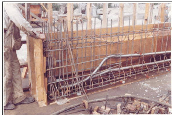
Figure 179. Building the forms for a concrete girder for the Kashwitna River Bridge, July 16, 1962. Photo courtesy of ADOT&PF Bridge Section, Juneau.
