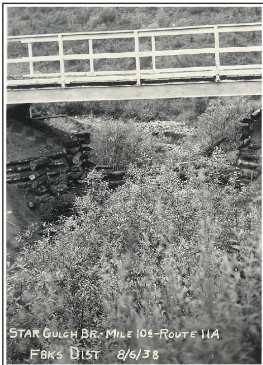
Figure 101. The steel stringer bridge at Star Gulch, August 6, 1938. U.S. Alaska Road Commission Collection, PCA 61-13-396, Alaska State Library.
