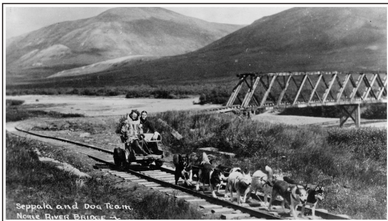
Figure 76. Leonard Seppala with a dog team and pupmobile on the Nome-Shelton Tramway. The Nome River Bridge, a Howe timber truss structure built by the ARC in 1924, is in the background at right. Photo courtesy of ADOT&PF Bridge Section, Juneau.
