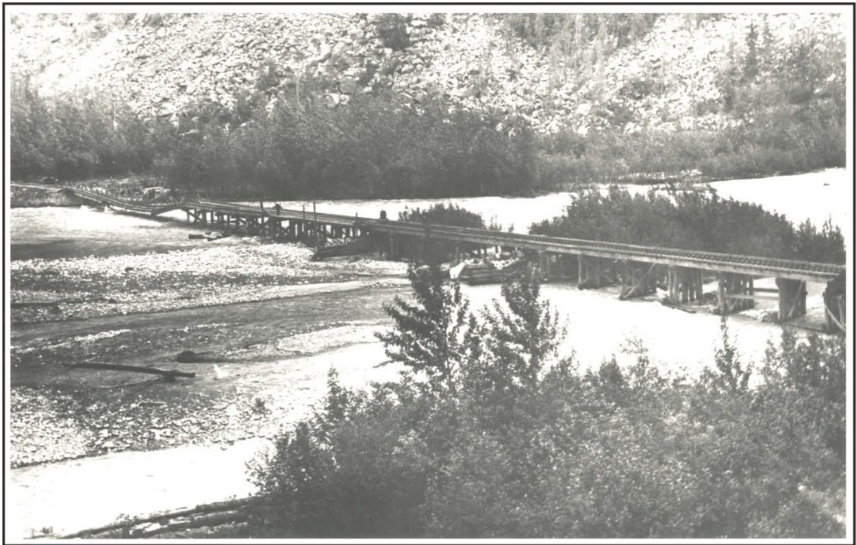
Figure 26. A damaged WP&YR timber trestle bridge at Mile 4 after the 1901 Skagway River flood. H.D. Barley Collection, Photo #5226, Yukon Archives, Whitehorse.
