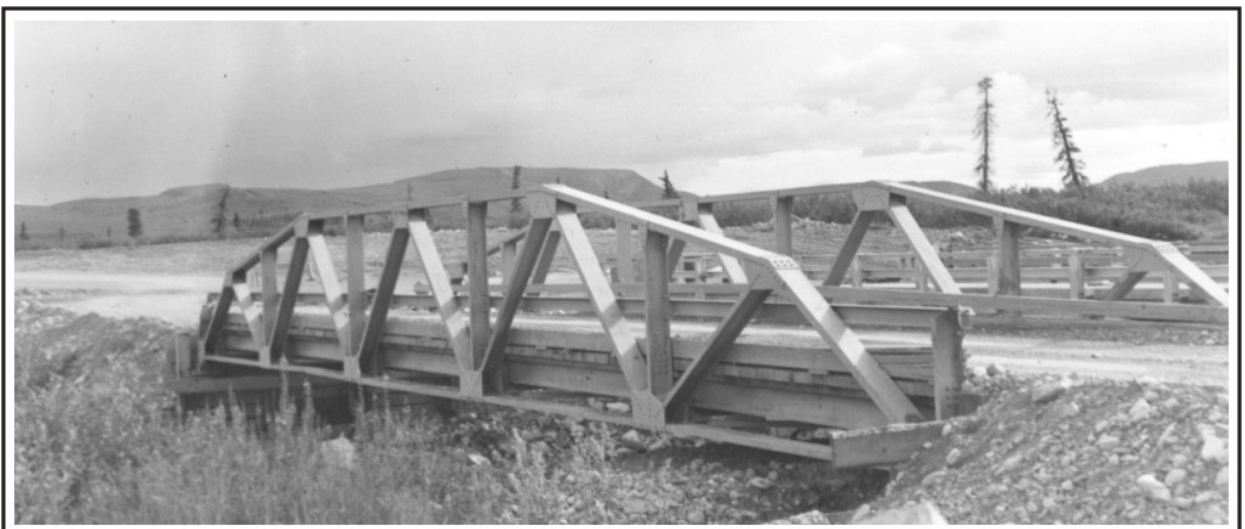
Figure 131. Steel pony truss bridge erected at Phelan Creek on the Richardson Highway in 1943. Photo by L.D. Bruesch, August 1958, courtesy of ADOT&PF Bridge Design Section, Juneau.
