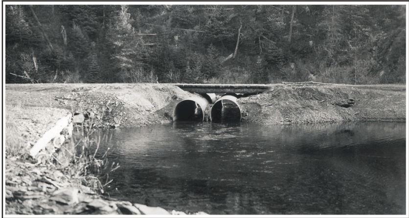
Figure 107. A temporary timber stringer bridge over two metal culverts, Mile 9 of the Seward Highway, October 17, 1937. U.S. Alaska Road Commission Collection, PCA 61-66-22, Alaska State Library.
