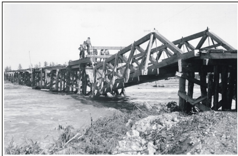
Figure 65. Collapsed pony timber truss bridge, 1920s. Location unknown. Photo courtesy of Candy Waugaman, Fairbanks.
