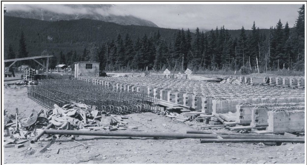
Figure 163. Precast concrete stringers for BPR bridges on the Seward Highway, July 1951. U.S. Alaska Road Commission Collection, PCA 61-94-33, Alaska State Library.
