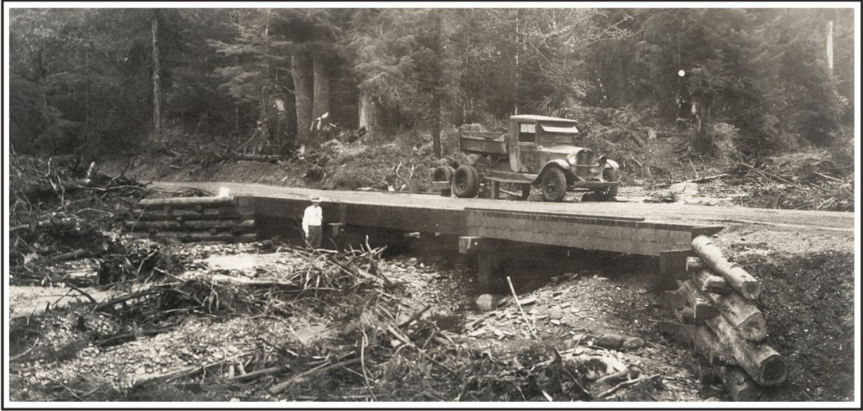
Figure 113. A timber stringer bridge at Bird Creek on the Wrangell Highway, August 10, 1930. U.S. Alaska Road Commission Collection, PCA 61-59-143, Alaska State Library.
