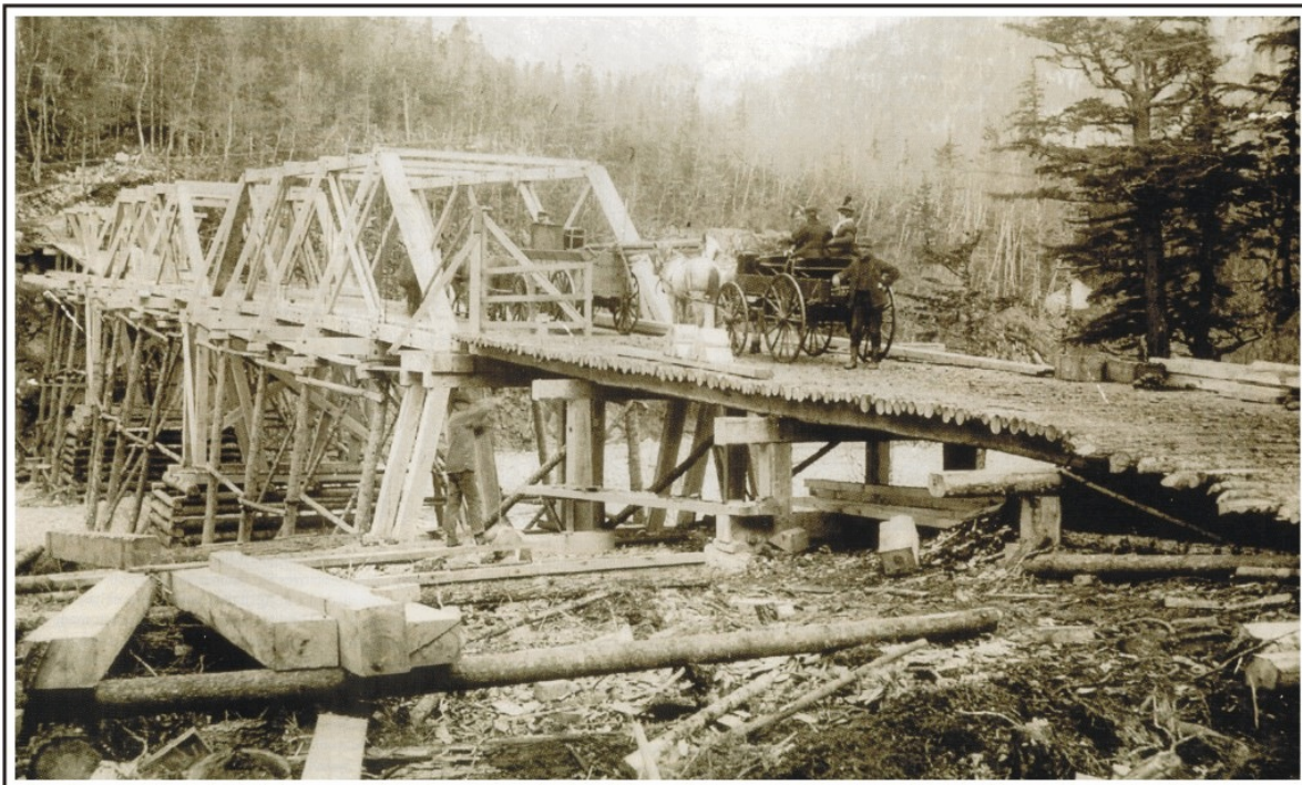
Figure 23. Timber through truss bridge over the Skagway River on the Brackett Wagon Road, 1898. E.A. Hegg photo, BW 19-1-155, Klondike Gold Rush National Park, Skagway.
