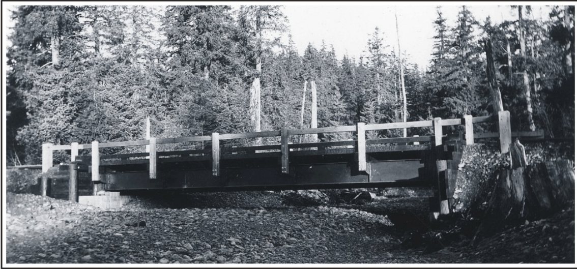
Figure 115. The steel I-beam bridge at Heney Creek on Point Whiteshed Road at Cordova, 1937. U.S. Alaska Road Commission Collection, PCA 61-54-151, Alaska State Library.
