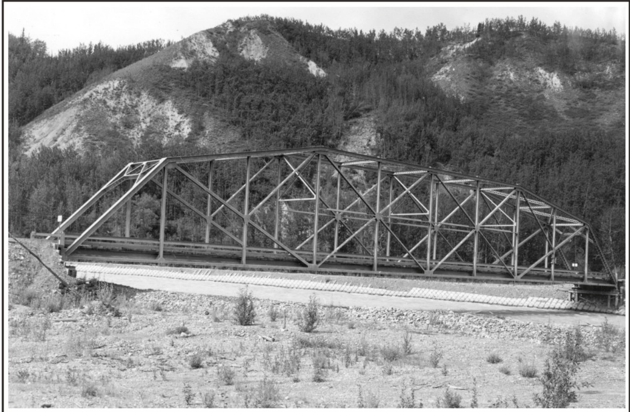
Figure 130. The steel camelback truss bridge built in 1942-1943 at Tonsina River on the Richardson Highway. Photo courtesy of ADOT&PF Bridge Section, Juneau.
