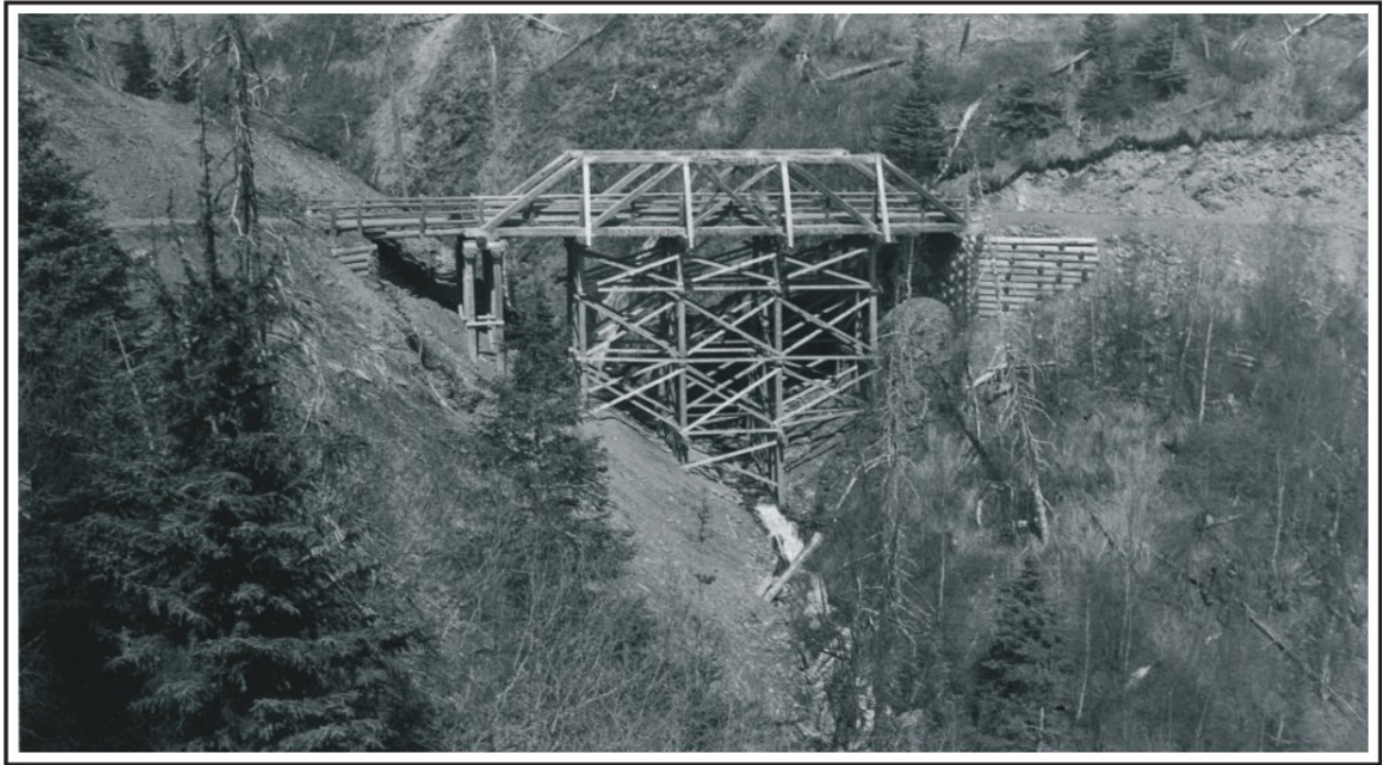
Figure 79. The timber Parker truss bridge at Frenchy Creek on the Moose Pass-Hope Road, May 1936. U.S. Alaska Road Commission Collection, PCA 61-70-102, Alaska State Library.
