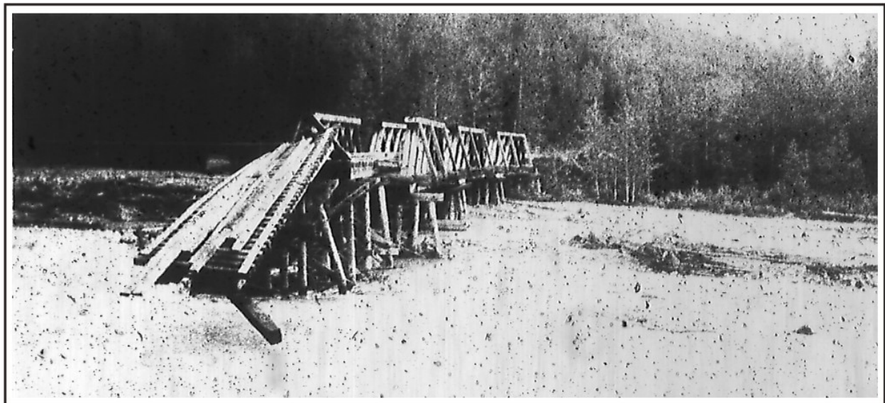
Figure 111. Damage to the Sutton-Chickaloon King River Bridge, a railroad bridge converted for automobiles, after flooding, September 4, 1934. U.S. Alaska Road Commission Collection, PCA 61-11-265, Alaska State Library.
