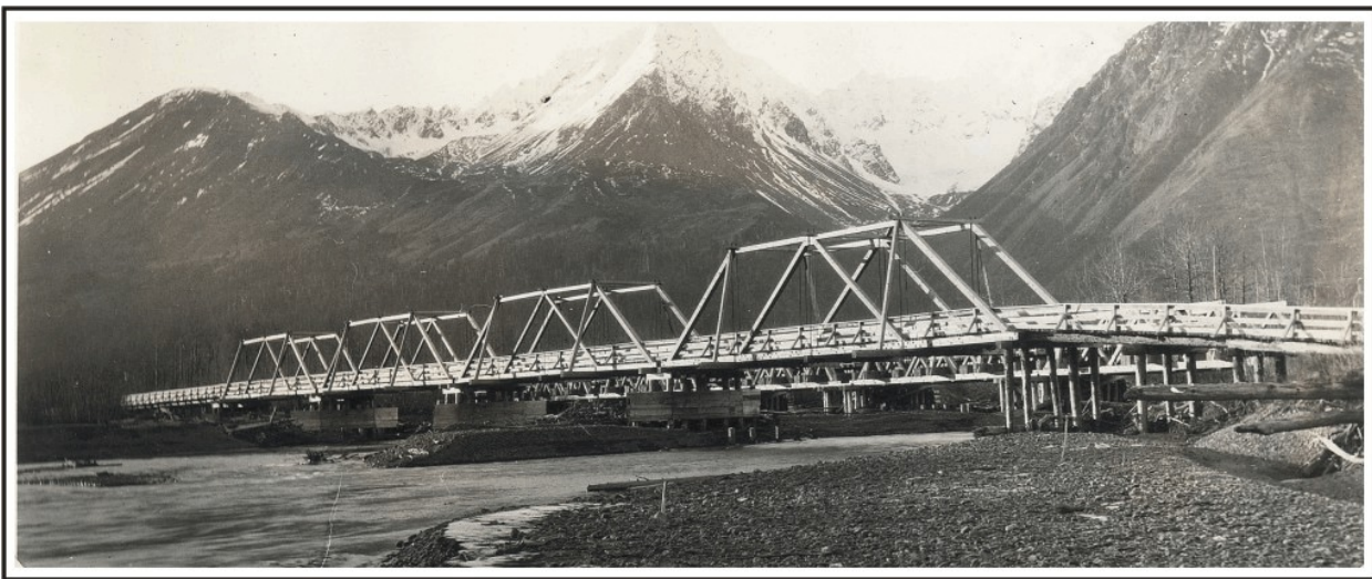
Figure 78. The four-span Howe truss Resurrection River Bridge at Mile 3 of the Seward-Kenai Lake Road, November 1926. This bridge was built by the BPR in the mid-1920s. C.F. Wyller, photographer, U.S. Alaska Road Commission Collection, PCA 61-65-127, Alaska State Library.
