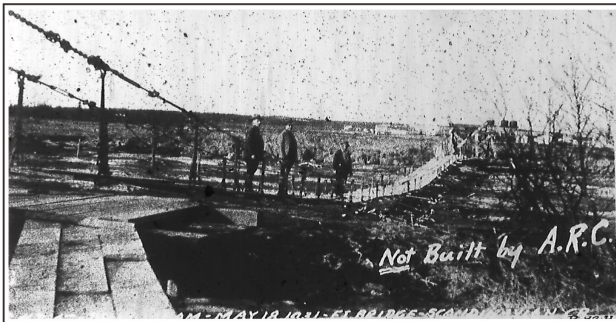
Figure 109. A suspension footbridge built by miners at Scandinavian Creek in the Innoko District, May 18, 1931. U.S. Alaska Road Commission Collection, PCA 61-11-13, Alaska State Library.
