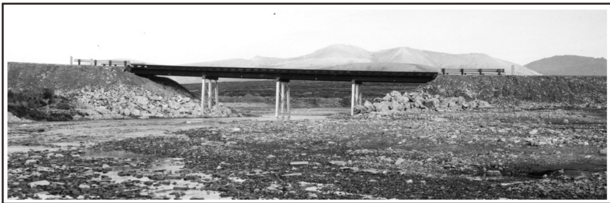
Figure 177. The laminated timber stringer bridge at Cripple Creek, 1963. Photo by the contractor, courtesy of ADOT&PF Bridge Section, Juneau.
