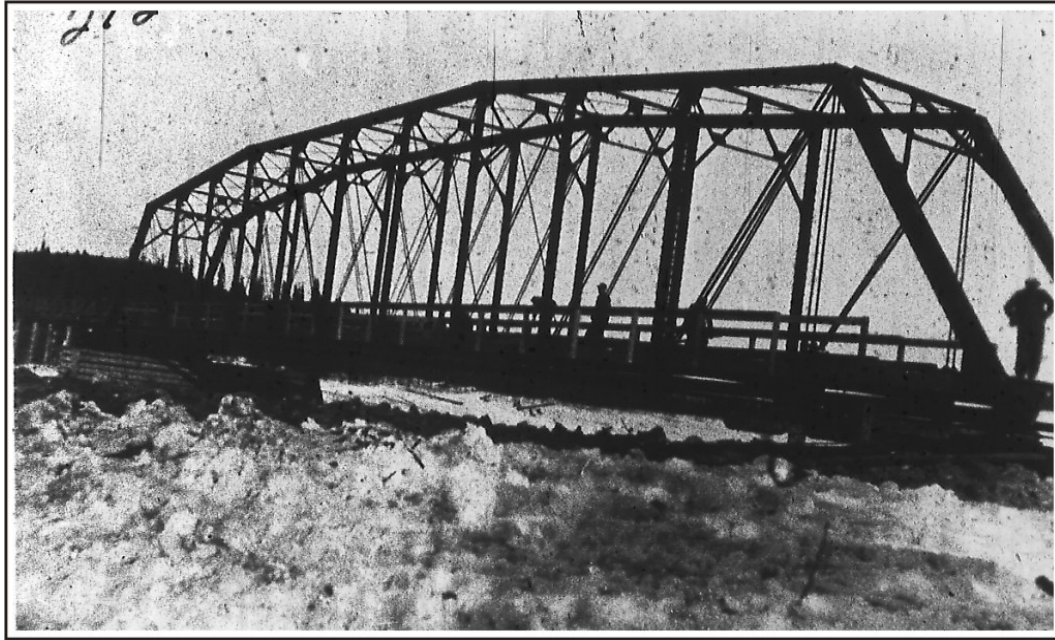
Figure 60. The Salcha River Bridge, an all-steel 180-foot Camelback truss span with 345 feet of trestle approach, at Mile 331 of the Richardson Highway, 1925. U.S. Alaska Road Commission Collection, PCA 61-12-273, Alaska State Library.
