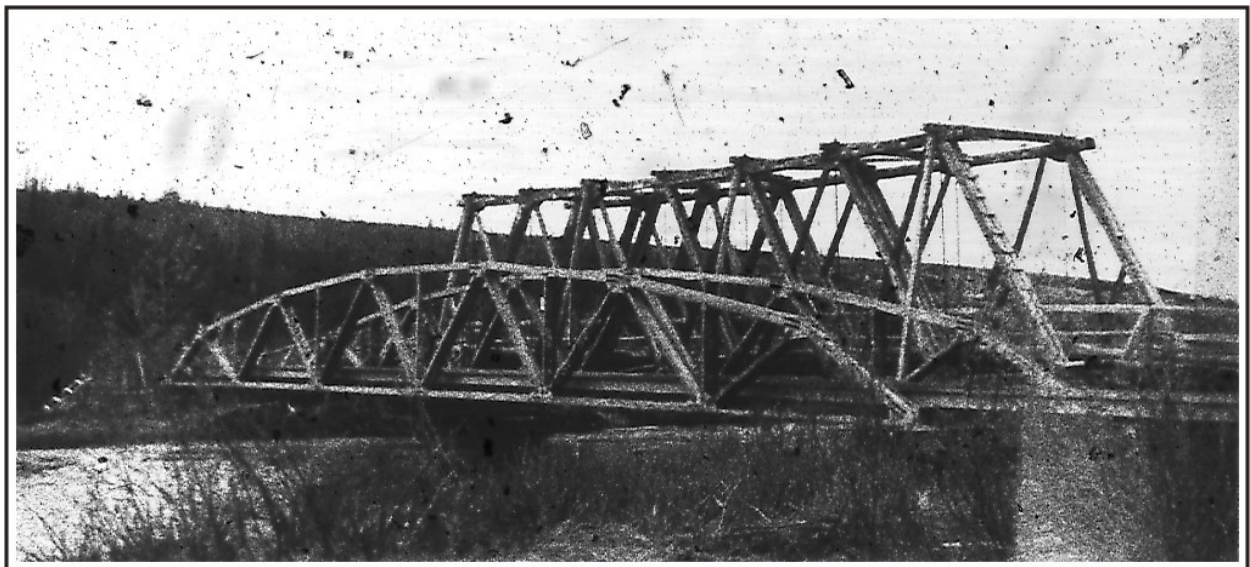
Figure 97. The steel pony bridge at Ganes Creek, 1937. The old timber Howe truss is in the background. U.S. Alaska Road Commission Collection, PCA-16-1-07, Alaska State Library.
