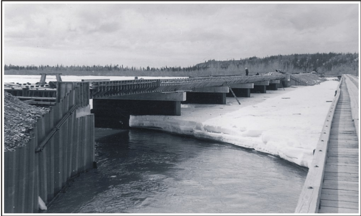
Figure 158. One of the two 330-foot multi-span steel stringer bridges at the Chistochina River under construction, May 14, 1955. The old timber trestle bridge is at right. U.S. Alaska Road Commission Collection, PCA 61-23-112, Alaska State Library.
