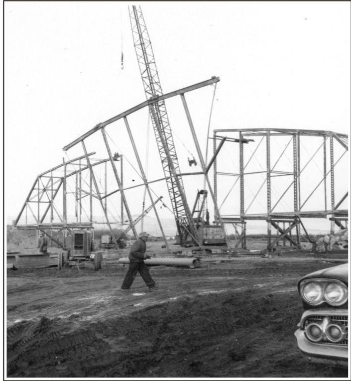
Figure 182. A crew re-erecting the old Cushman Street Bridge at the Kuzitrin River, September 1960. Photo courtesy of ADOT&PF Bridge Section, Juneau.
