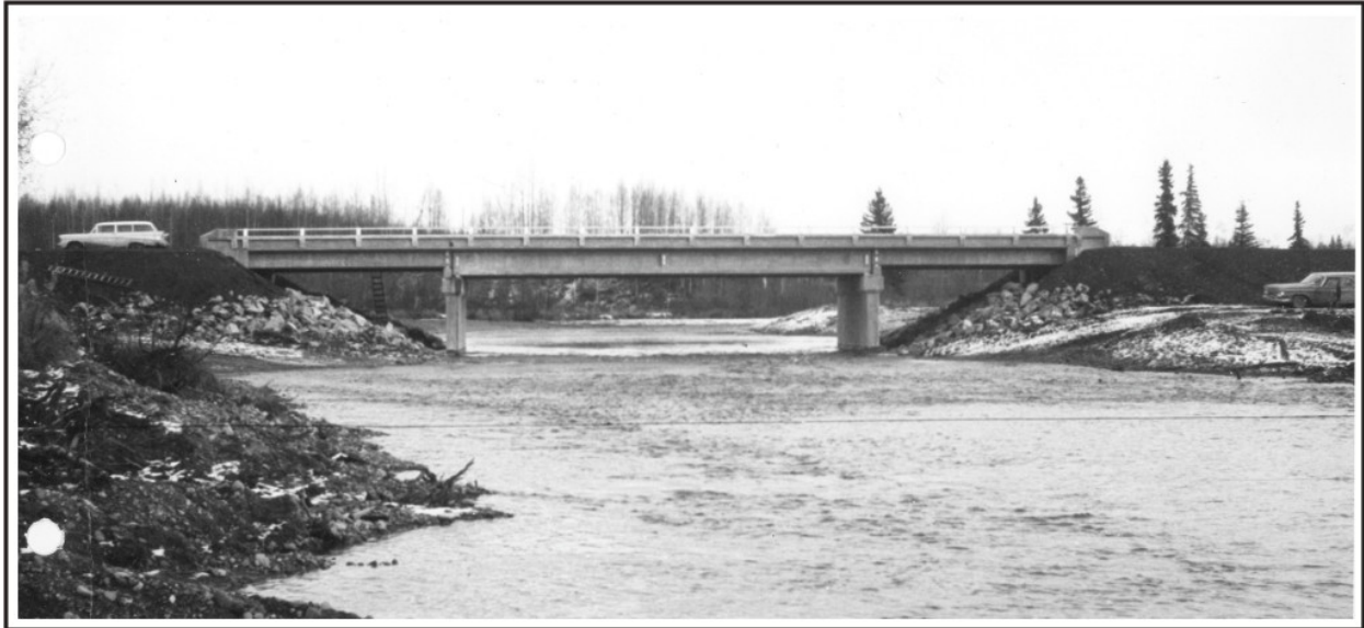
Figure 178. The prestressed concrete girder bridge at Sheep Creek on the Palmer-Cantwell Highway, 1963. Photo by M-B Construction Company, Seattle, courtesy of ADOT&PF Bridge Section, Juneau.
