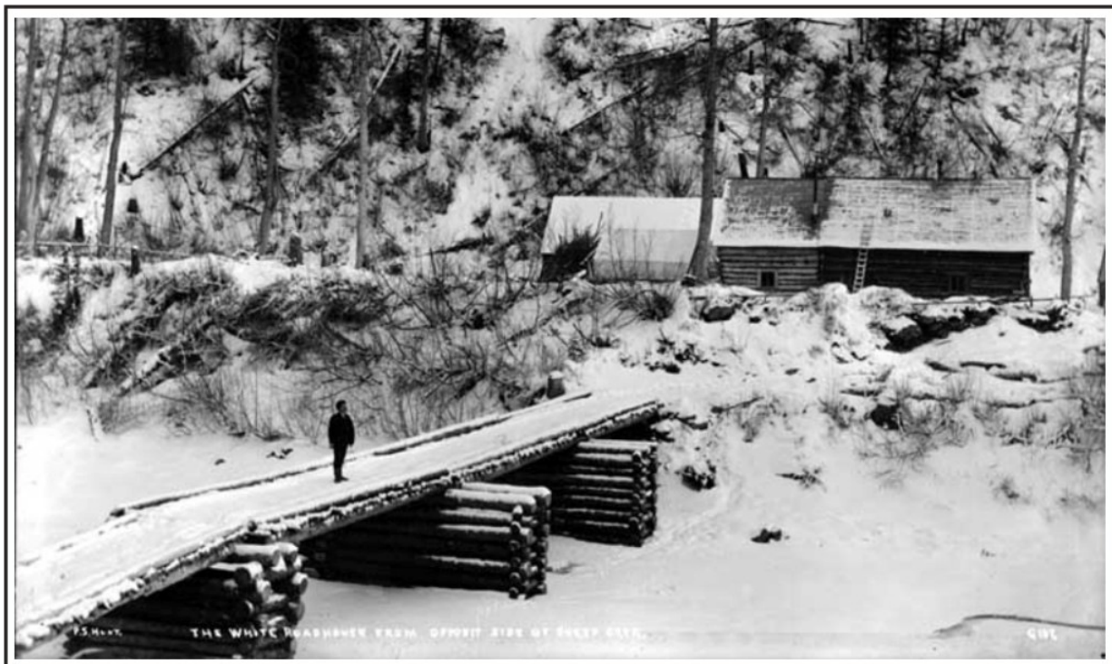
Figure 40. A log bridge with log cribbed piers at Sheep Creek on the Valdez-Fairbanks Trail. White's Roadhouse is in the background. Crary-Henderson Collection, B62-1-a-426, Anchorage Museum of History and Art.
