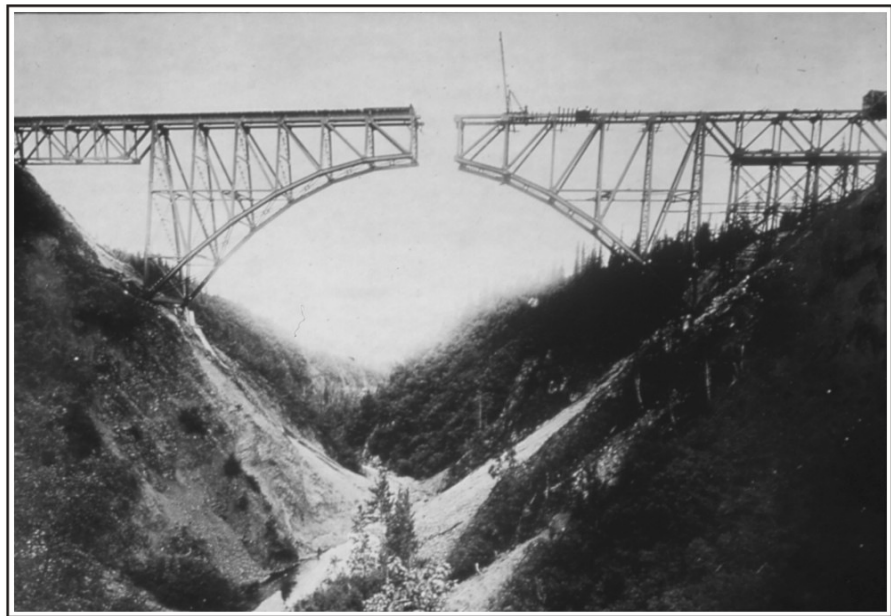
Figure 29. The steel arch Hurricane Gulch railroad bridge during construction by the AEC, August 1921. Photo courtesy of the ADOT&PF Bridge Section, Juneau.
