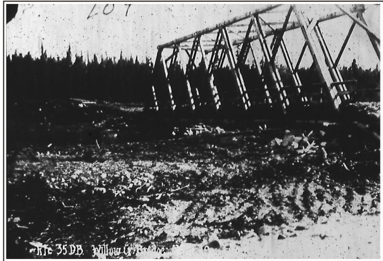
Figure 110. Howe timber truss bridge at Willow Creek on the Willow Station-Lucky Shot Road, 1934. U.S. Alaska Road Commission Collection, PCA 61-9-104, Alaska State Library.
