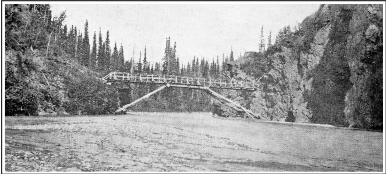
Figure 67. The Bull River Bridge, a log arch span, on the pack trail near Colorado Station. U.S. Alaska Road Commission Collection, PCA 61-11-38, Alaska State Library.
