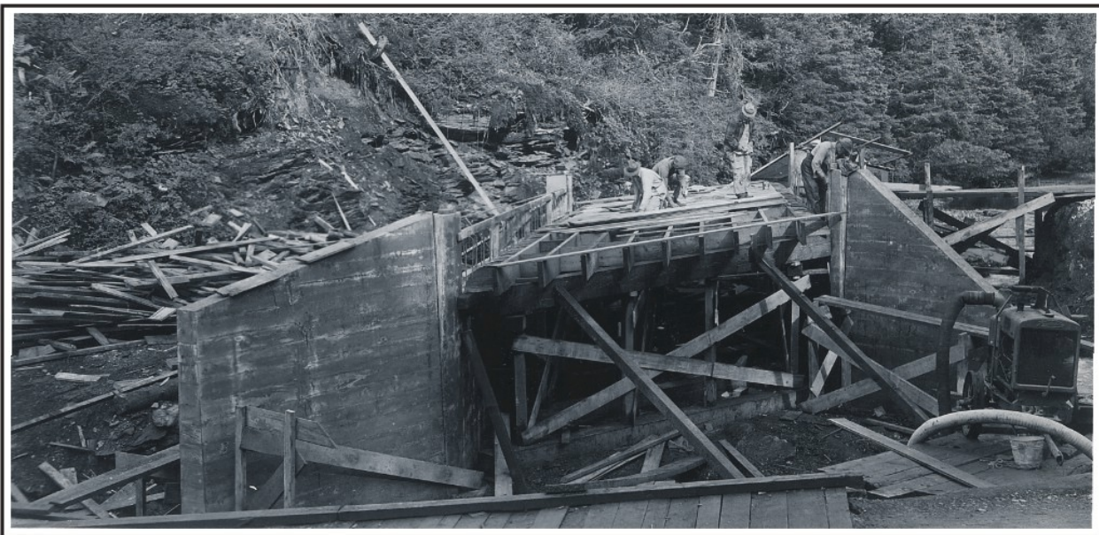
Figure 120. Workers finishing forms for the concrete deck slab on Bridge Station 106 at Mile 8.4 of the Seward Highway, October 1937. Photograph by F.E. Swartz, U.S. Alaska Road Commission Collection, PCA 61-66-43, Alaska State Library.
