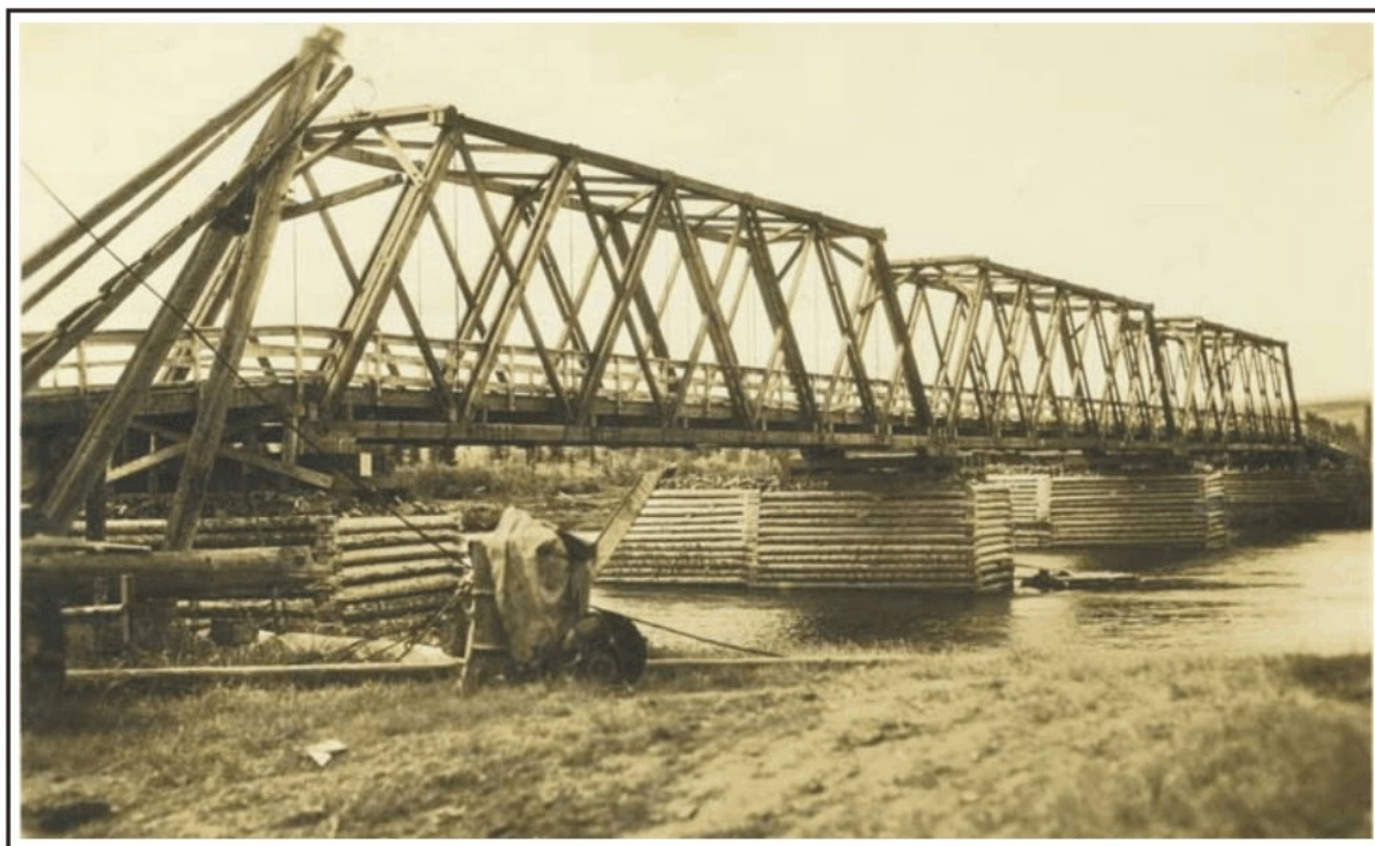
Figure 59. The Birch Creek Howe timber truss bridge on the Fairbanks-Circle Road, 1920s. Skinner Foundation, PCA 44-02-220, Alaska State Library.
