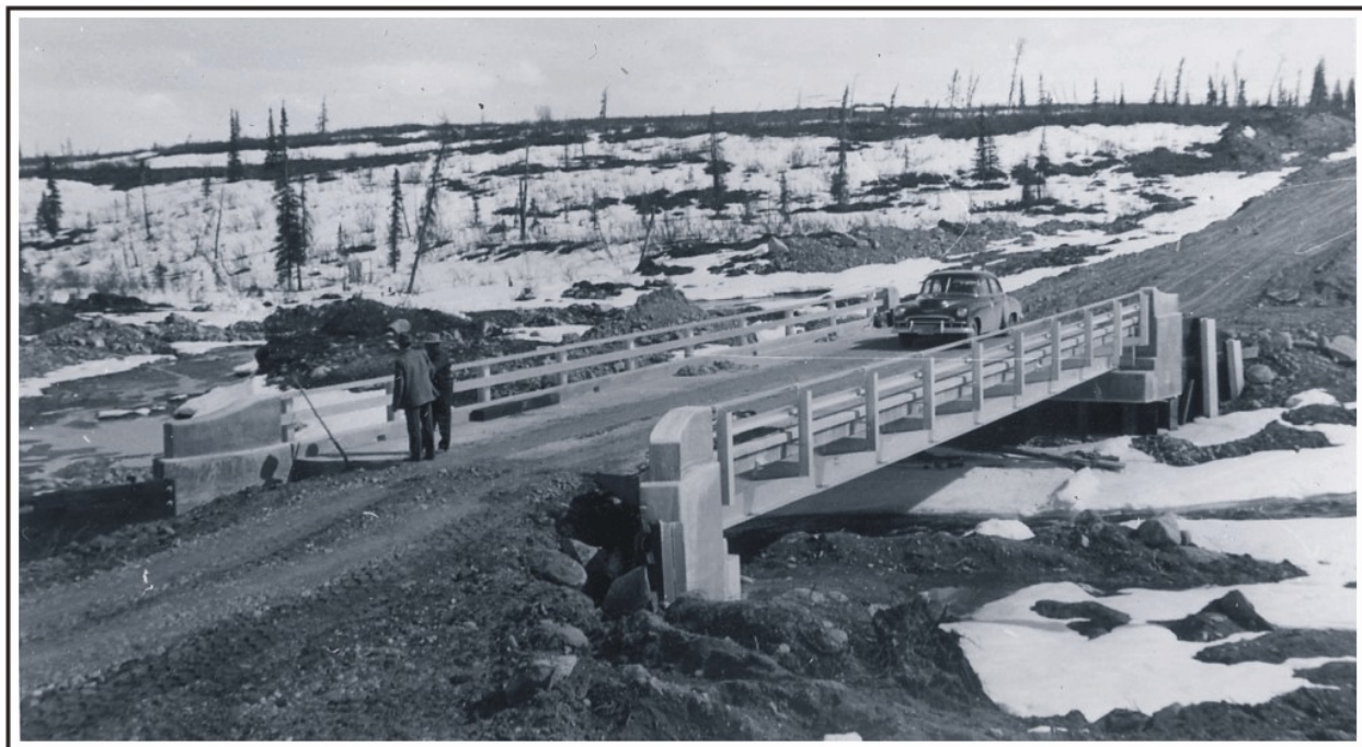
Figure 160. Steel I-beam bridge at Brushkana River on the Denali Highway, May 20, 1955. U.S. Alaska Road Commission Collection, PCA 61-18-72, Alaska State Library.
