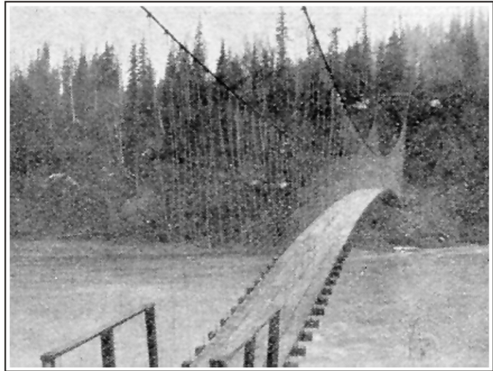
Figure 69. The Chulitna River Bridge near Honolulu Creek, a 360-foot suspension span. U.S. Alaska Road Commission Collection, PCA 61-11-49, Alaska State Library.
