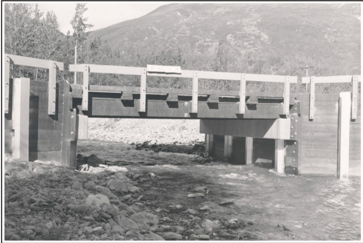
Figure 155. The Boulder Creek Bridge, one of four standard single span treated timber bridges built on the Richardson Highway in 1953. Photo courtesy of ADOT&PF Bridge Section, Juneau.
