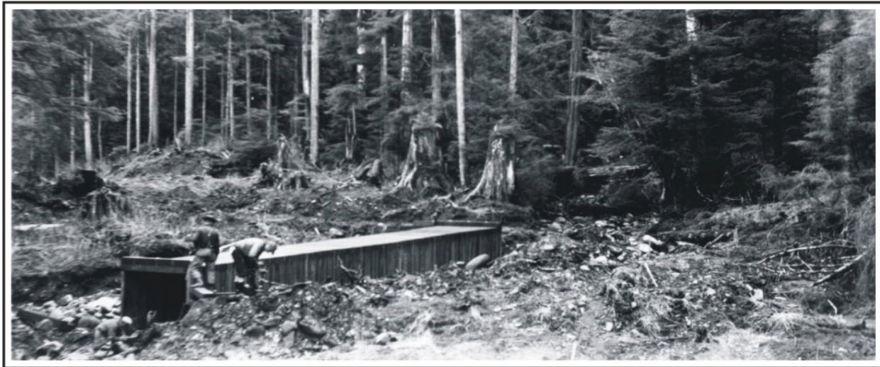
Figure 119. A BPR crew building a timber box culvert on the Wrangell Highway, 1939. Photo by Mr. Cohn. U.S. Alaska Road Commission Collection, PCA 61-59-33, Alaska State Library.
