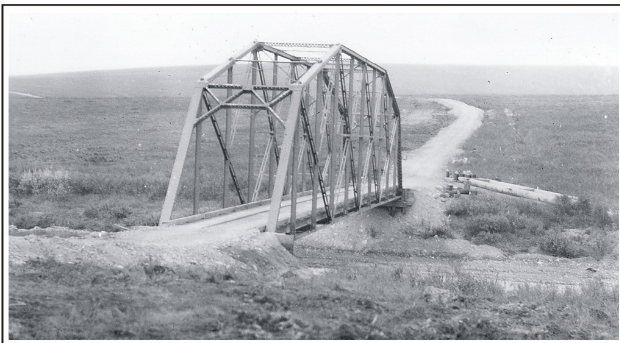
Figure 134. Camelback truss bridge at Kougarok River, September 30, 1941. U.S. Alaska Road Commission Collection, PCA 61-141-16, Alaska State Library.
