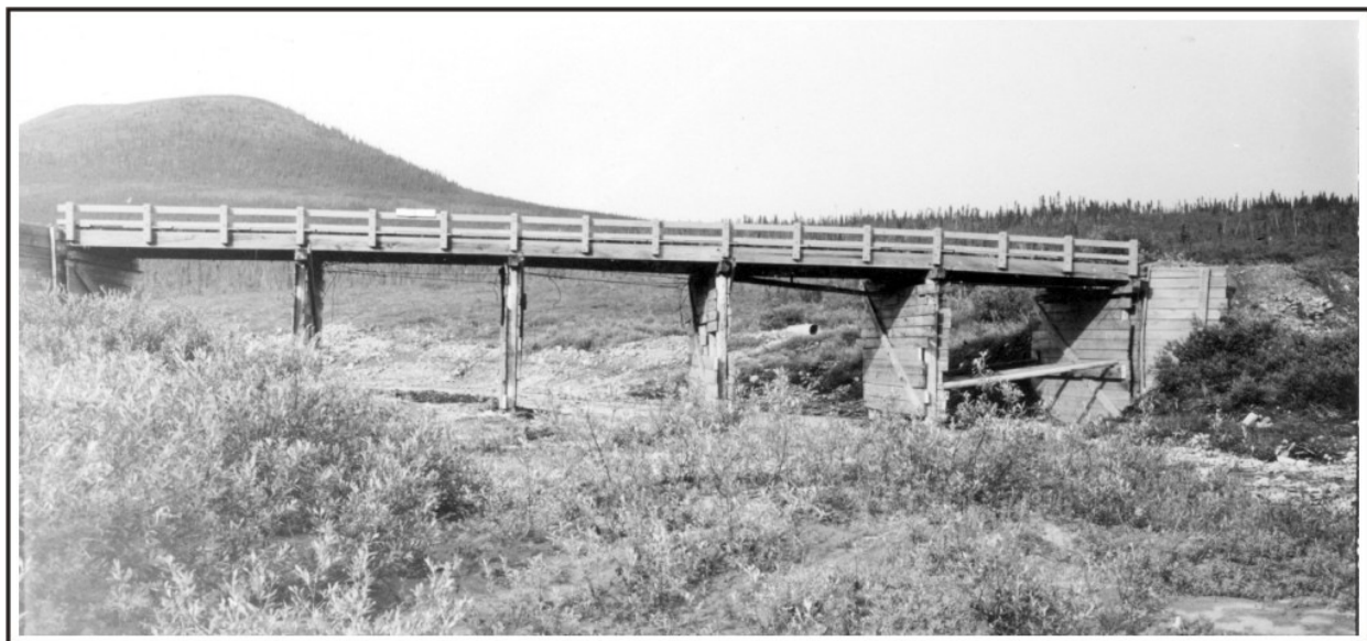
Figure 147. The timber pile trestle bridge built in 1949 at North Fork/12 Mile Creek on the Steese Highway. Photo taken in 1959 courtesy of ADOT&PF Bridge Design Section, Juneau.
