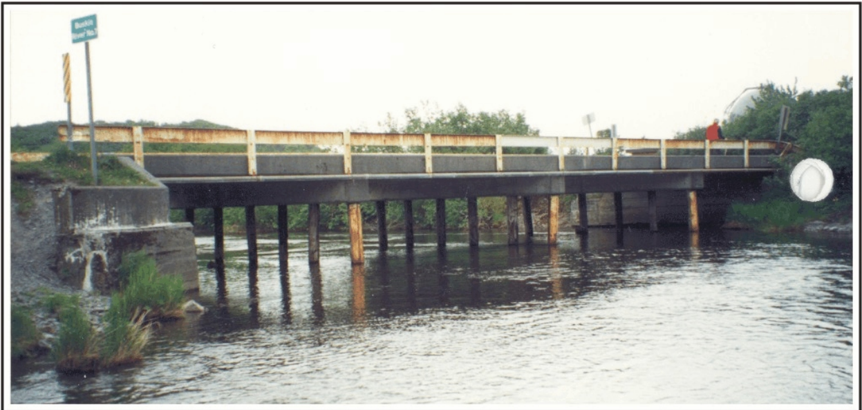
Figure 189. The U.S. Navy concrete slab continuous bridge at Bushkin River No. 7, July 6, 1996. Photo by Frank Muchmore and Jerry Mastin, ADOT&PF Bridge Section, Juneau.
