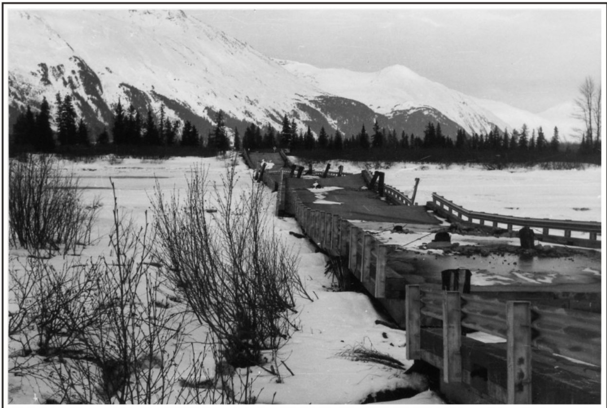
Figure 195. Earthquake damage to a concrete slab bridge, showing timber pilings punched through the concrete deck, April 1964. Photo courtesy of Bob Maurant, Juneau.
