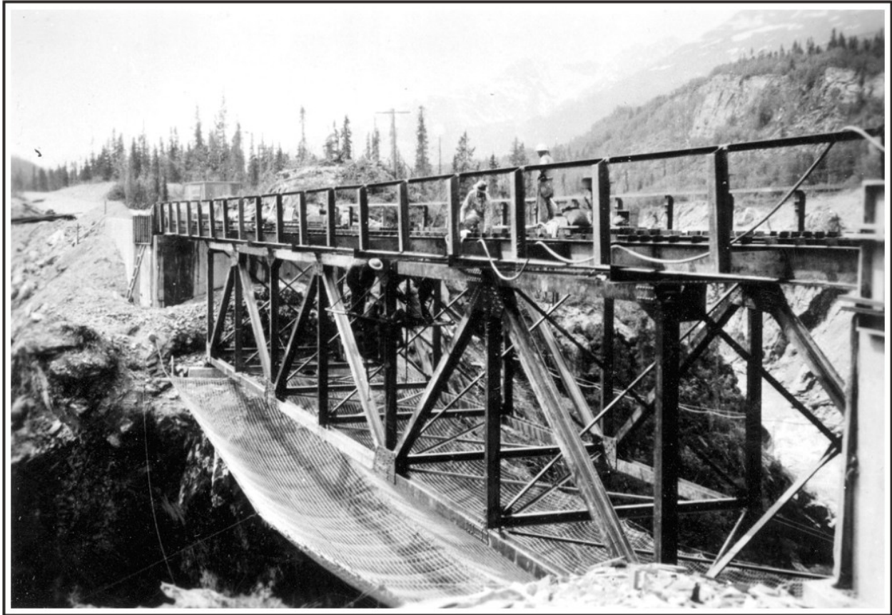
Figure 157. A crew constructing the steel deck truss bridge at the Tsaina River on the Richardson Highway, June 28, 1954. Photo courtesy of ADOT&PF Bridge Section, Juneau.
