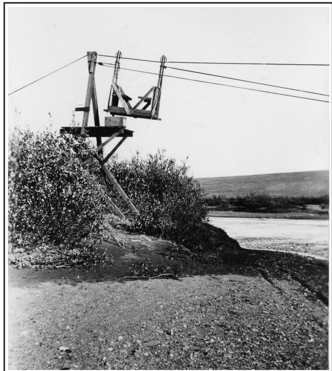
Figure 72. A standard cable tram installed by the ARC on river crossings. Photo courtesy of ADOT&PF Bridge Section, Juneau.
