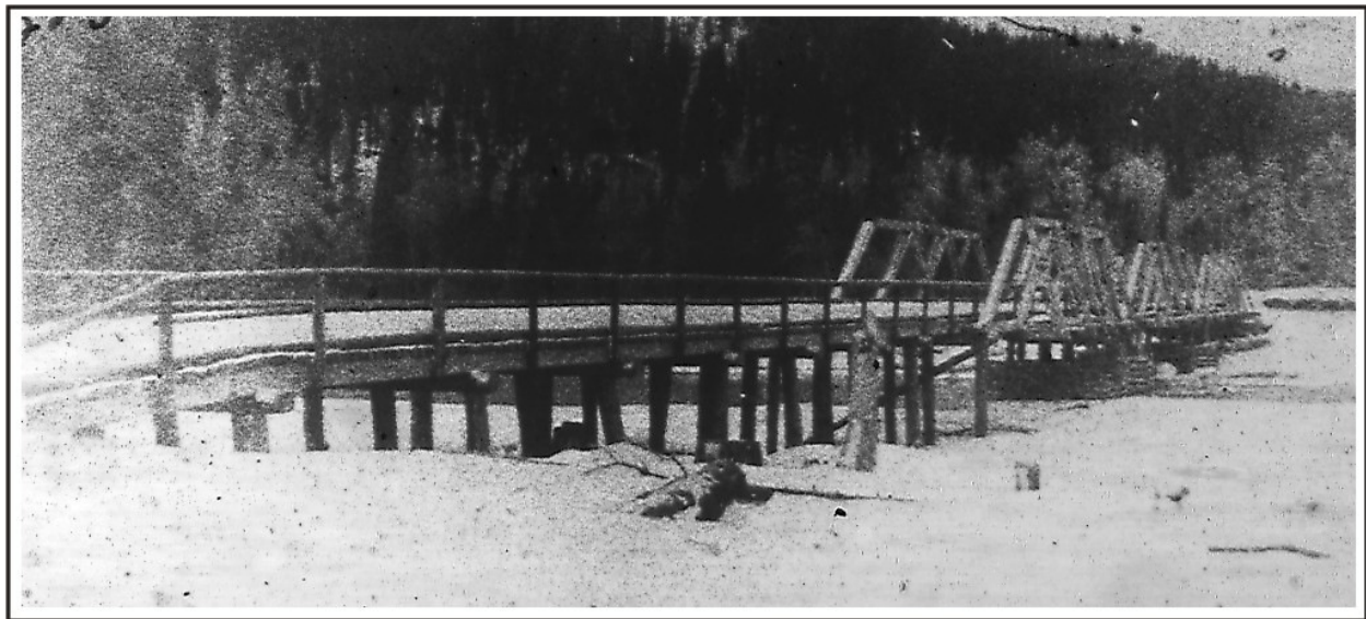
Figure 88. The Moose Pass-Takotna Bridge, a timber pony truss bridge, 1930s. U.S. Alaska Road Commission Collection, PCA 61-1-325, Alaska State Library.
