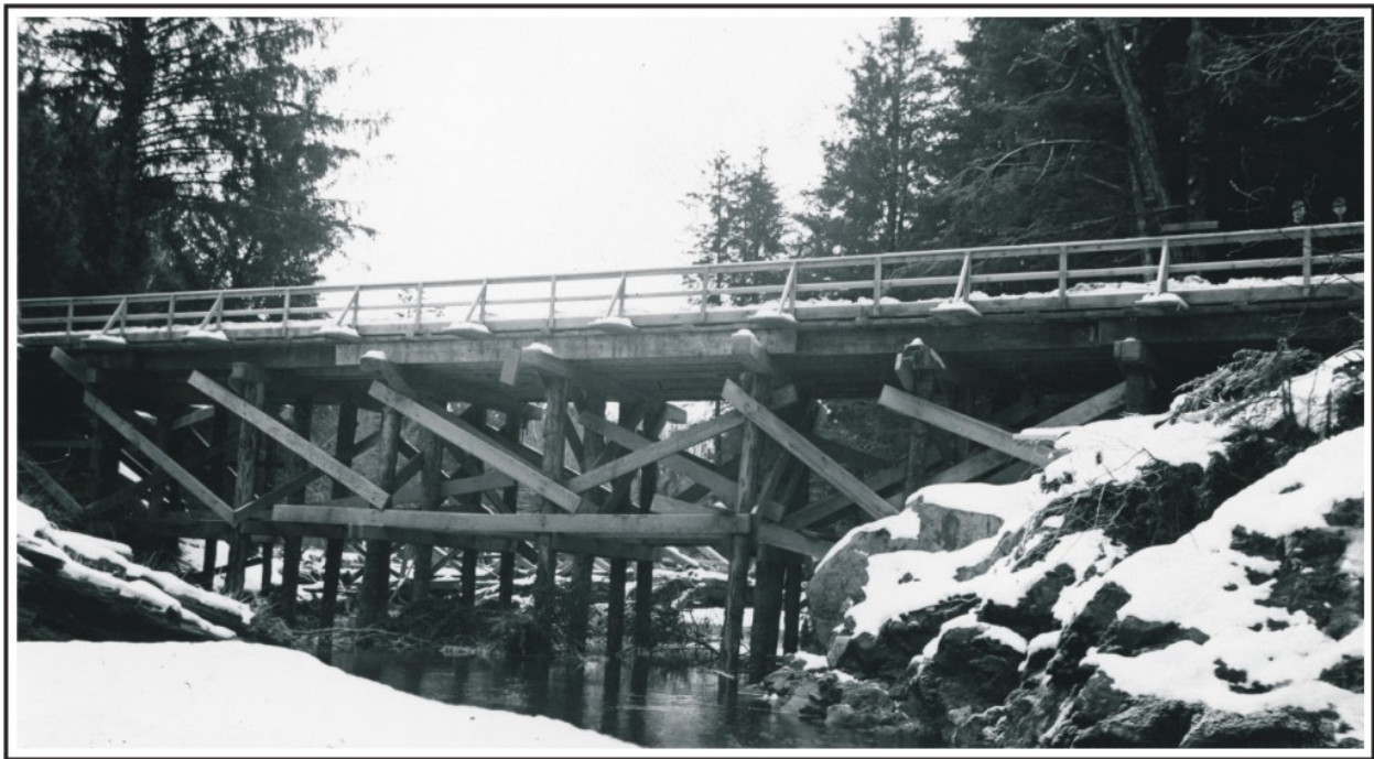
Figure 143. Temporary timber trestle bridge built by the U.S. Navy at Indian River near Sitka, Fall 1942. U.S. Alaska Road Commission Collection, PCA 61-76-18, Alaska State Library.
