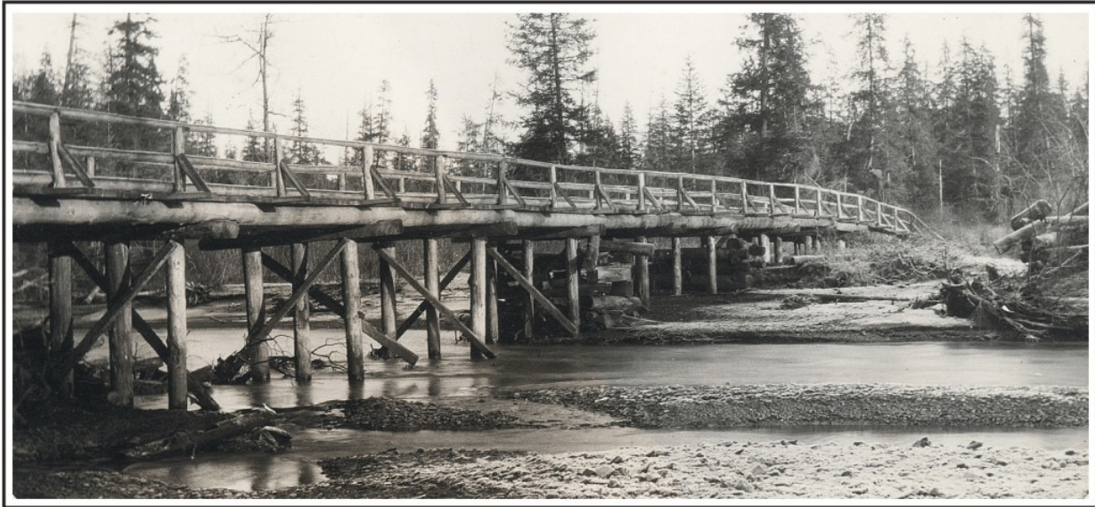
Figure 77. Bridge No. 5, a pile trestle bridge built by the BPR, at Mile 7 of the Seward-Kenai Lake Road, June 10, 1927. U.S. Alaska Road Commission Collection, PCA 61-66-16, Alaska State Library.
