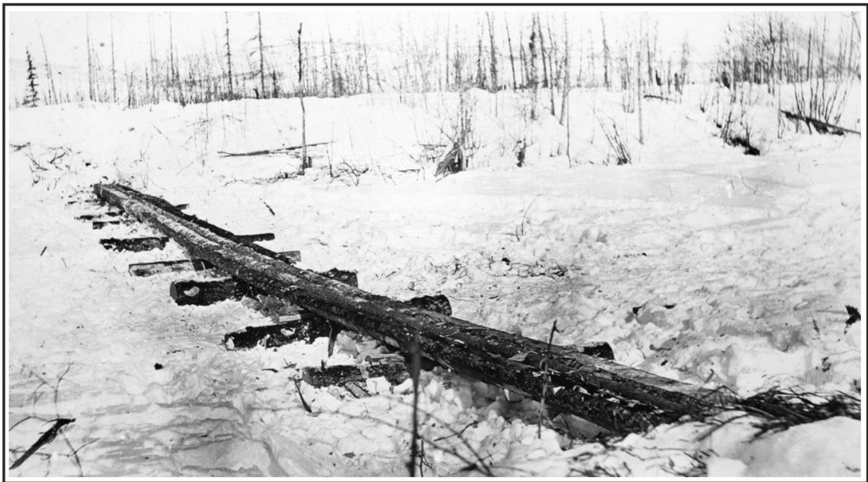
Figure 18. An example of a simple log foot bridge built in the interior in the early 1900s. Rita Cottnair Album, 1974-130-101, University of Alaska Fairbanks.
