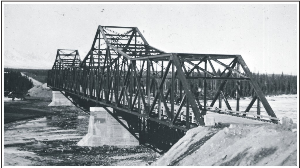
Figure 140. The cantilevered 3-span steel Warren truss bridge at the Tanana River on the Alaska Highway, 1944. U.S. Alaska Road Commission Collection, PCA 61-107-B69, Alaska State Library.
