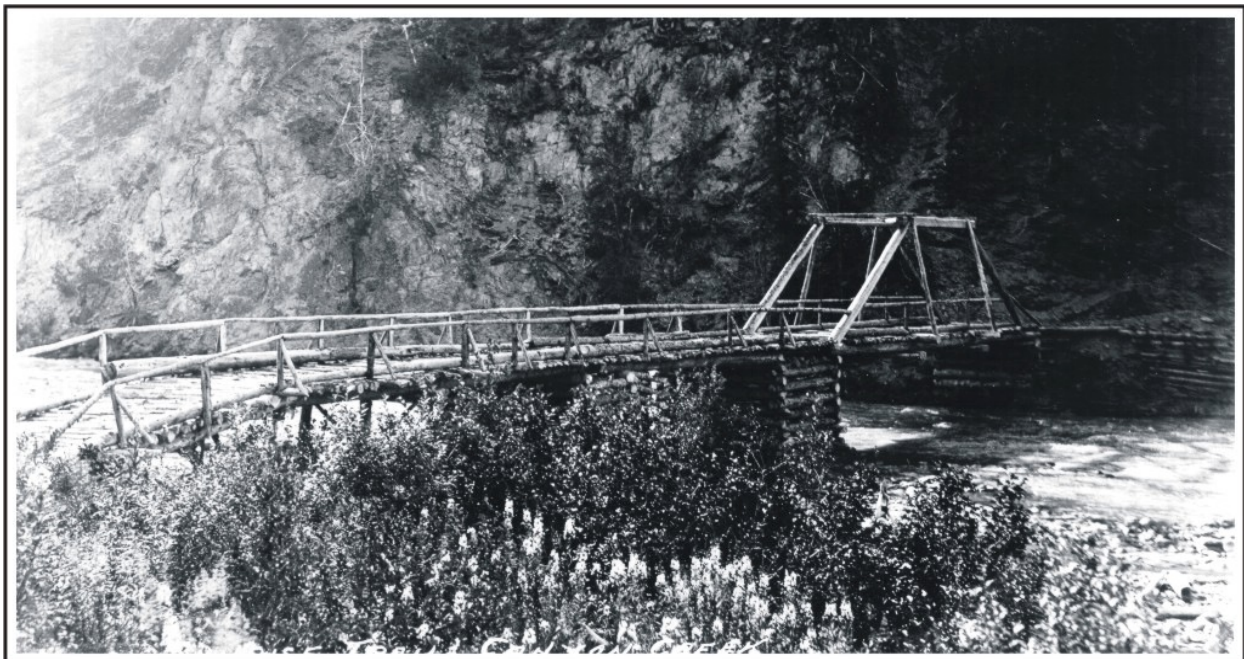
Figure 44. An example of a queen post truss bridge, one of the first bridges over Canyon Creek on the trail to Sunrise near Turnagain Arm, 1911. Photo by L.H. Peterson, Lot 8749, Library of Congress, Washington, D.C.
