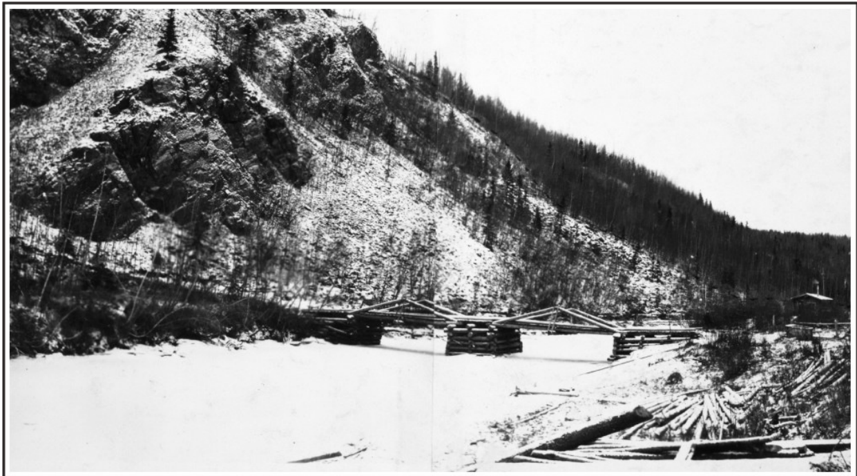
Figure 47. The two span king post truss bridge at Shaw Creek on the Valdez-Fairbanks Road, winter 1912. Rita Cottnair Collection, 1974-130-41, University of Alaska Fairbanks.
