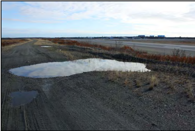
Photo 20: Thaw-settlement depression in road surface along E/W runway.
