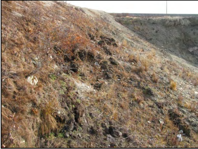
Photo 1: Approximate 2H:1V slope in mining cut east of Nome.
