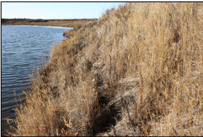
Photo 26: Tension cracks in vegetated slope above mining pit.
