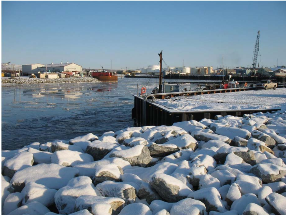
Photo 10 – Sheet pile and riprap shorelines within the Inner Harbor.
