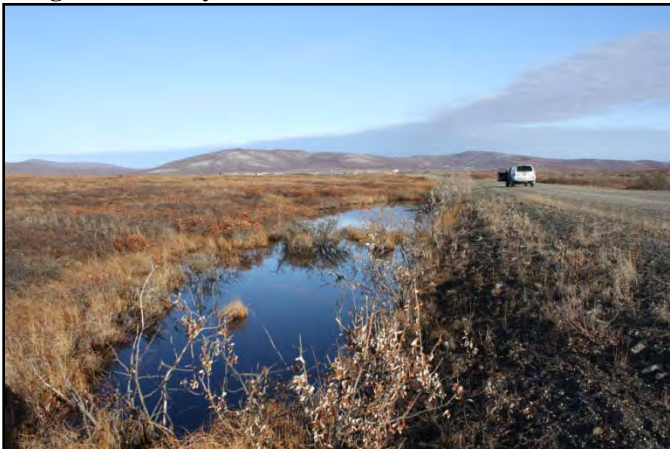
Photo 21: Thaw settlement at toe of road embankment along N/S runway.
