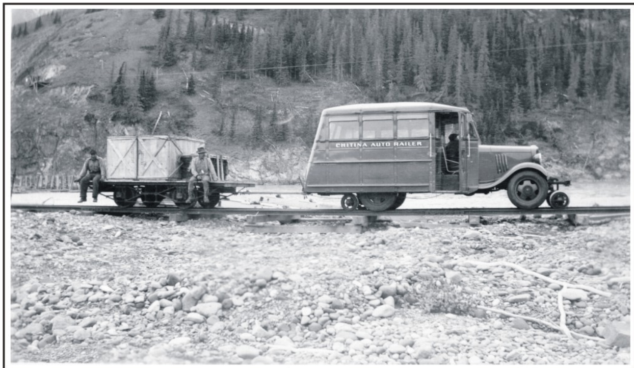
Figure 20. O.A. Nelson's "Chitina Auto Railer," 1940s. Nelson used this rig to carry passengers and freight between the Copper River (background) and McCarthy. Photo courtesy of Robert Coats, Anchorage.
