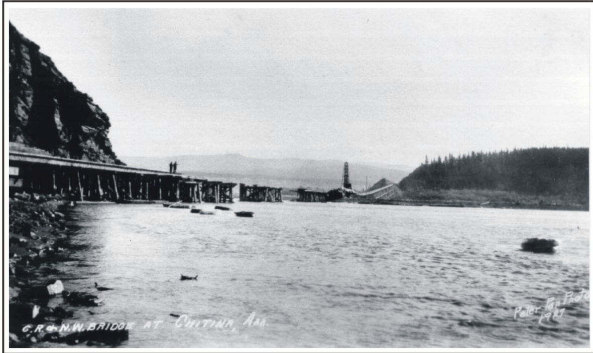
Figure 12. The trestle bridge over the Copper River east of Chitina, damaged during flooding in August 1927. Photo courtesy of Malcolm Storey, Vancouver, Washington.
