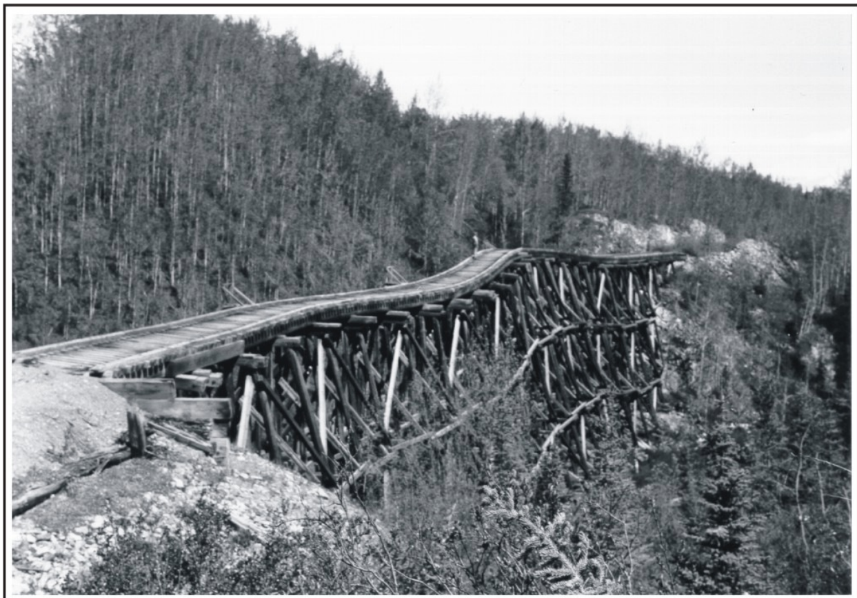
Figure 27. The sagging trestle bridge east of Long Lake, June 1962. The view is looking east. Photo by Lynn Yehle, U.S. Geological Survey, Denver.
