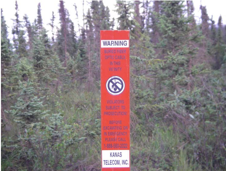
Figure 18. Kanas Telecom fiberoptic line marker (NLUR photo).
