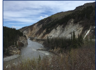
The highway is constrained by areas of slope instability and erosion by the river in the Nenana Canyon (MP 239-241)
