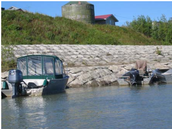
Figure 7 – Cement bag revetment to protect main bank at Village of Noatak.
