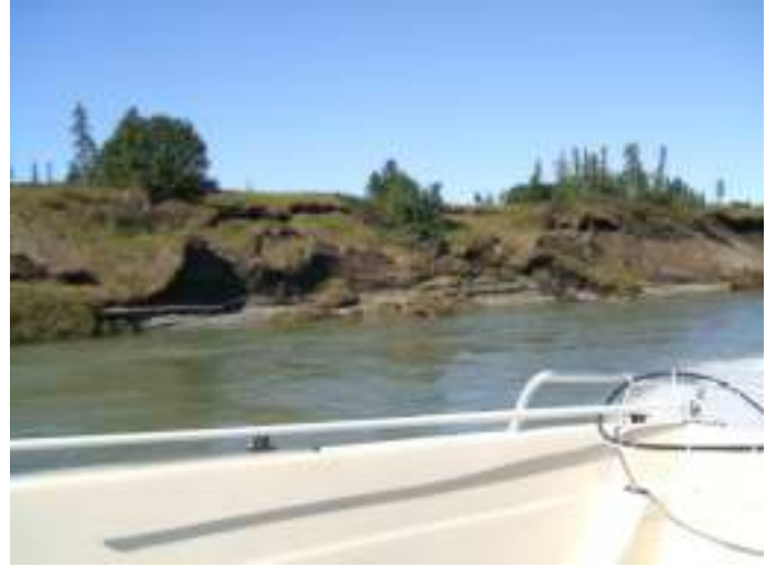
File Name:West Mainland bank erosion 1.jpg Capture Date:2006/08/16 15:58:48
