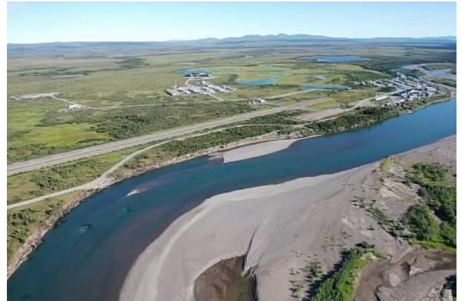
Noatak Airport, located on the shore of the Noatak River, is threatened by river erosion. - Photo by Jeff Luther
