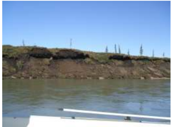
File Name:West Mainland bank erosion 3.jpg Capture Date:2006/08/16 16:03:25
