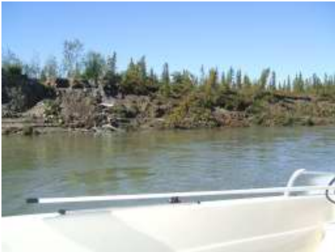
File Name:West Mainland bank erosion 2.jpg Capture Date:2006/08/16 15:59:01
