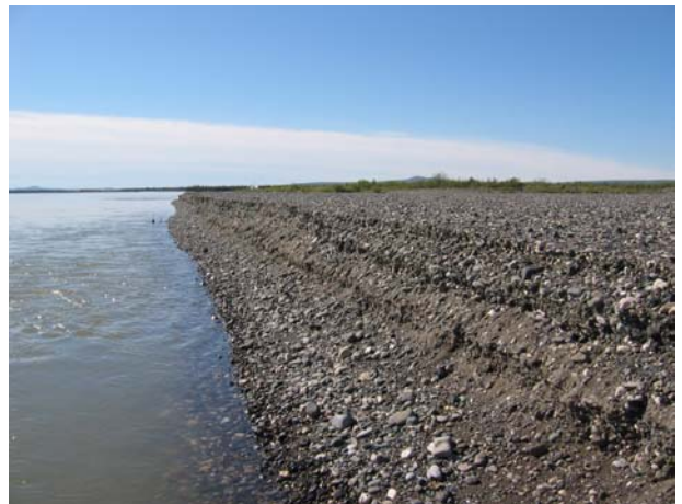
Figure 4 – At mid-section of island, looking downstream. Gravel bank is 2-3 feet above water surface elevation.
