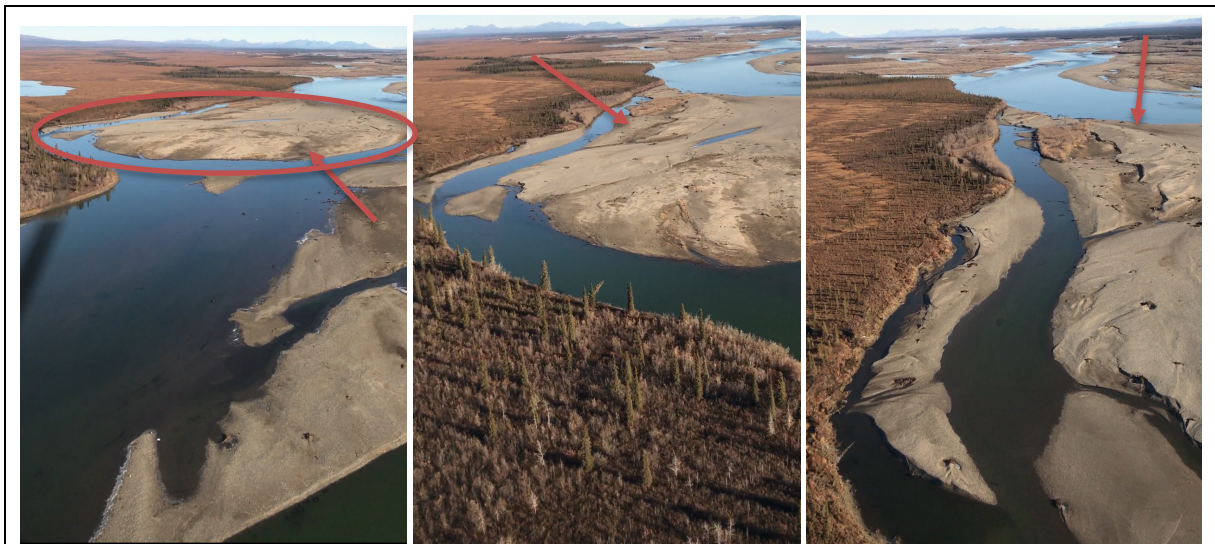
2017 Overview of Noatak River at Proposed River Material Source (South) (Red Arrows)
