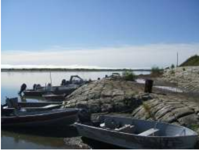
File Name:noatak erosion control project 2.jpg Capture Date:2006/08/16 15:55:29
