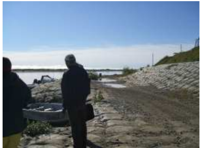
File Name:noatak erosion control project 1.jpg Capture Date:2006/08/16 15:55:03
