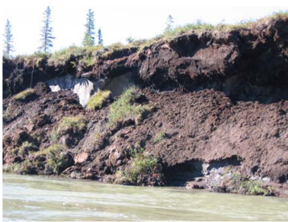
Figure 1 – Left bank of Noatak River downstream from village, with visible ice lenses and active erosion.
