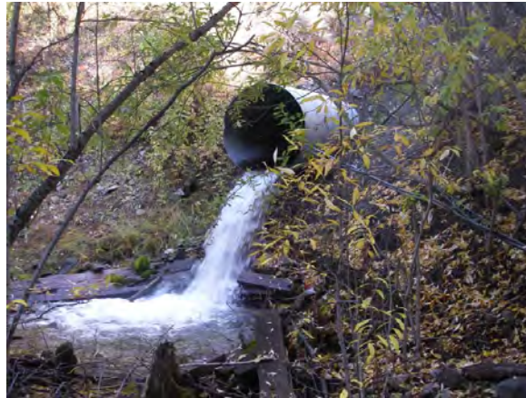
Figure 6-31. Swift Creek Crossing (MC 2), Downstream Looking Upstream
