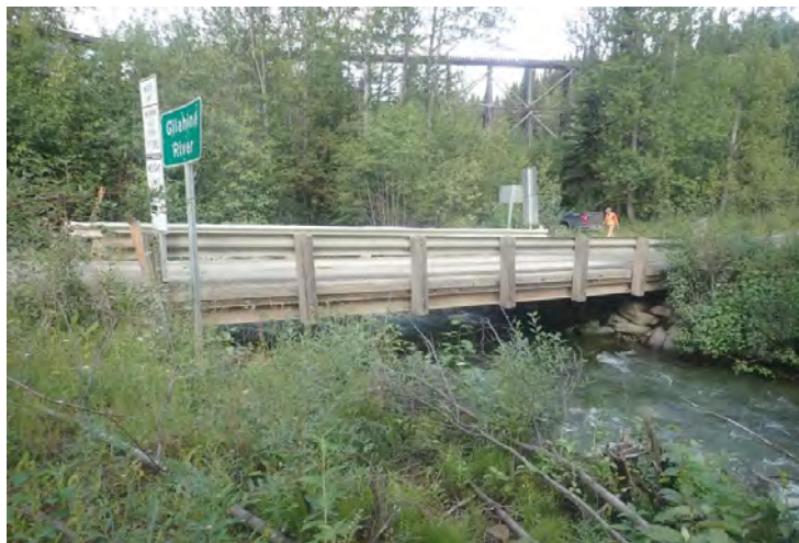
Figure 6-17. Gilahina River Bridge (BR 1194), Downstream Looking Upstream
