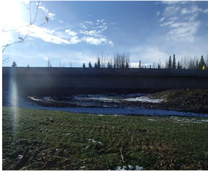
Figure 6-9. Chokosna River Bridge (BR 1193), Upstream Looking Downstream
