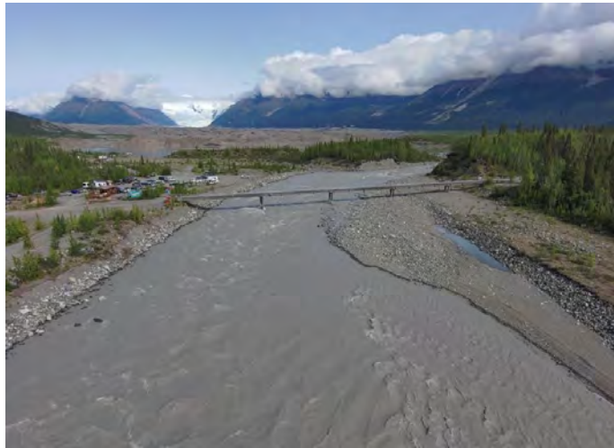
Figure 6-35. Kennicott River Bridge (BR 6004), Downstream Looking Upstream
