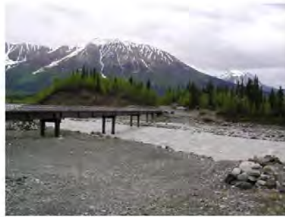
Kennicott River bridge crossing
