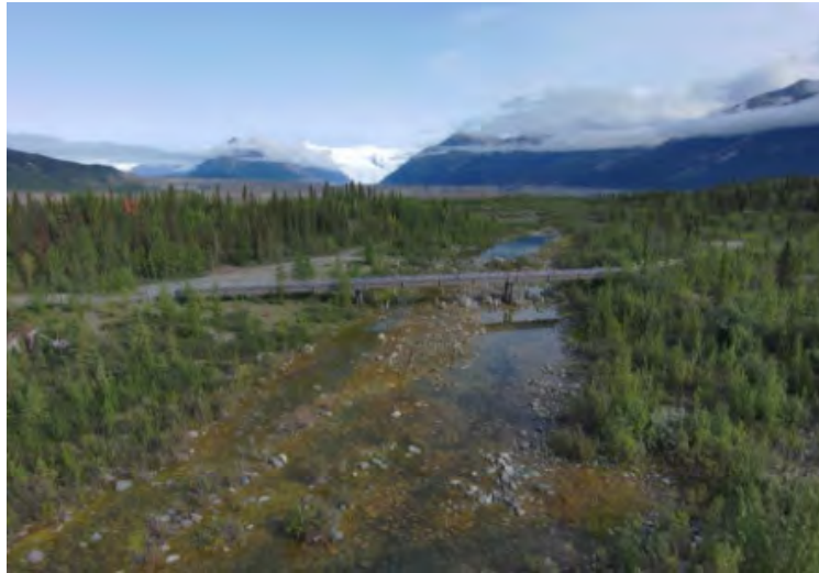
Figure 6-36. Kennicott River Bridge (BR 6005), Downstream Looking Upstream
