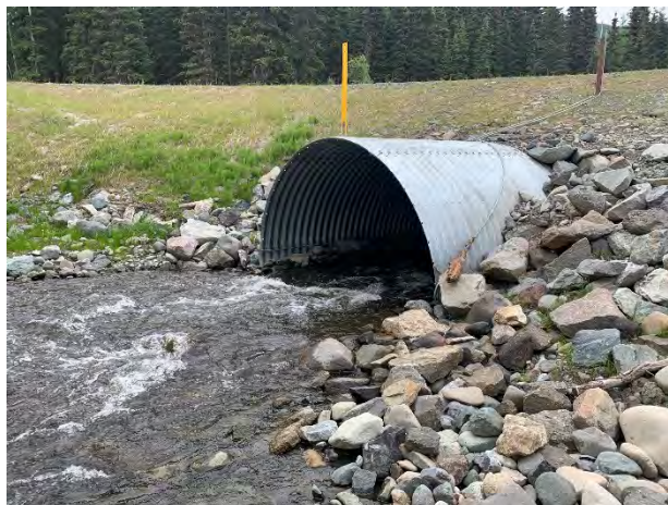
Figure 6-22. Crystal Creek (MC 9), Looking Upstream (post-improvement project)
