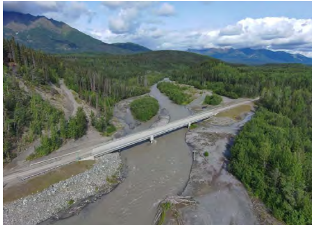
Figure 6-23. Lakina River Bridge (BR 1195), Upstream Looking Downstream
