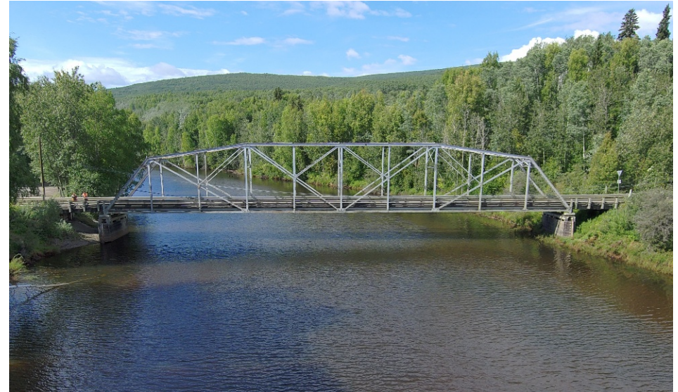
Picture looking west/downstream
