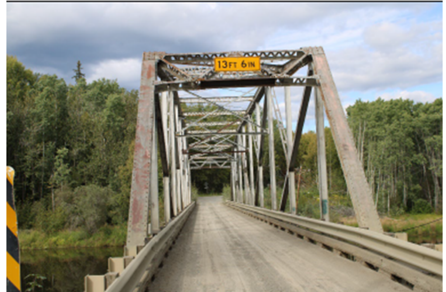
South portal of Hot Springs Slough Bridge, view north
