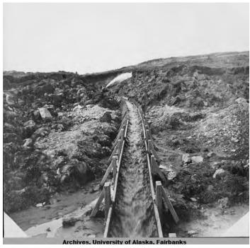
Figure 5. Water flume ditch for mining operations near Deering (UAF 2013a, Assec# UAF-1999-132-CO).
