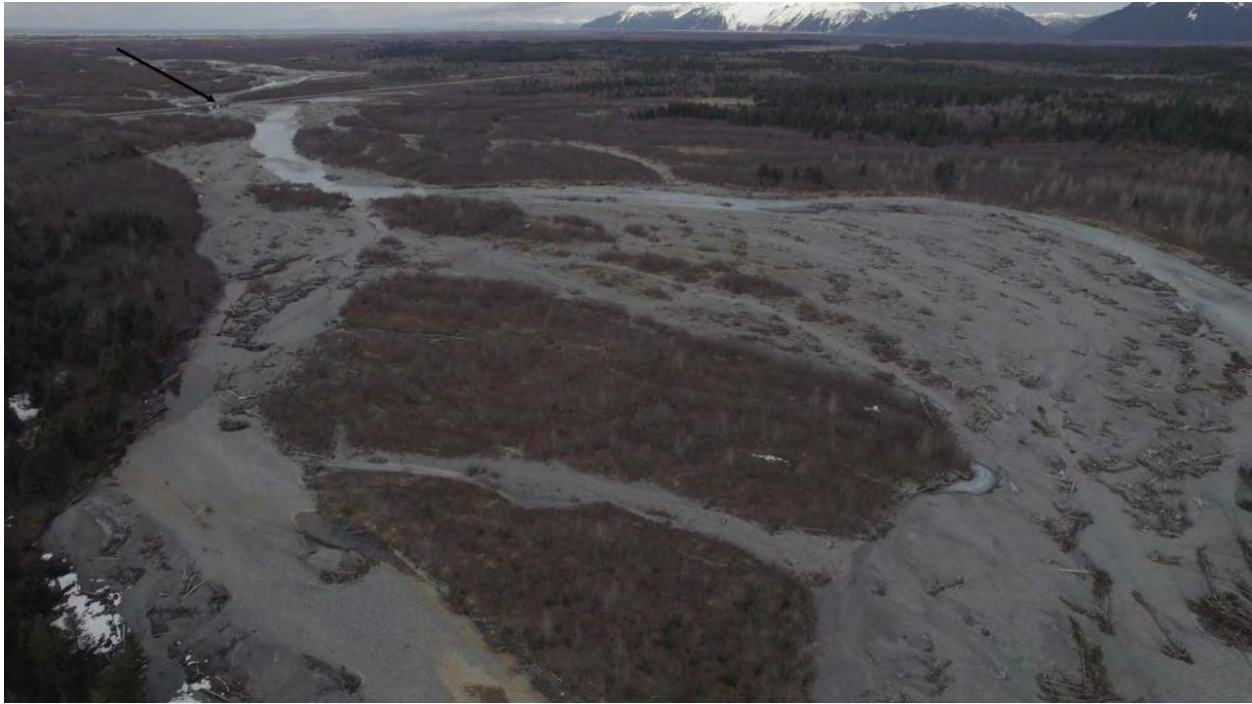
Image 2: Drone imagery showing the undersized bridge in the distance.
