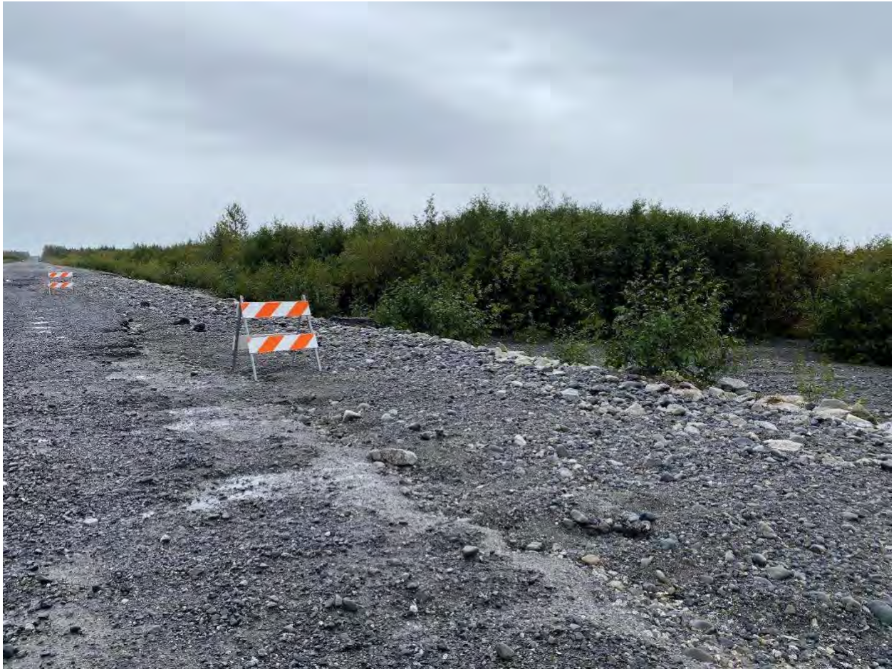
Image 5: "French mattress", Bridge approach from the west side. Loses road topping during high water events as river overtops the road.
