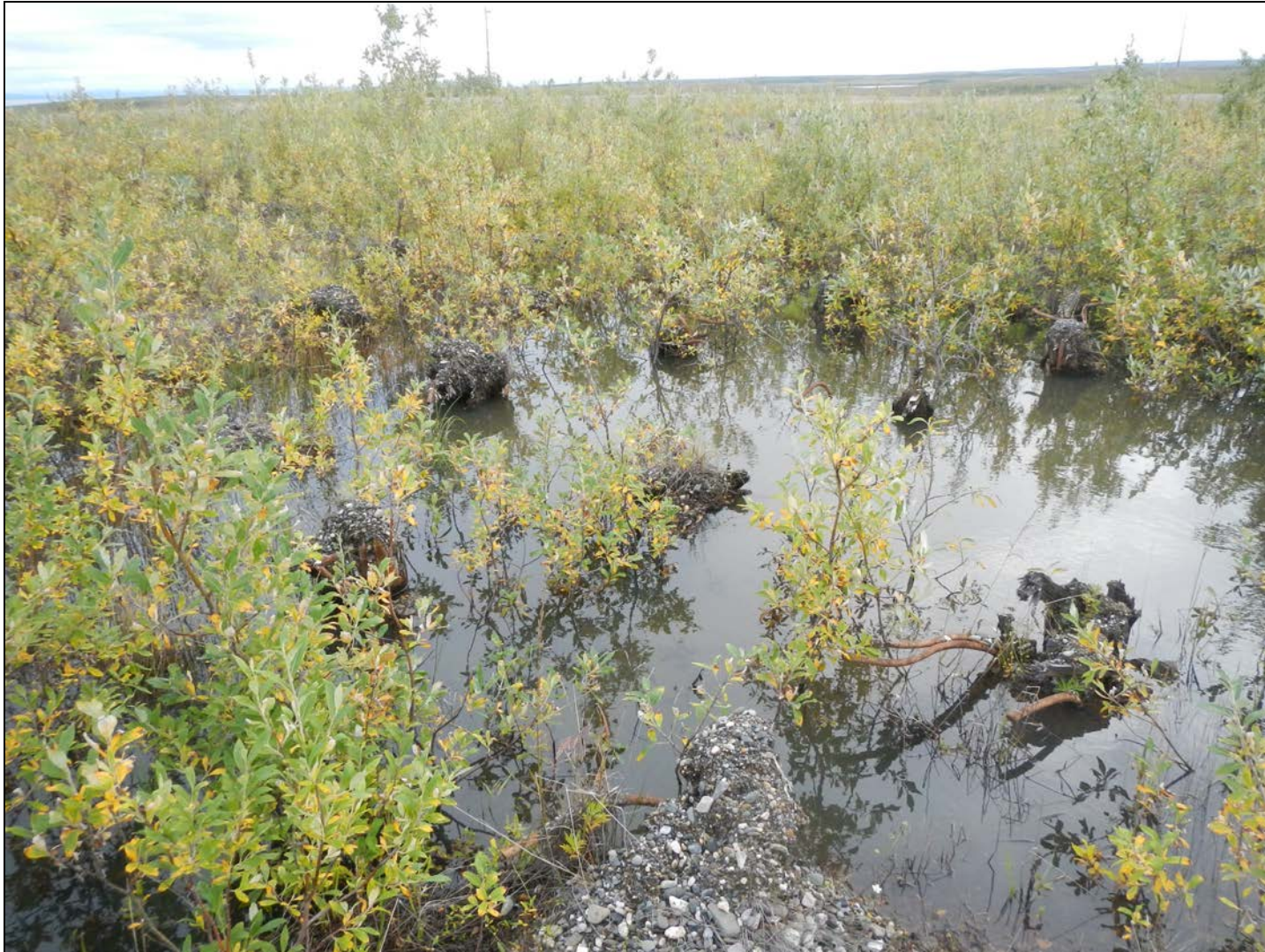
Figure 9. Foundation remains southeast of the Radome Tower Building (NLUR photo). These are included in Figure 8 and demonstrate the extent of the demolition carried out by the USAF on the buildings at the Kotzebue LRRS.
