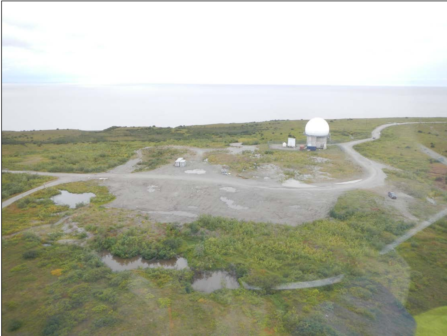
Figure 8. Aerial view looking west at the Radome Tower Building (KTZ-00190) within the high probability area of the Alternative A- Upgrade Route (NLUR photo). The LRRS Gravel Pad (KTZ-00232) is visible in the center. A portion of the LRRS Road System / Air Force Road (KTZ-00231) passes from left to right across the Gravel Pad. The road to the Kotzebue wind farm is visible as the lower road on the left of the photograph.
