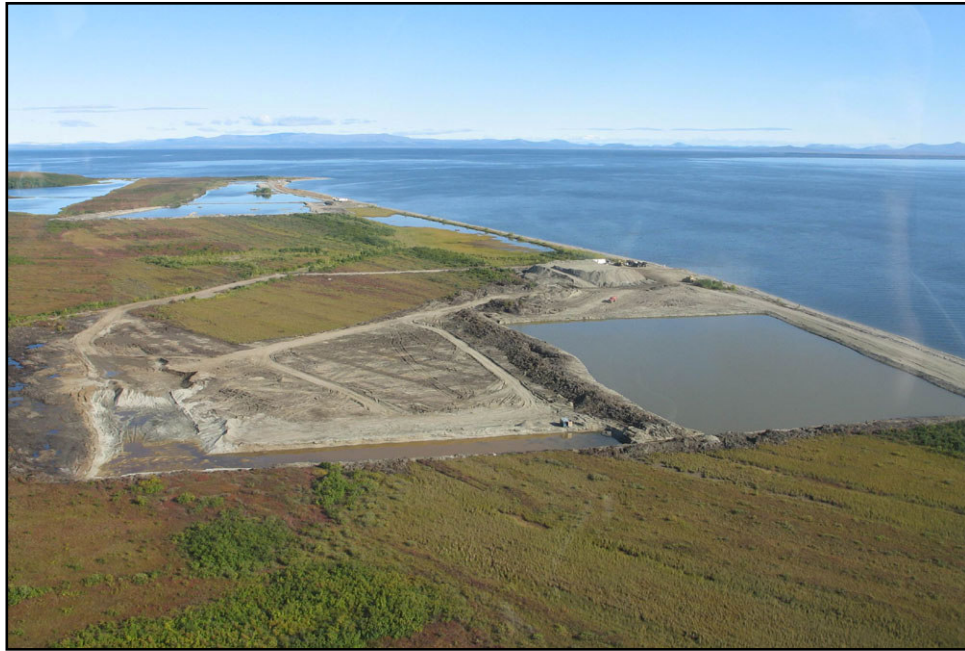
FIGURE 11: ACTIVE BORROW PITS, NIMIUK POINT (K.I.C/QAP Pt in foreground, and Drake Pit in background; 30 August 2006)
