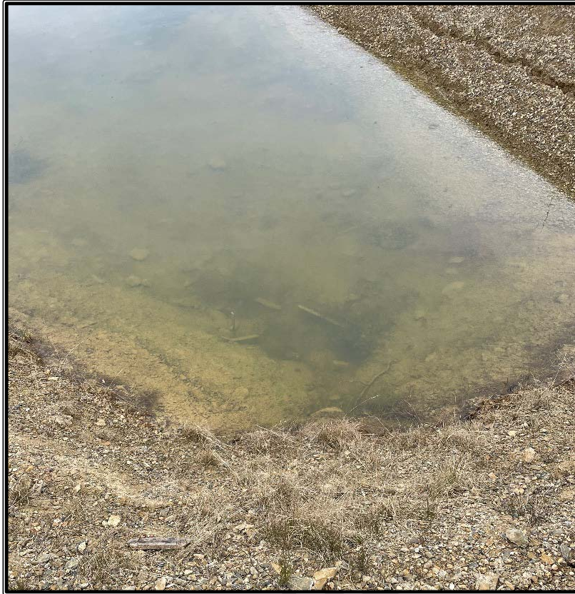
Figure 7: Infield Access Road Area – Culvert Inlet
