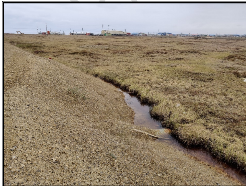
Figure 8: Infield Access Road - Culvert Outlet
