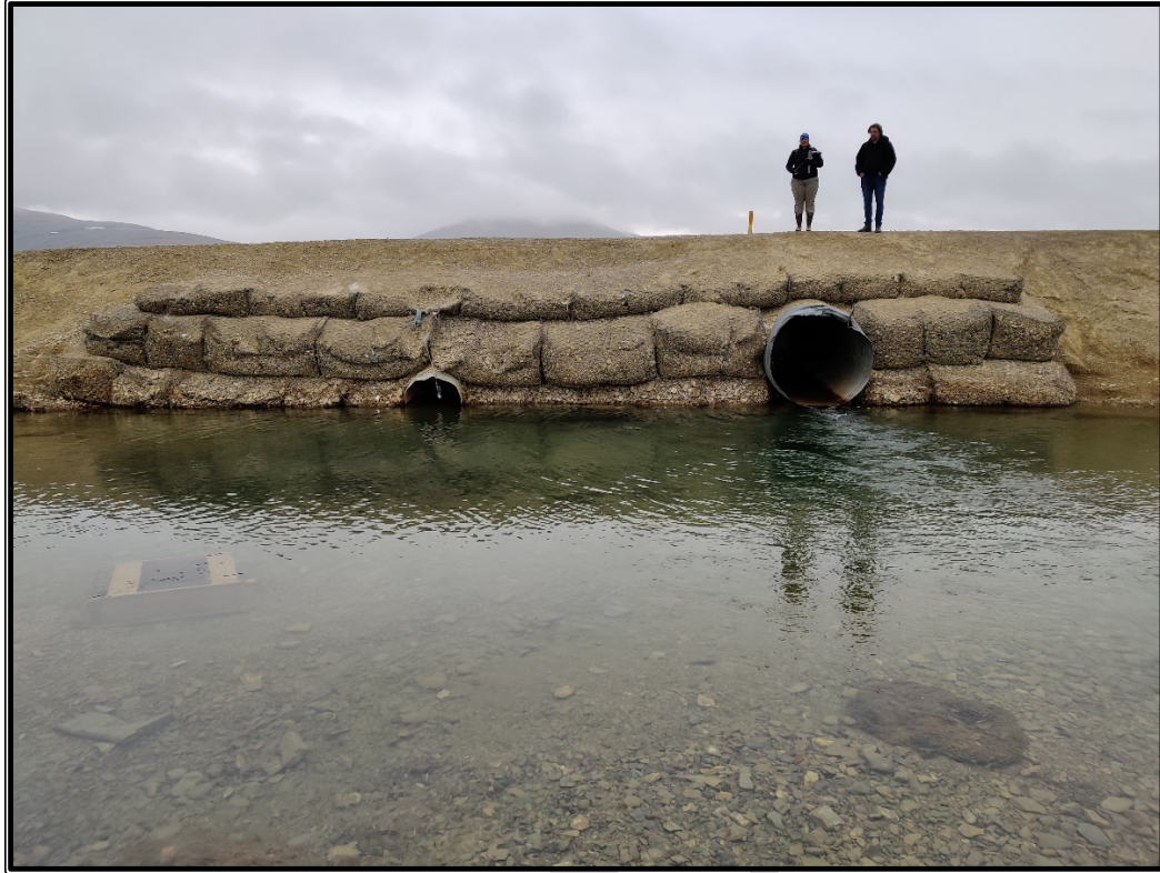
Figure 10: Shelman Creek Crossing – Clarence Road
