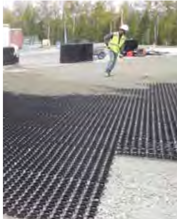
Grass Paver Fire Lane Installation
