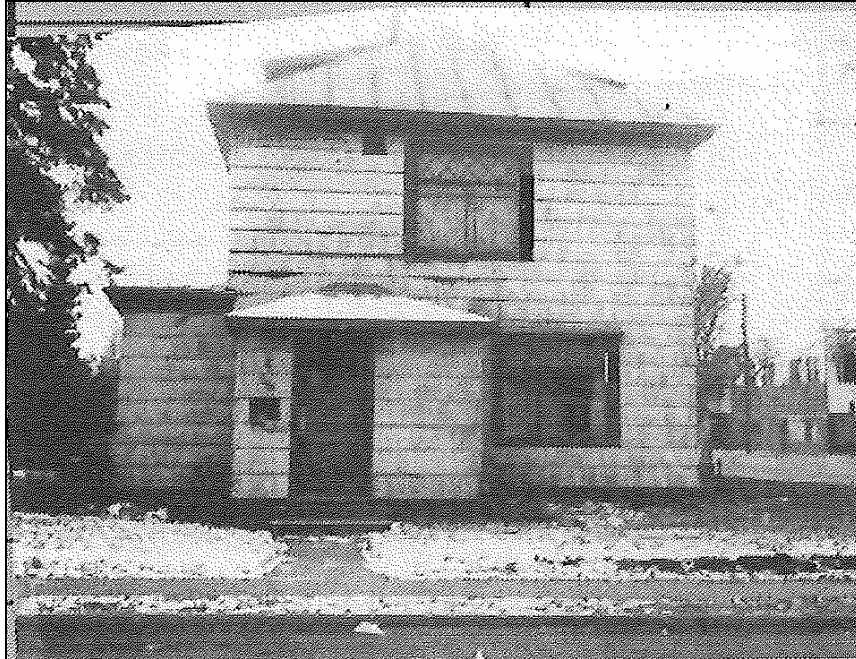
Figure 33: North elevation, decorative window detail, 1968. Assessors' photo.
