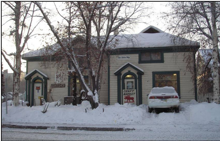
Figure 25. North elevation along 5 th Avenue, without foliage, Jan. 2008 (NLUR Photo).
