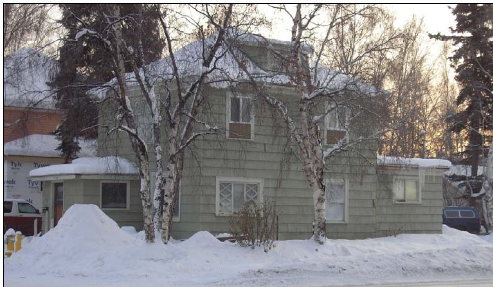
Figure 35: West elevation, Jan 2008 (NLUR Photo).
