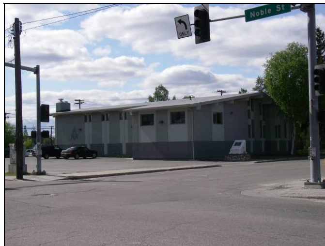
Figure 63: Masonic Temple east elevation (NLUR Photo).
