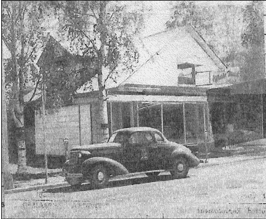
Figure 22. Undated assessor's photo showing west and north elevations.
