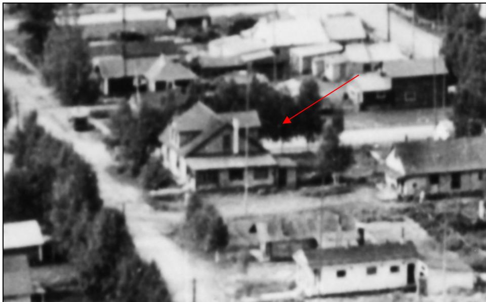
Figure 21: East and south elevations of 413 Noble, ca 1930s, prior to commercial conversion.
