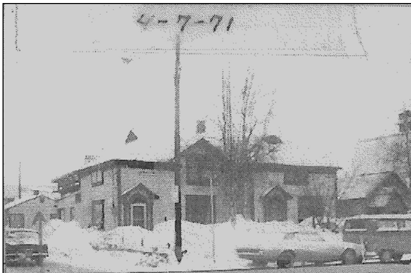
Figure 29: Right, FNSB Assessors' photo, north elevation, 1971
