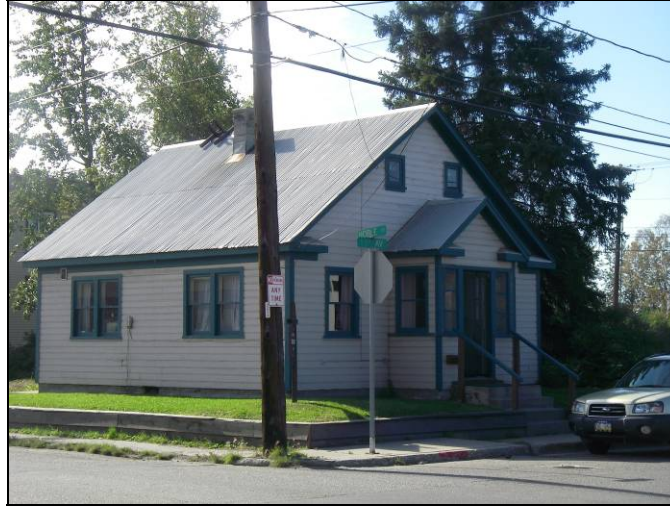
Figure 44: West and north elevations (NLUR Photo).
