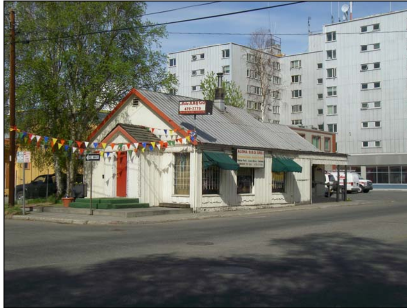
Figure 15: South and east elevations (NLUR Photo).
