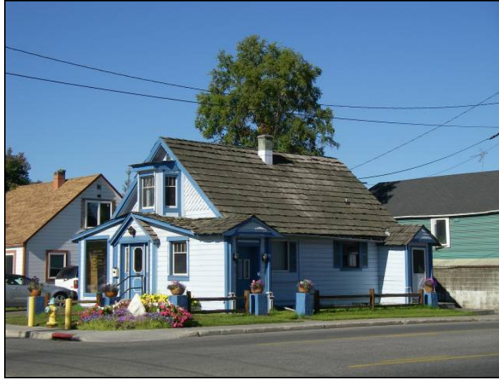
Figure 40: South and east elevations (NLUR Photo).
