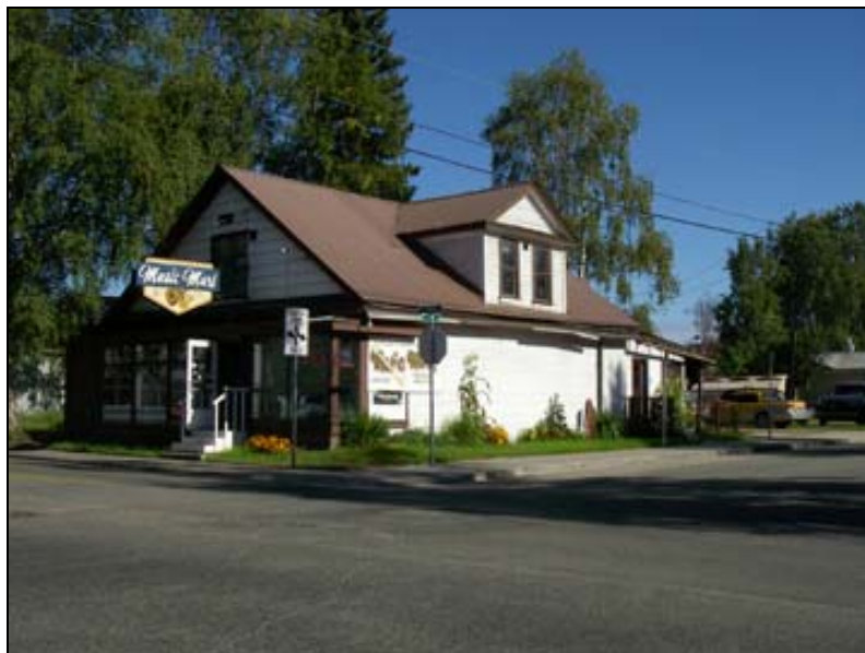
Figure 20. Music Mart, south and west elevations (NLUR Photo).
