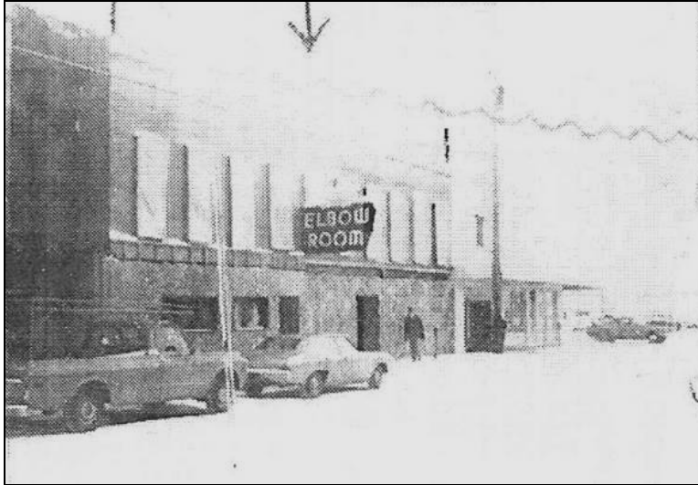
Figure 55. Elbow Room south elevation, December 1971, FNSB.
