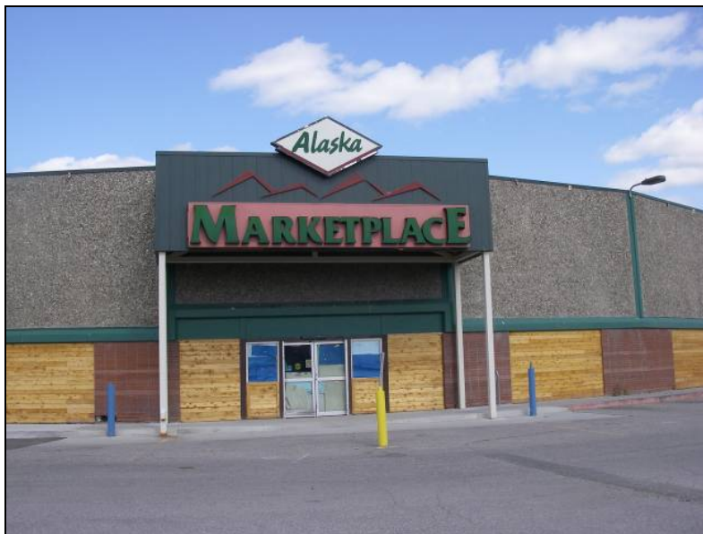
Figure 67: Main entrance, south elevation (NLUR Photo).
