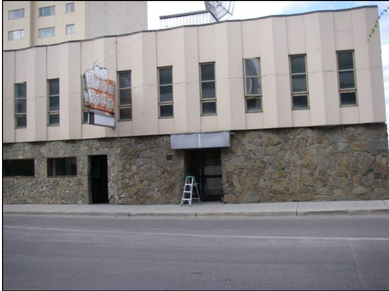
Figure 52. Elbow Room south elevation (NLUR Photo).
