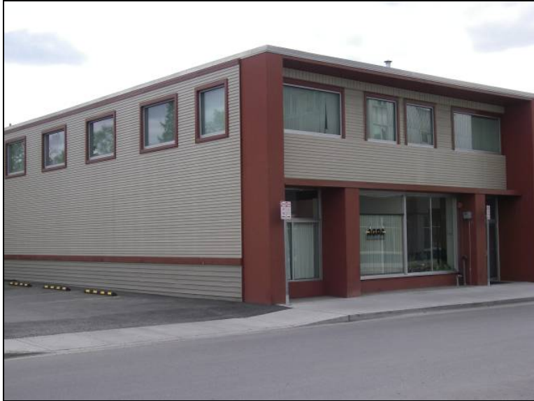
Figure 60: Port Authority north and east elevations (NLUR Photo).
