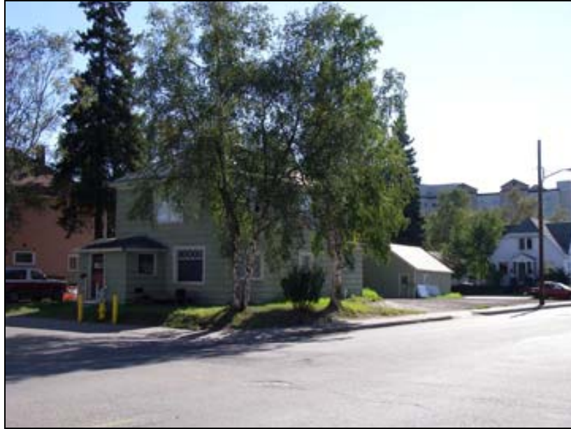
Figure 30: Left photo, north and west elevations (NLUR Photo).
