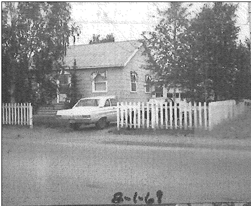
Figure 46: Assessors' photo, west elevation, 1968.
