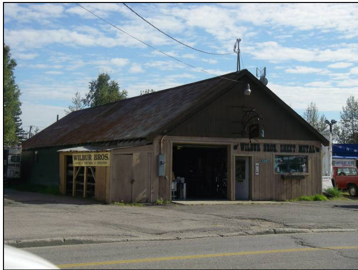
Figure 50: West and north elevations (NLUR Photo).
