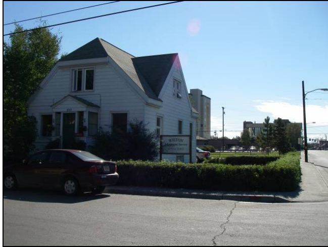
Figure 43. North and west elevations. Setting looking south (NLUR Photo).
