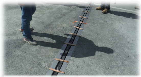
The new WIM site on the Klondike Highway
