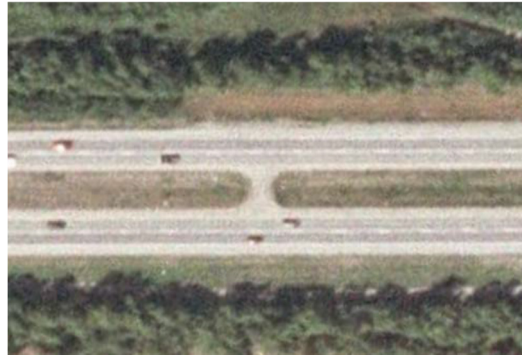
Freeway Crossover Example
