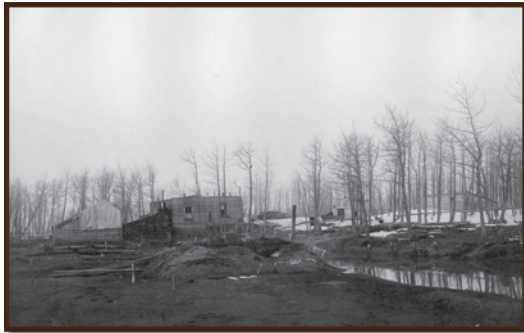
Buildings at Pilgrim Hot Springs, Alaska.
