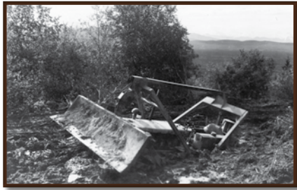
Road construction equipment in deep mud.
