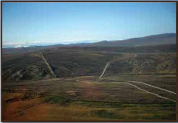
Dalton Highway and Trans-Alaska Pipeline
