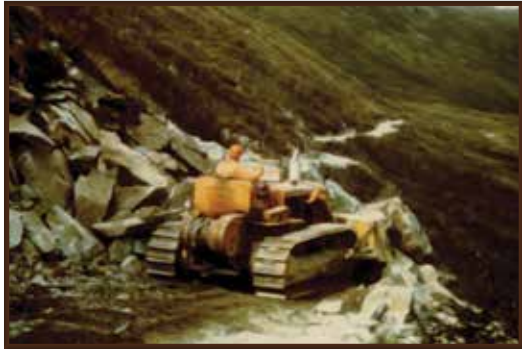
Clearing a rock-slide on Williamsport-Pile Bay Road with a bulldozer. Carl and Lyle Williams
