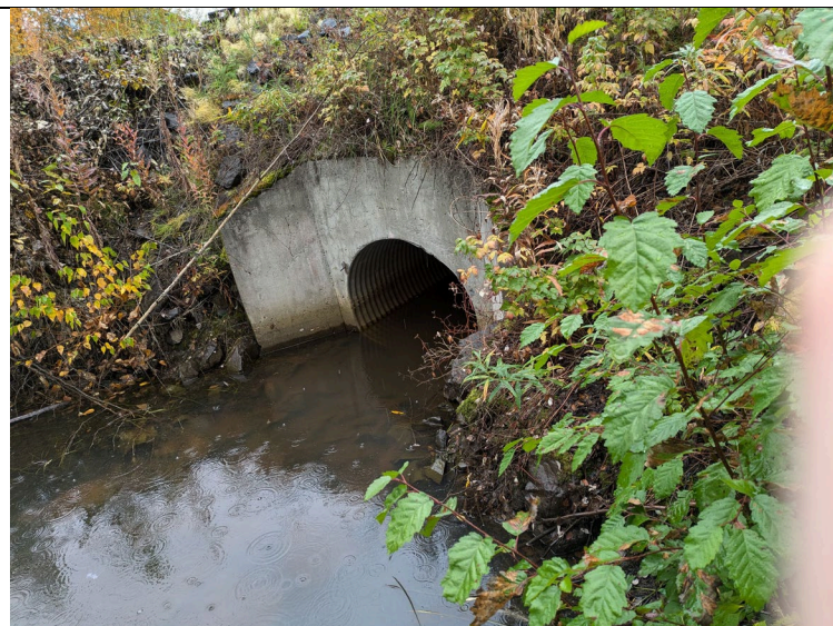
Description: Outfall 4B
