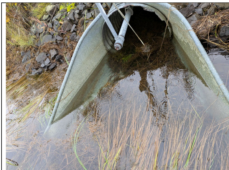
Description: Outfall 7D
