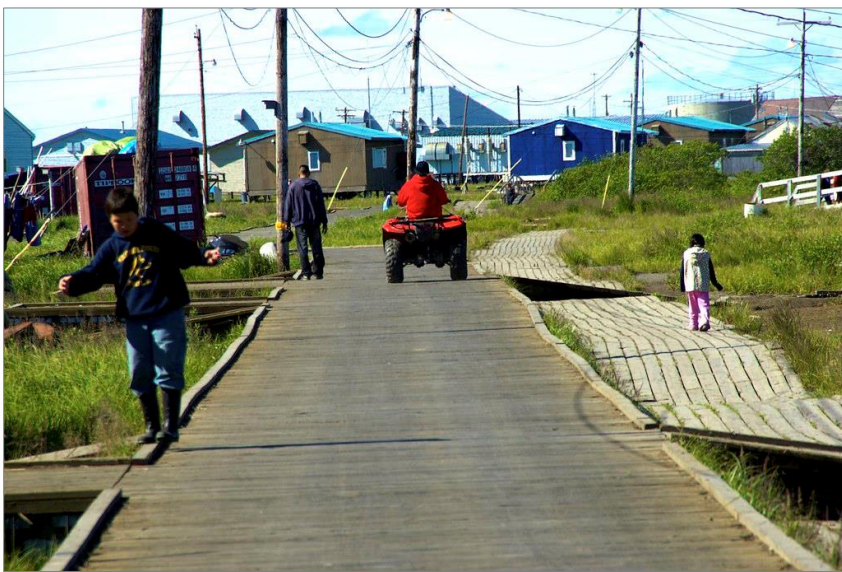
Figure 2. Board road in Kotlik, Alaska.
