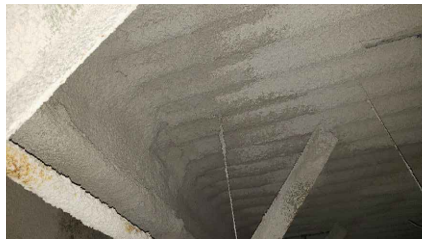
LOCATION 4: ACM FIREPROOFING ON PANDECKING IN GOOD CONDITION.
