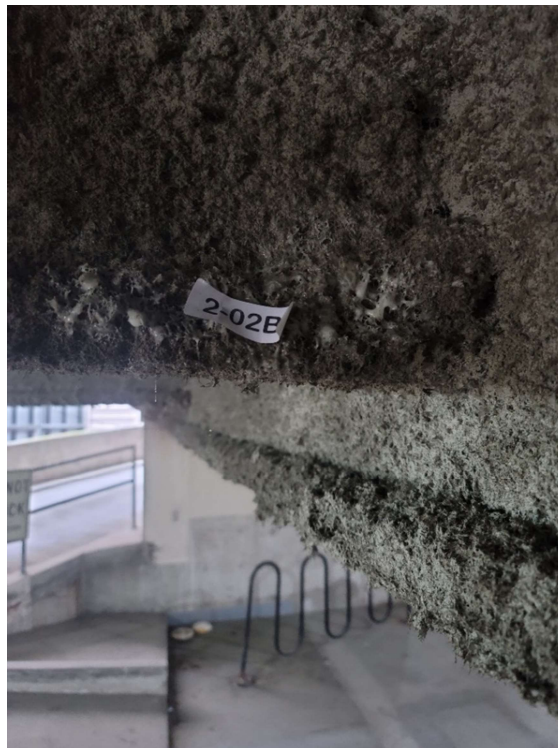
Photo 2: Dark gray fireproofing – standard spray pattern
