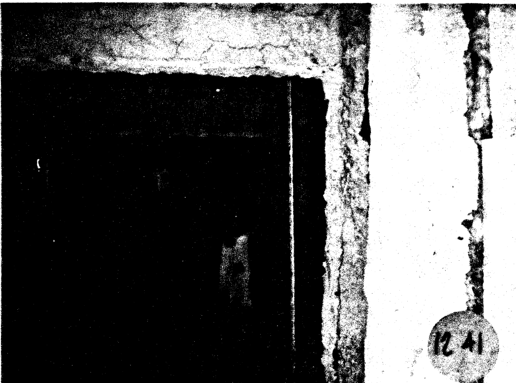
2. [12-41] Spray-on Fireproofing Below Ramp in Gallery 116
