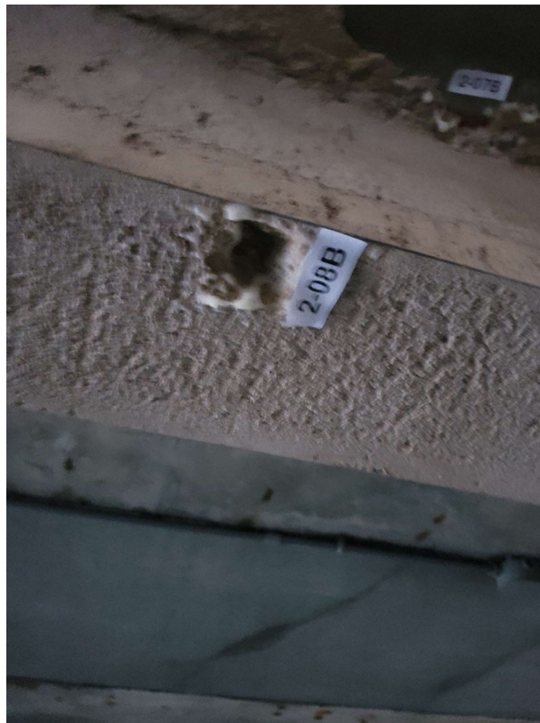
Photo 6: Tan fireproofing coating – sandy – smoothed
